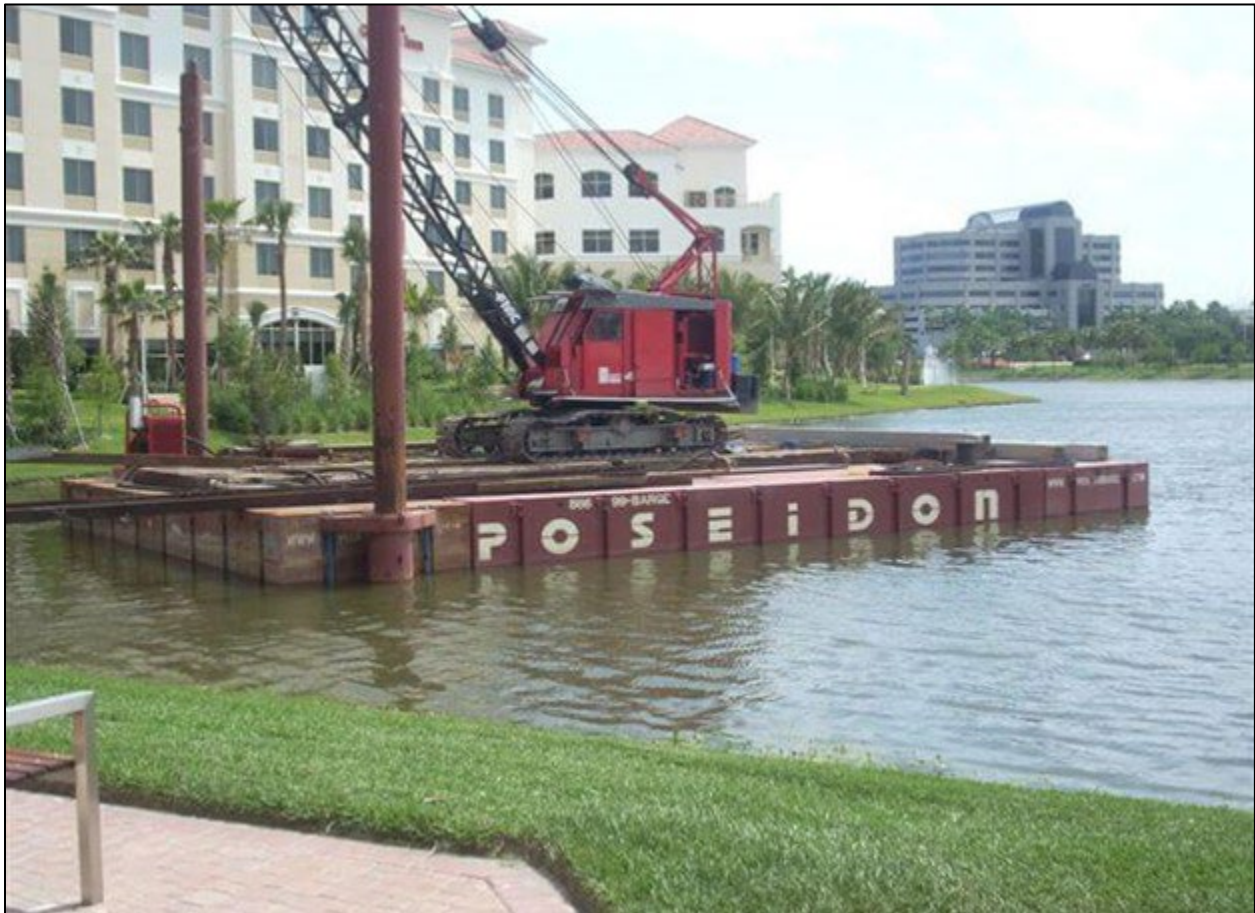
Figure 2-18. Photograph of a Sectional Barge with Mounted Crane
