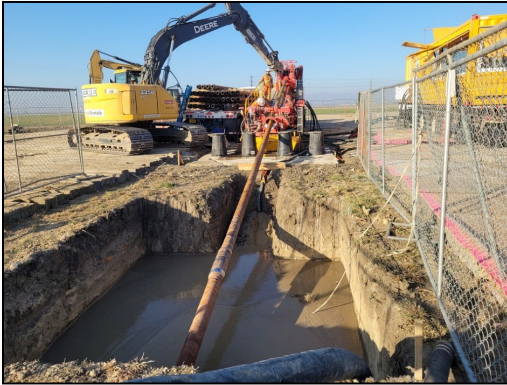
Figure 2-7. Photograph of an Example Drilling Rig and Bore Pit from a Previous Project
