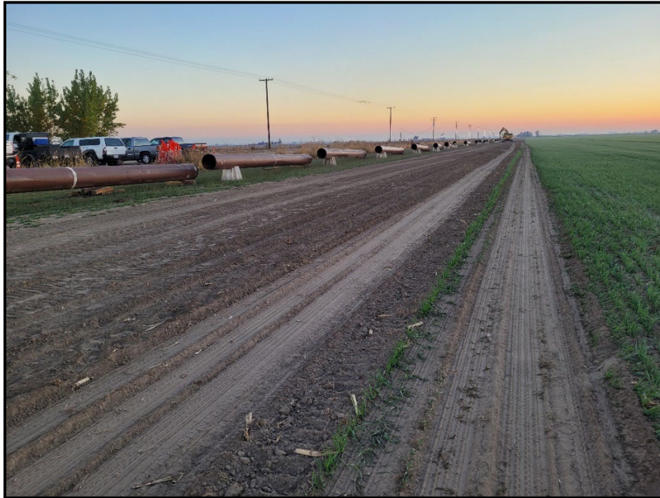
Figure 2-4. Photograph of Example Pipe Staging Area 4
