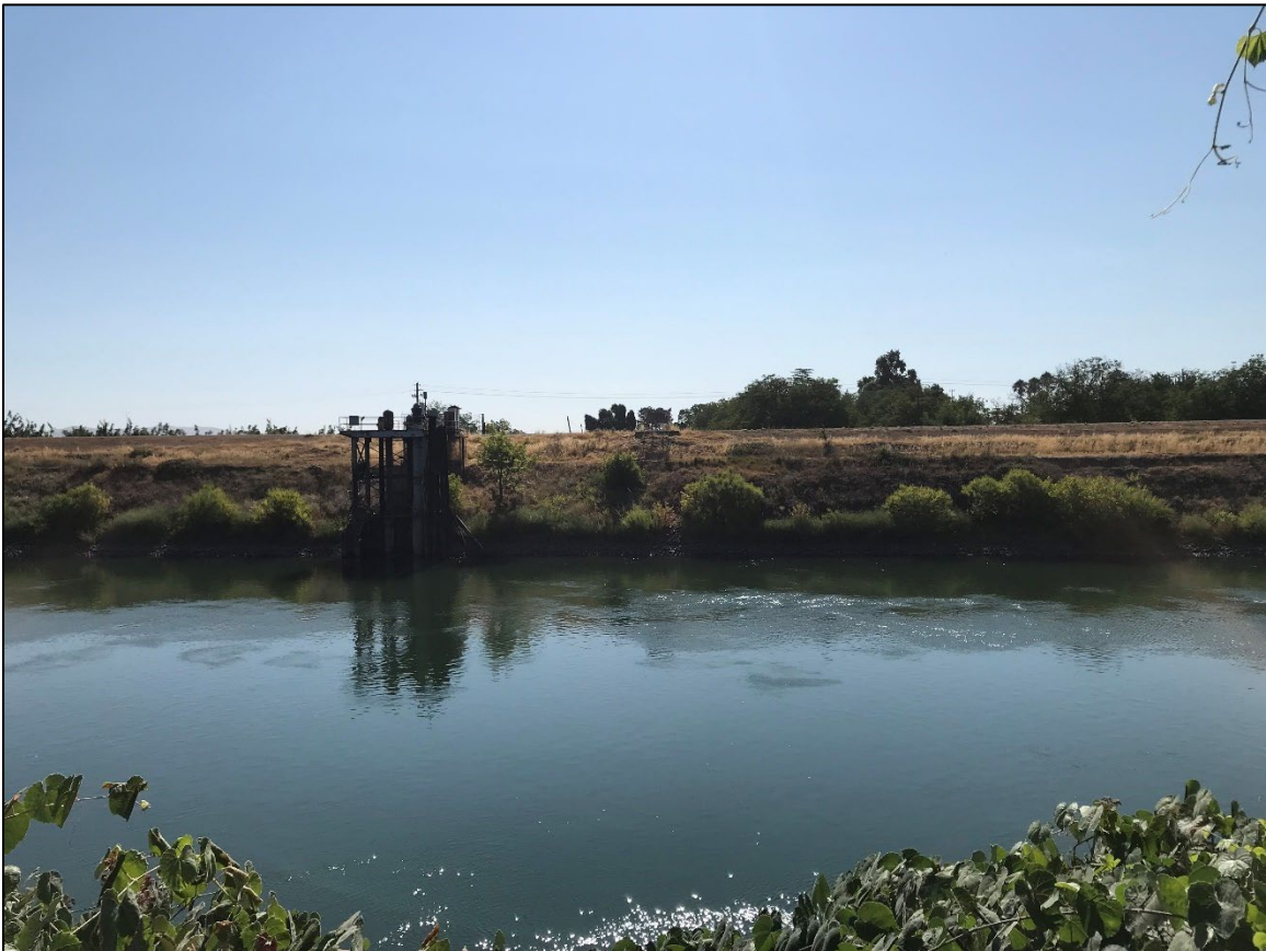
Figure 2-14. Photograph of Segment 4 Pipeline Alignment through East Levee Taken from West Side of Sacramento River
