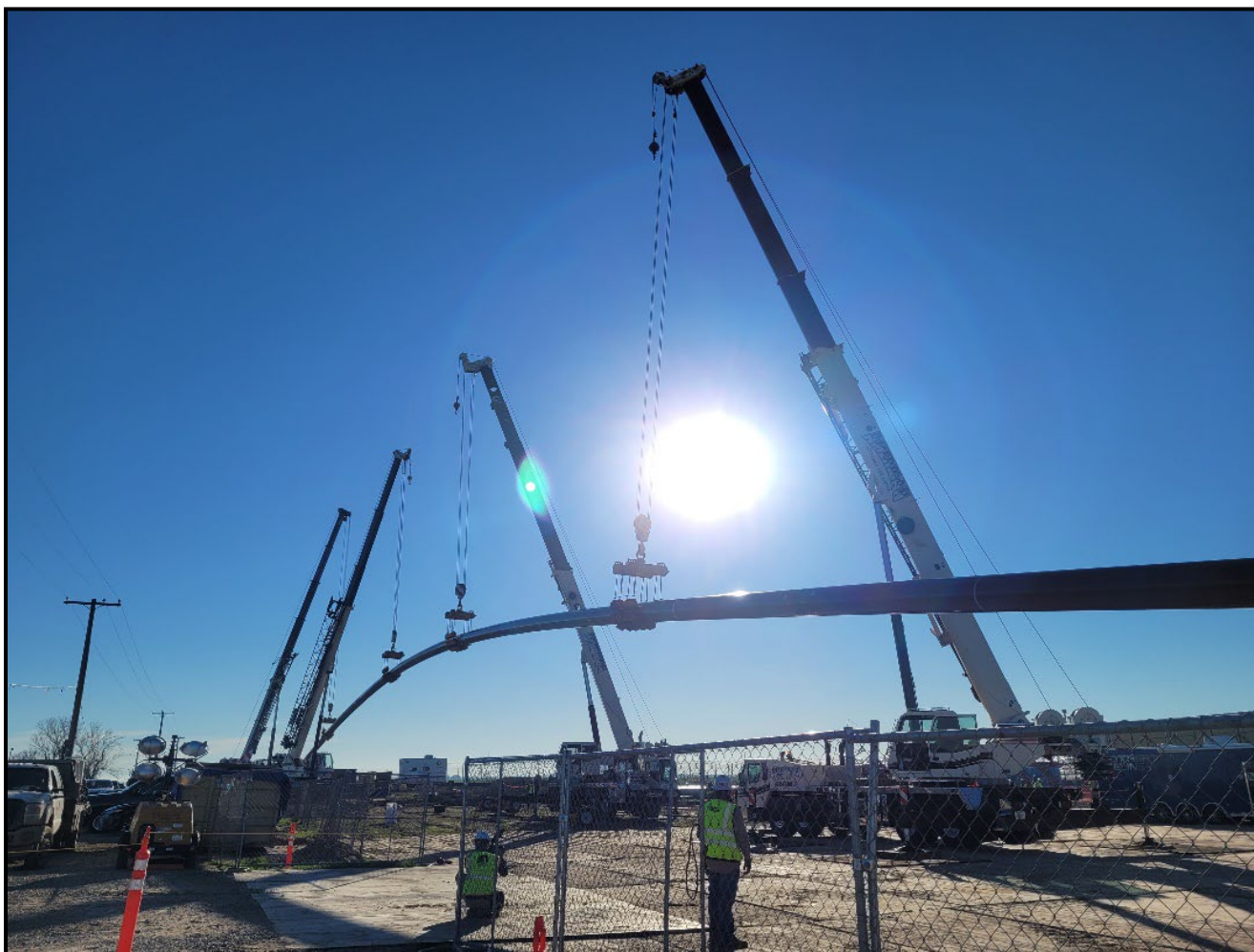
Figure 2-8. Photograph of Side-booms Supporting the Pipeline During Pullback 5
