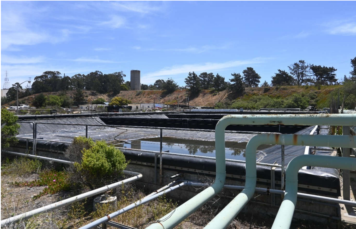
Figure 18 Retaining Basin, Facing East
