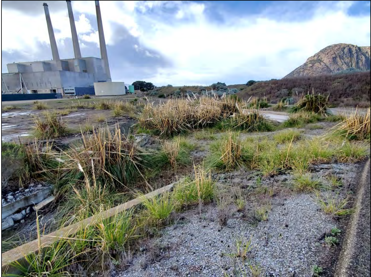
Photo 4: Image viewing south of disturbed areas with concrete and asphalt surfaces. Note invasive pampas grass growing. March 11, 2021
