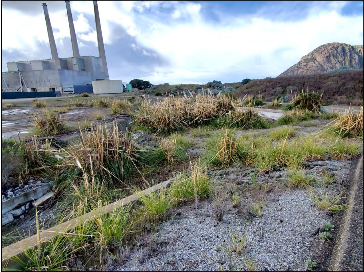
Photo 4: Image viewing south of disturbed areas with concrete and asphalt surfaces. Note invasive pampas grass growing. March 11, 2021
