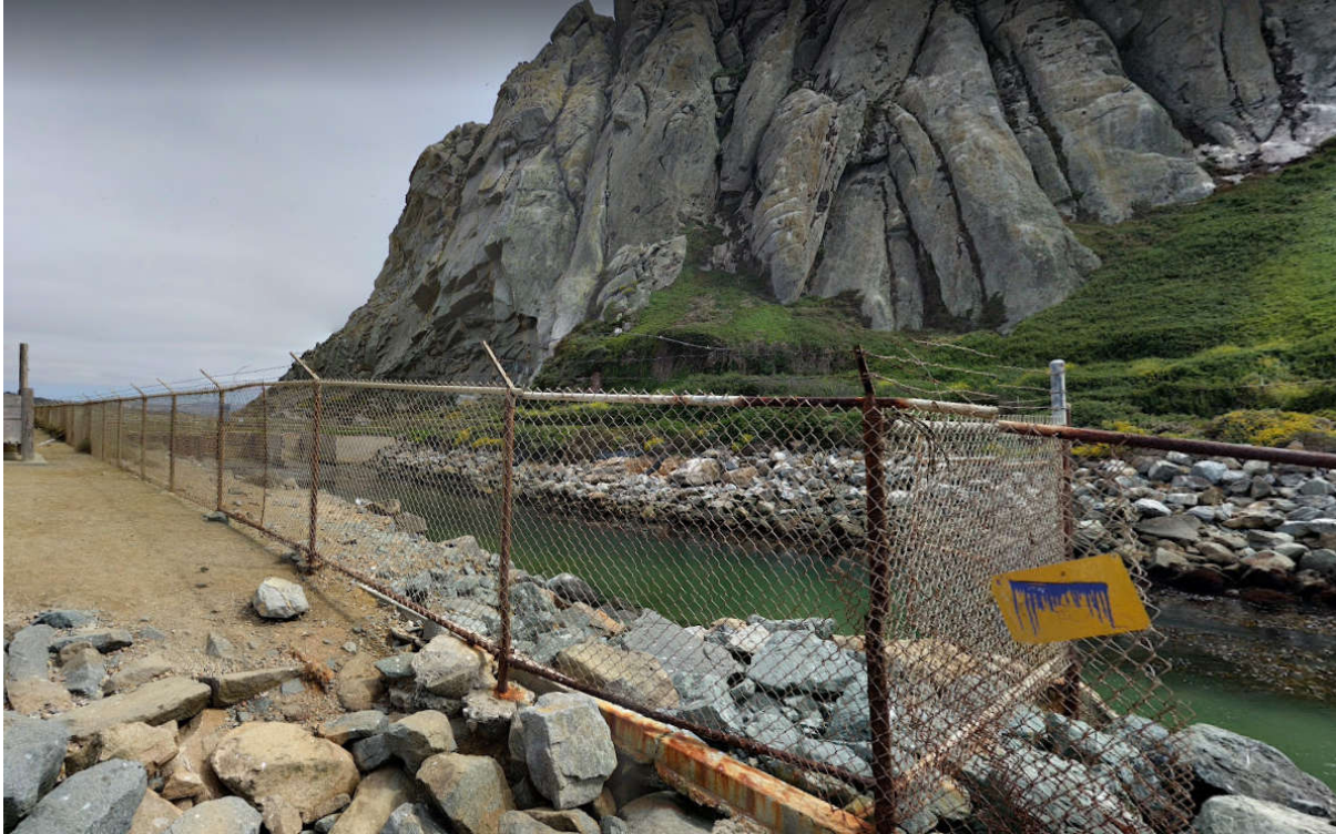
Figure 22 Overview of Cooling Water Discharge Outlet and Channel, Facing South
