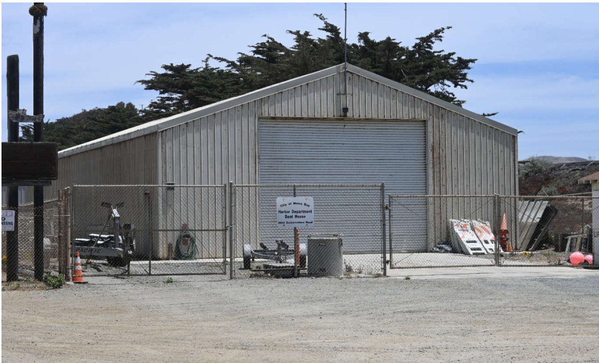
Figure 25 Butler-Type Building at Harbor Department Boat House Facility, North and West Elevations, Facing East
