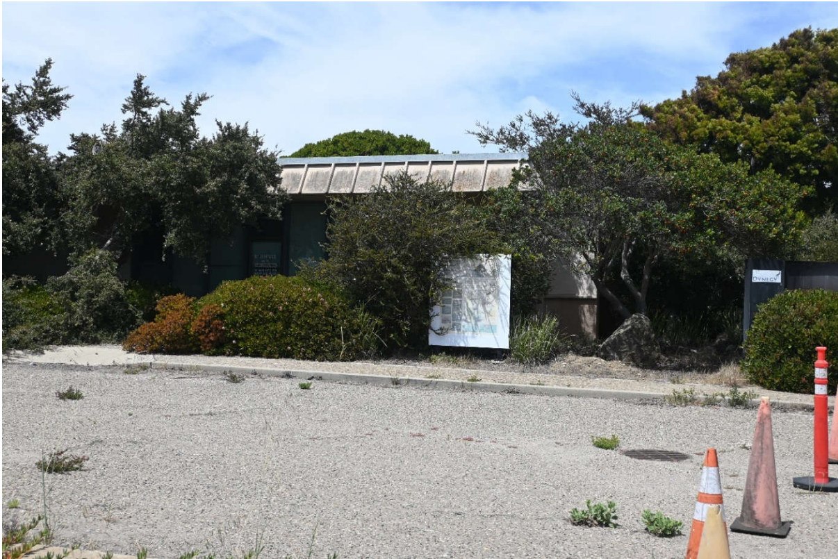
Figure 14 Gatehouse, South Elevation, Facing North
