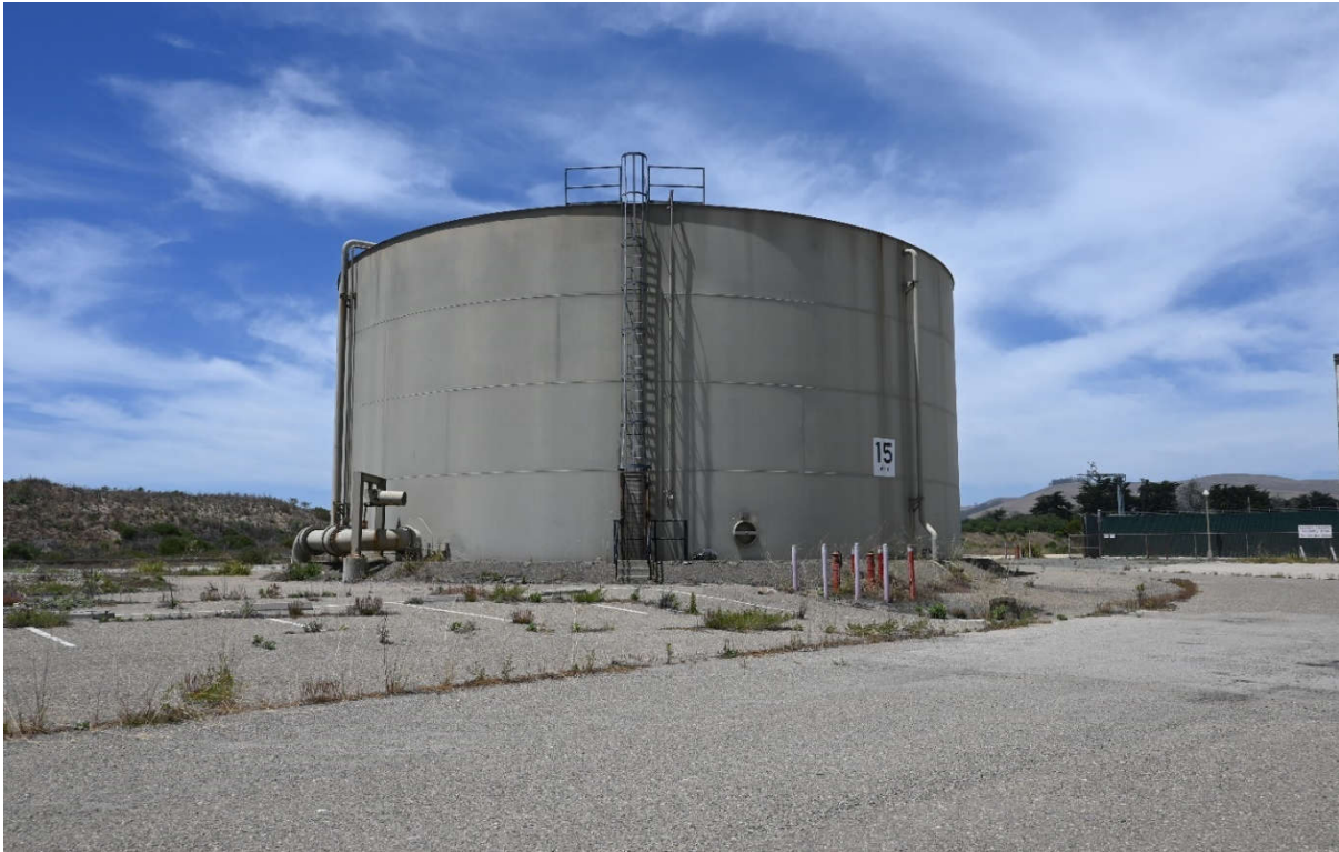
Figure 16 Displacement Oil Tank, Facing North
