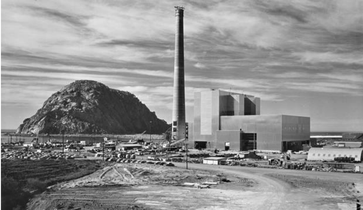
Figure 26 Morro Bay Power Plant Under Construction, 1954
