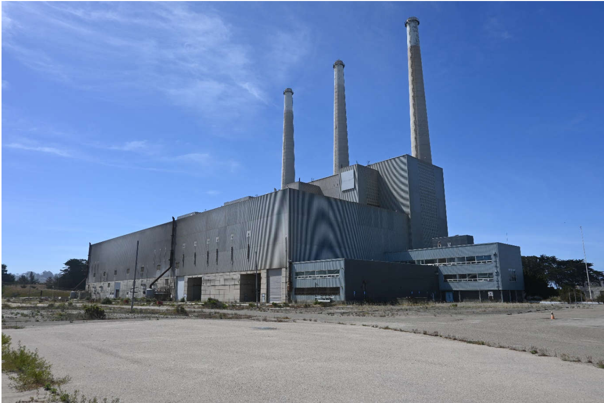
Figure 6 Overview of Generating Plant, North and West Elevation, Facing Southeast
