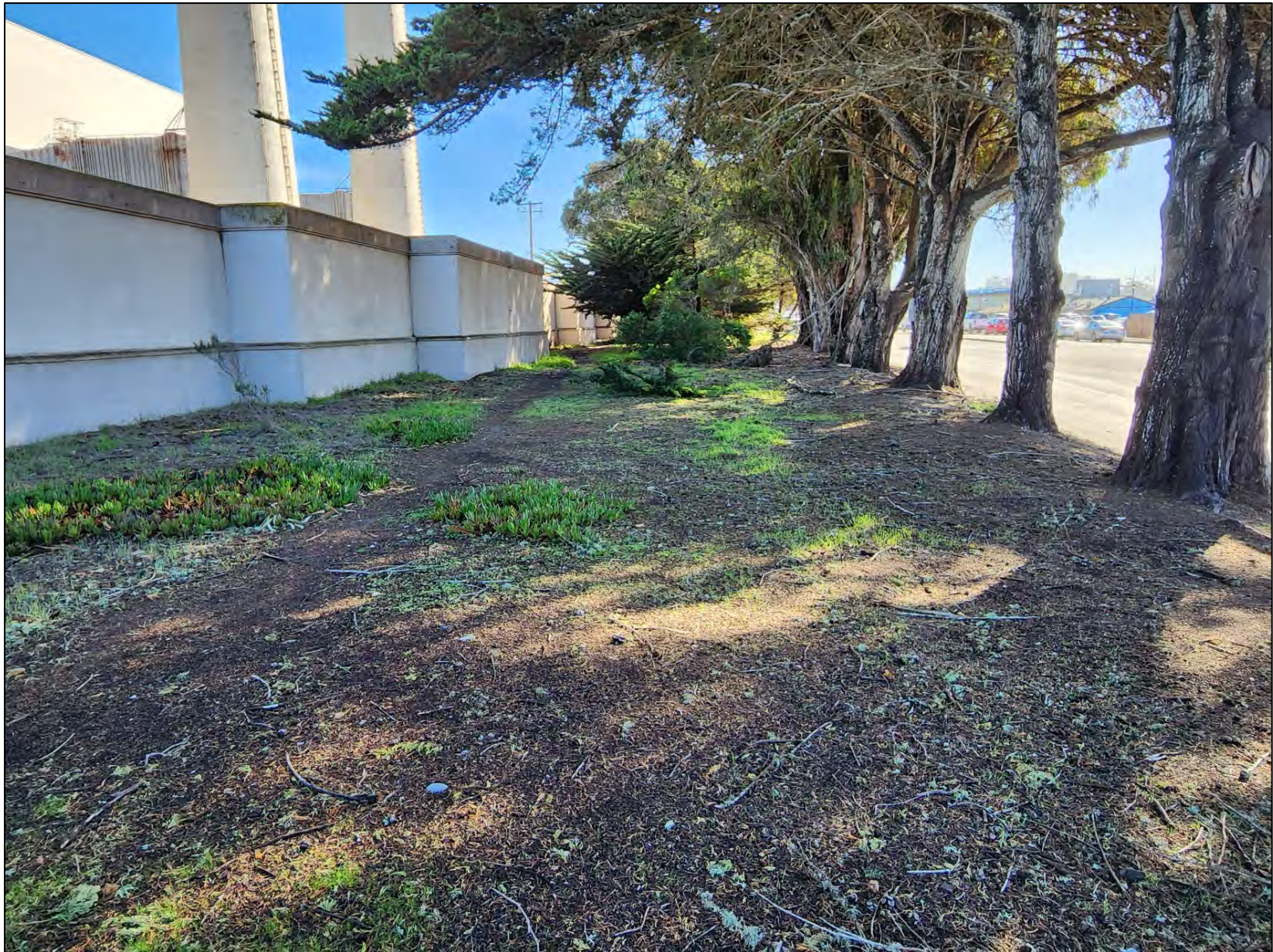
Photo 4: Image viewing southeast along the power plant's perimeter wall. December 28, 2022
