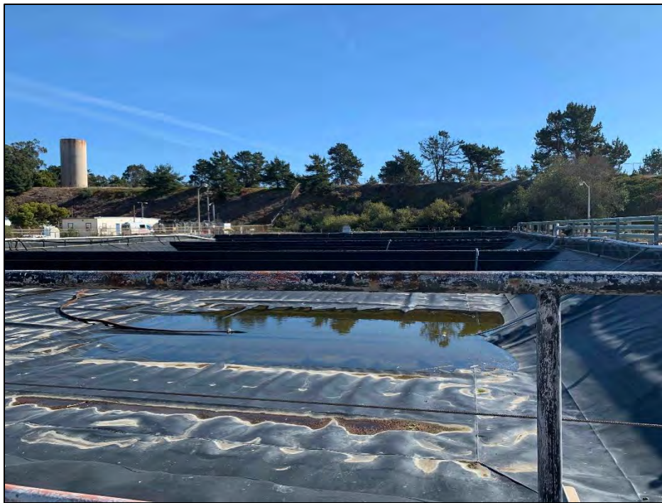
Photograph 7. Current MBPP infrastructure, ponded water visible (aspect: southeast; December 16, 2020).
