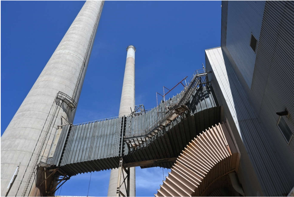
Figure 12 Gas Duct Adjoining Unit 4 Boiler Stack, Facing West
