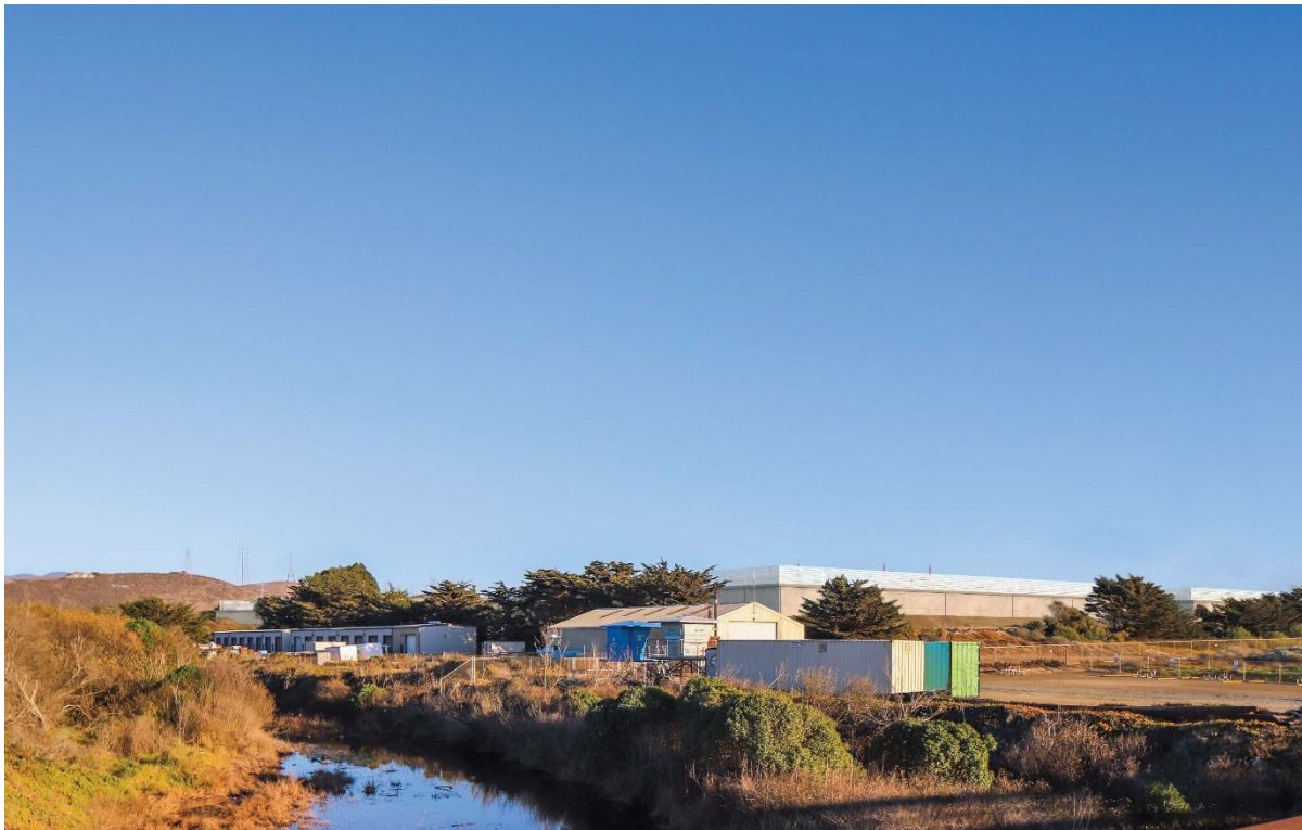
Simulated View 3. Simulated view after construction of the BESS and demolition of the power plant building and stacks.
