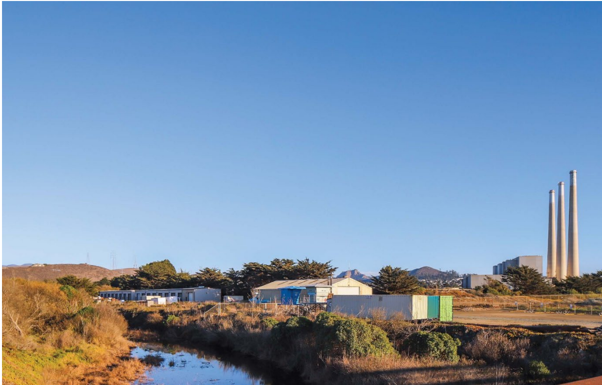
Photograph 3. Existing view looking southeast from bicycle bridge.
