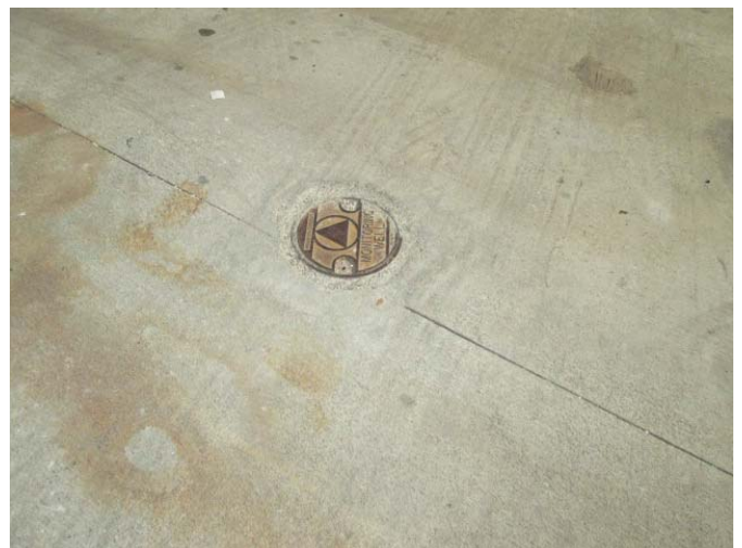
Picture 24 – Methane monitoring well south of building #4
