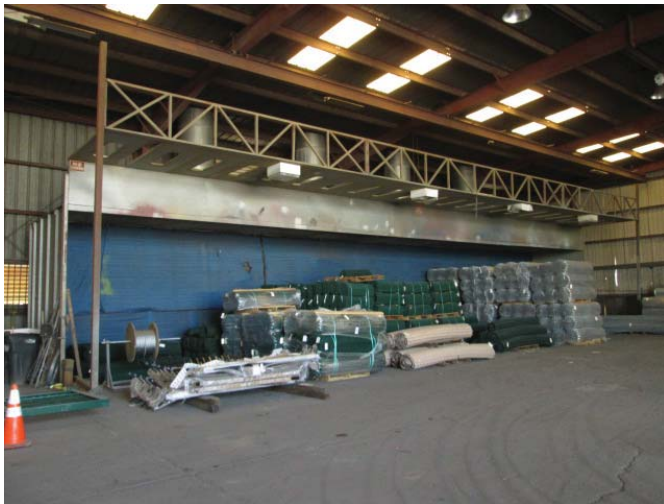
Picture 20 – Building #2 spray paint booth
