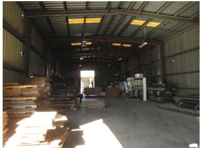
Picture 5 – Interior of building #3 looking west
