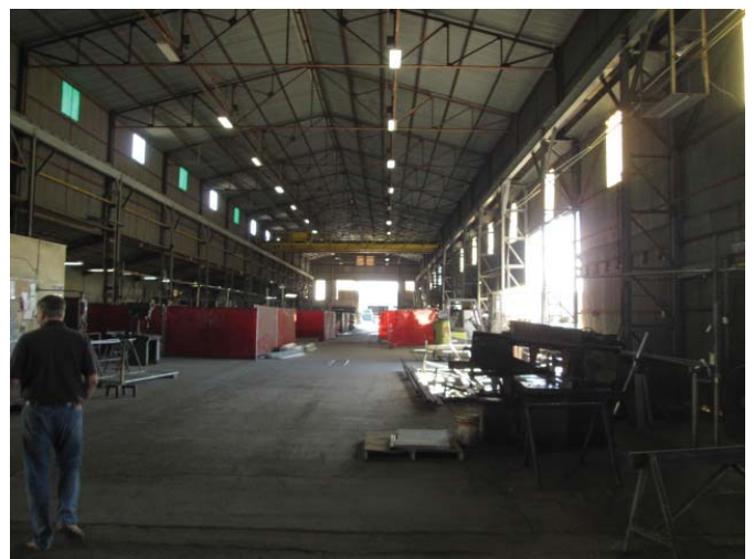
Picture 12 – Interior of building #1
