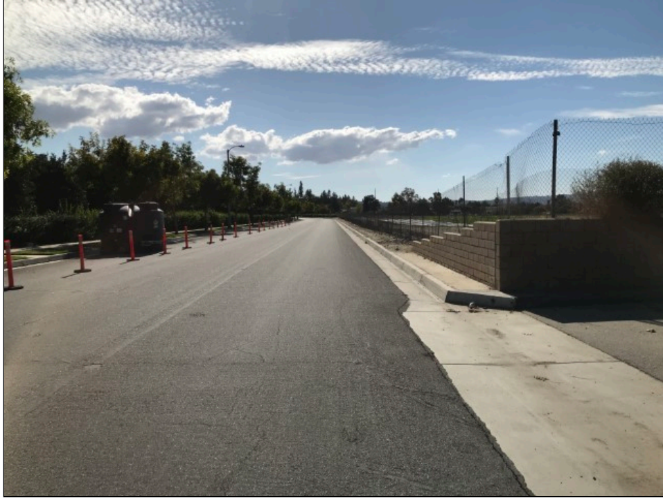
Photo 7: View of the eastern portion of the subject property, facing south.
