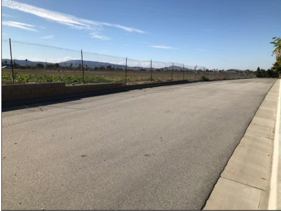
Photo 3: View of the northern portion of the subject property, facing west.
