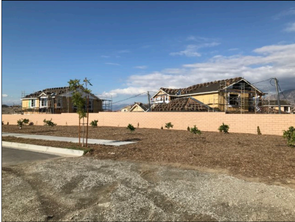
Photo 20: View of the residential construction lots adjoining to the northwest.
