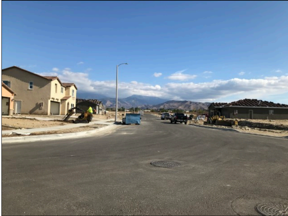
Photo 22: View of the residential construction lots adjoining to the west.
