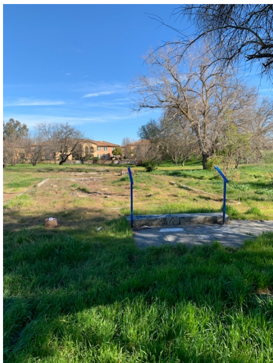
Foundation A, view easterly
