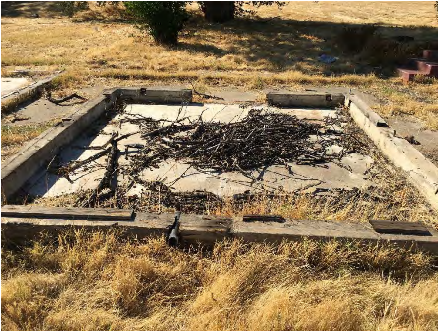
Photo 9: View of a small foundation or platform in between buildings. One possible drain pipe observed in the wood frame.
