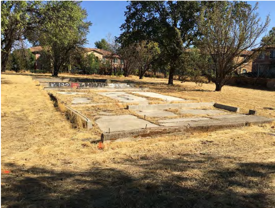
Photo 7: View of the eastern most foundation observed on Site, facing northeast.
