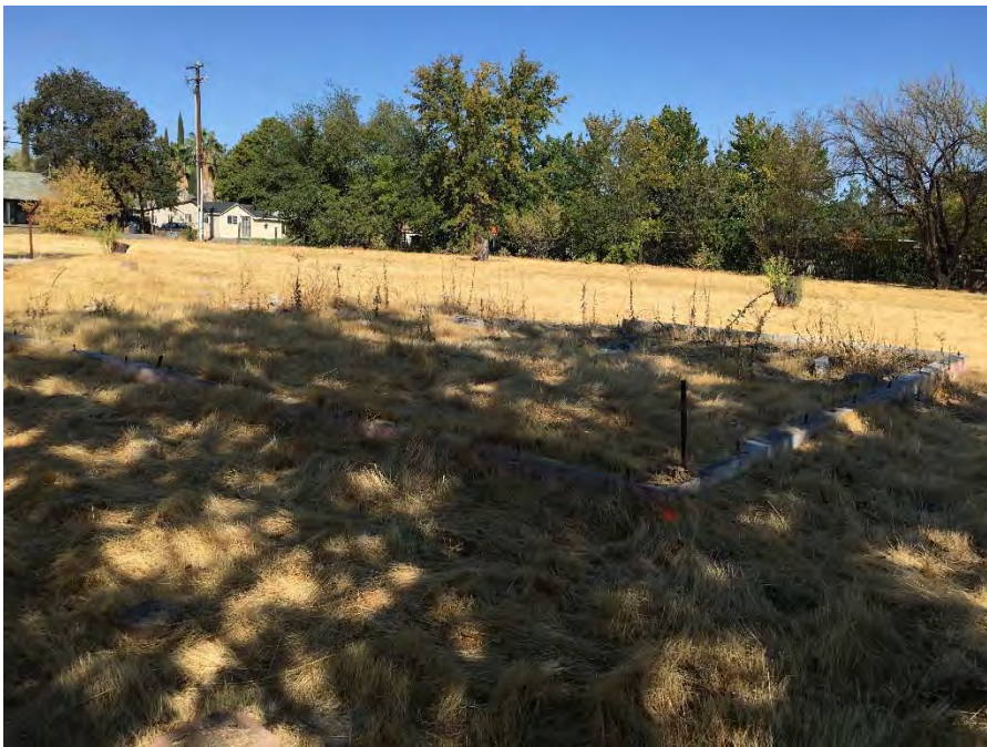
Photo 10: View of western most foundation observed on Site, facing northwest.
