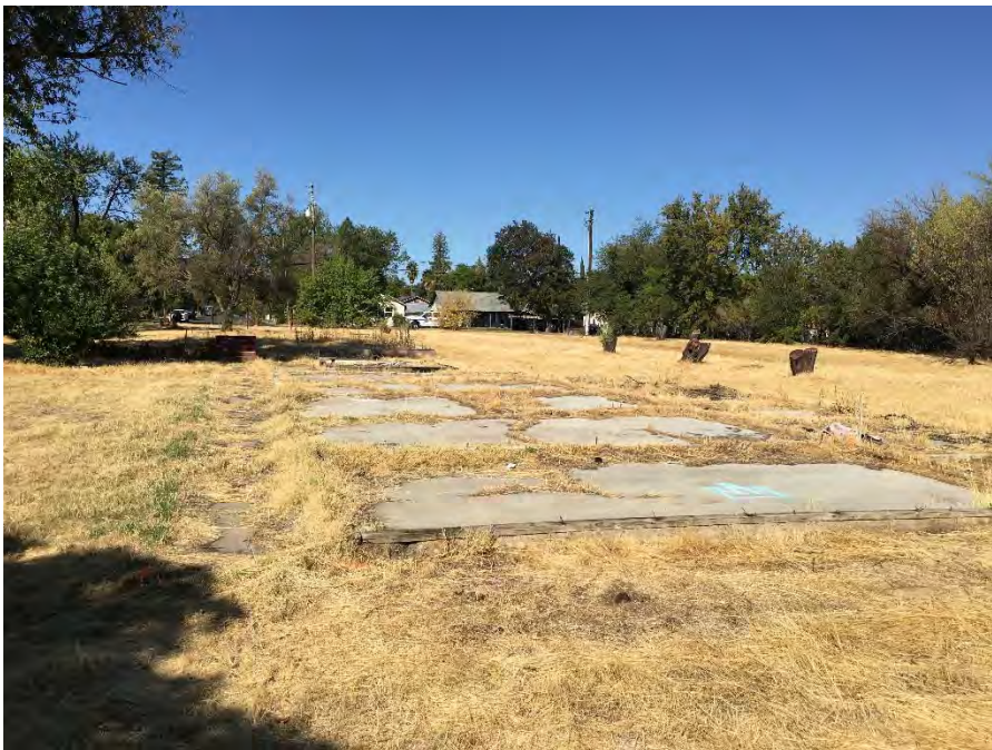
Photo 8: View of the center foundation observed on Site, facing west.
