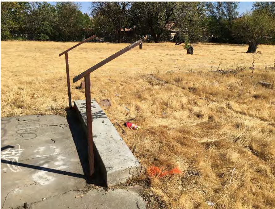
Photo 12: Unknown feature on edge of western most foundation on Site.
