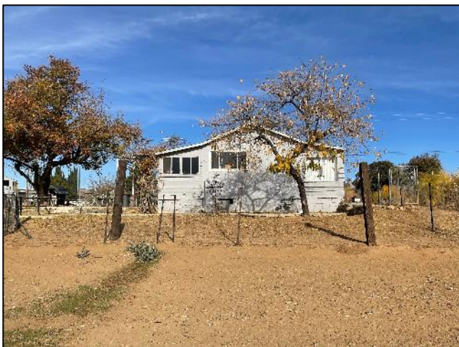
Figure 23. Overview of Structure B, facing north
