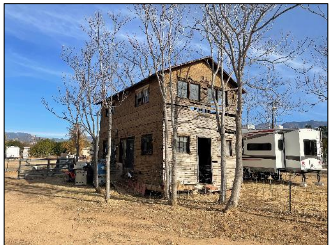
Figure 24. Overview of Structure C, facing northeast
