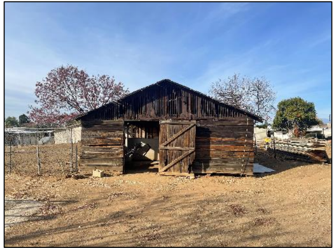
Figure 22. Overview of Structure A, facing west
