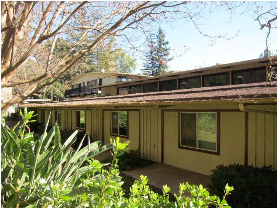
Photograph 8. Rear (west) elevation showing clerestory windows and replaced vinyl windows, view to northeast
