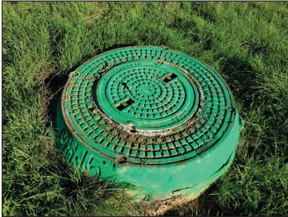
View of manhole cover.
