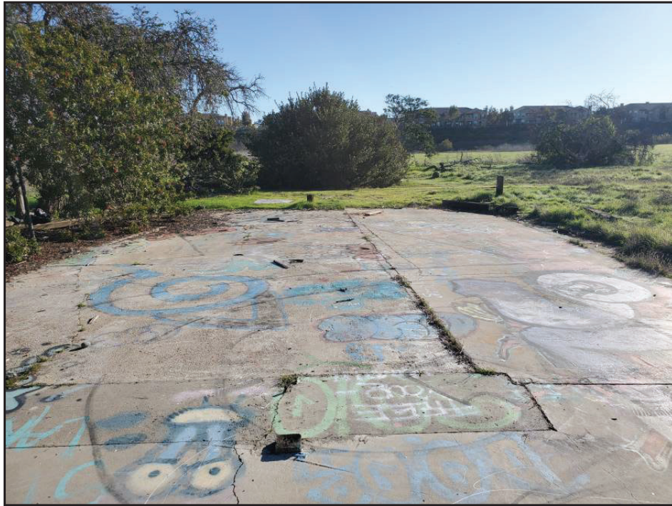
View of former building pads.
