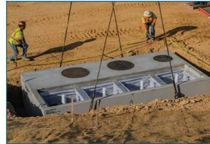
The Modular Wetlands® is simple, easy to install, and has a space-efficient design that offers lower excavation and installation costs compared to traditional tree-box type systems. The structure of the system resembles precast catch basin or utility vaults and is installed in a similar fashion.
