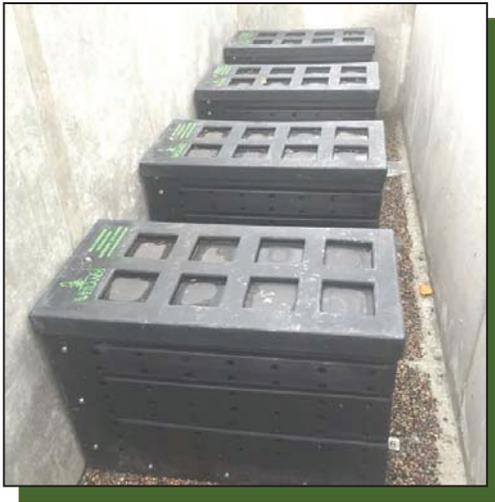
Pre-filter cartridges with tops on.
