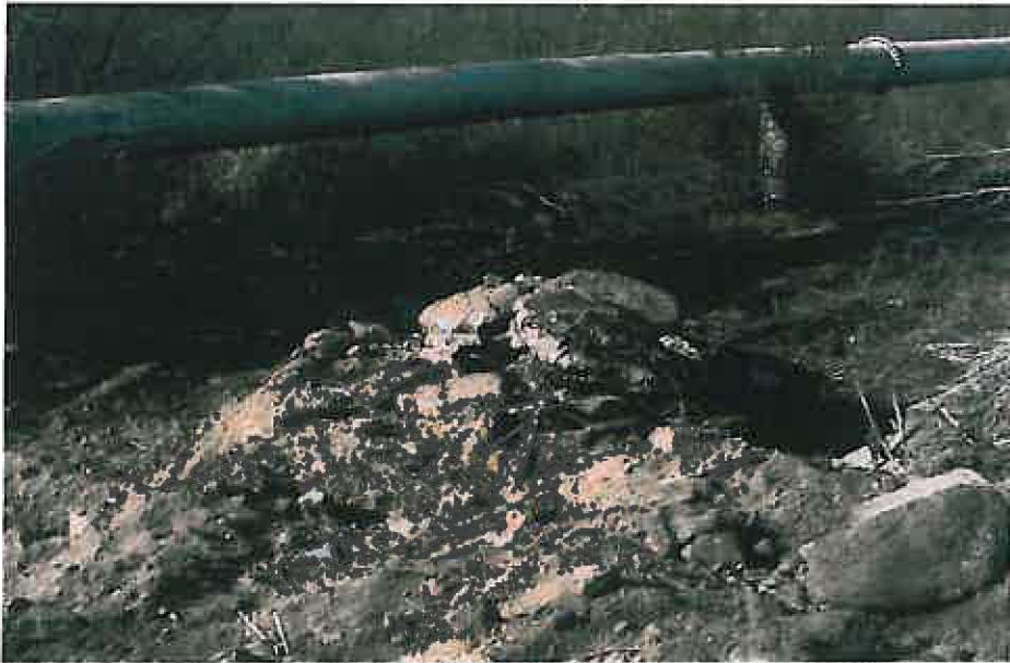
13. Concrete construction debris in the river on the northwestern portion of the Property.
