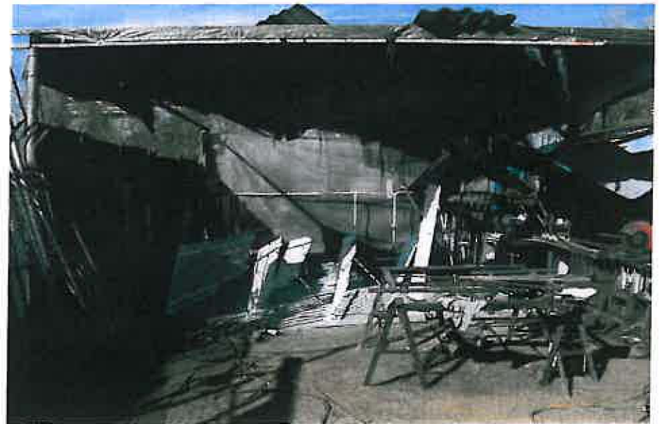
12. Paint spray area at Monroy's Towing on the western portion of the Property.
