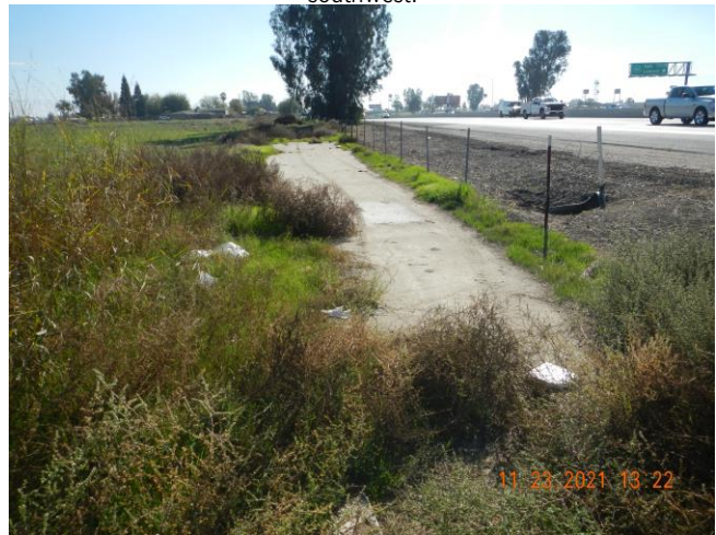
Photograph 4: General view from the northwest corner facing south.
