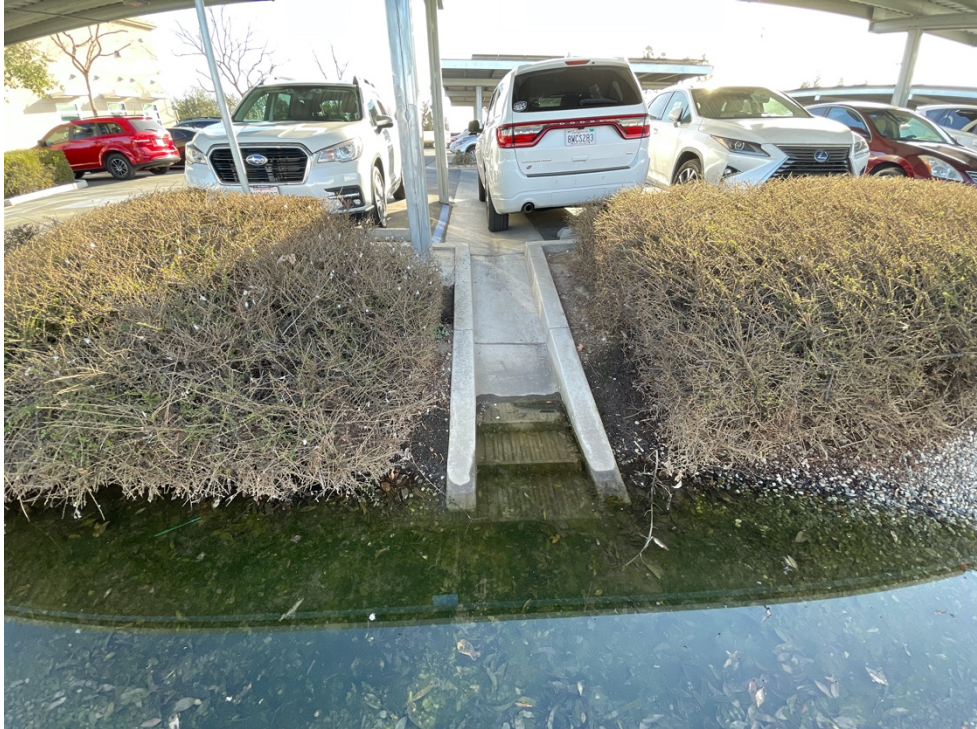
Photo 5. View of curb cut leading from parking facilities to ditch in northern portion of the project buffer, facing north. February 21, 2022.
