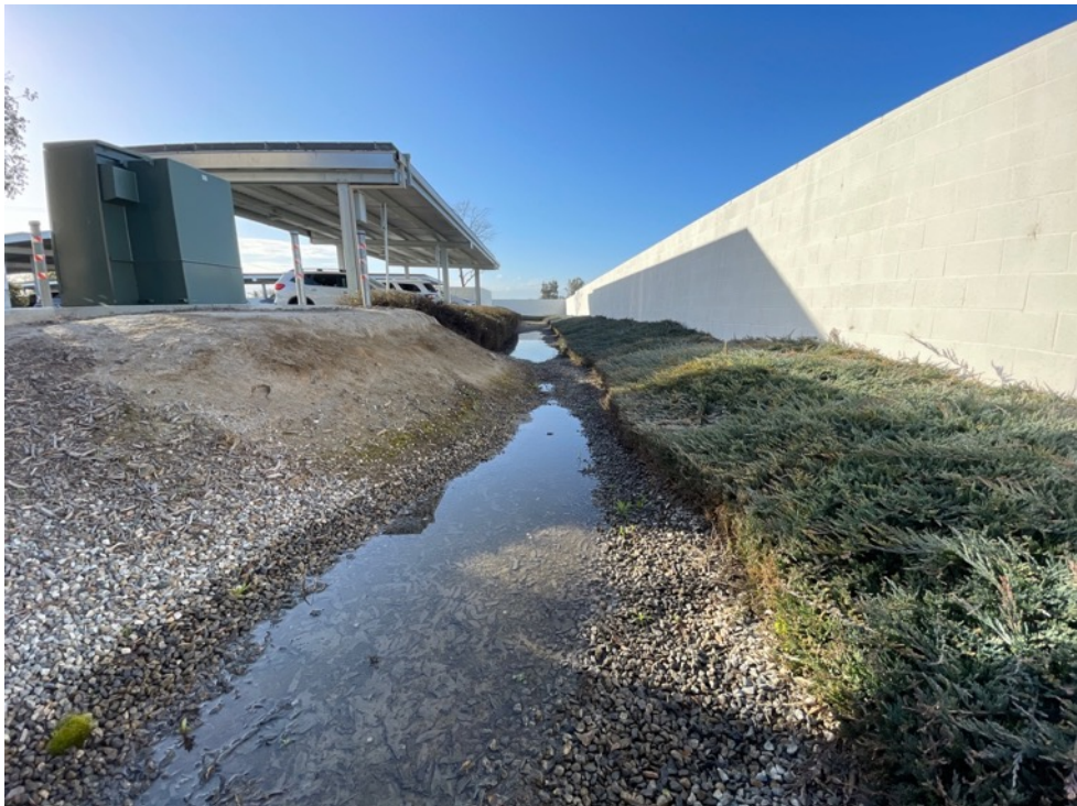
Photo 4. View of ditch in northern portion of the project buffer, facing south. February 21, 2022.
