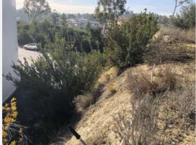
Photo 2. Top of hillside, facing west towards the proposed pump station location.
