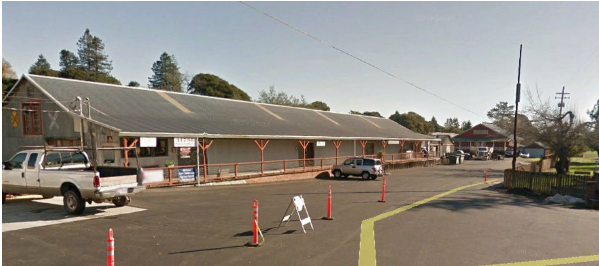
Figure 4.1-41 PEN-1, PEN-3, and PEN-8 Looking Southeast
