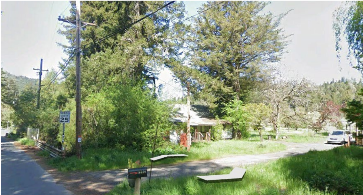
Figure 4.1-6 GUE-4 from Laughlin Road, Looking North
