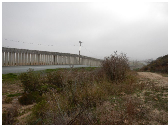
BS-P2: View east/downstream of BS-Ditch 2
