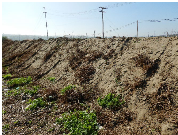
TRF-P10: View east of floodplain berm
