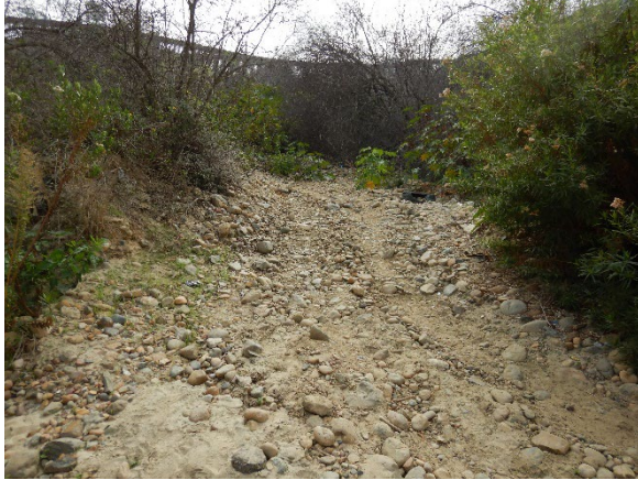
GC-P3: View of access road/ATV track on river left
