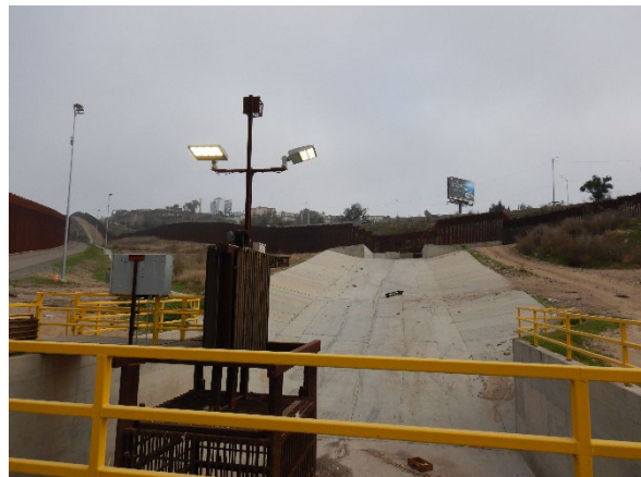
BS-P6: View south of Canyon Drain 1
