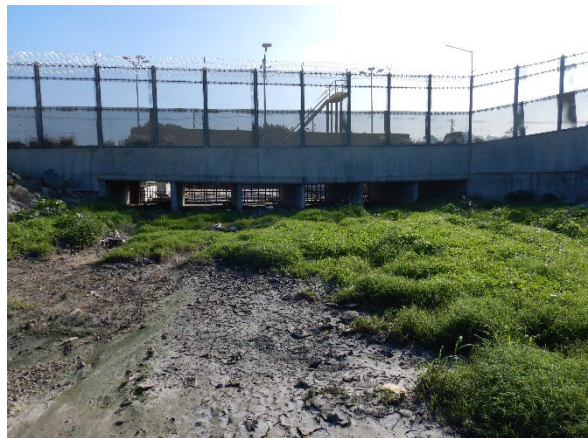
TRF-P17: View south of Stewart's Drain box culverts
