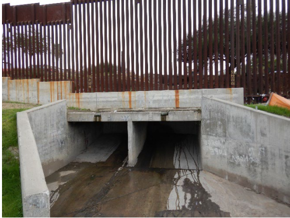
BS-P3: Box culverts of Silva Drain
