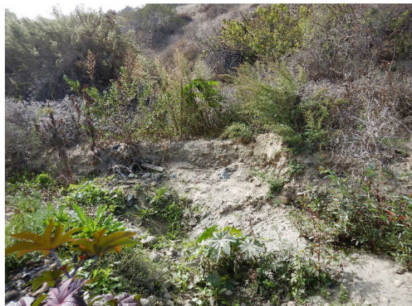
SG-P6: View west near road crossing, benching and vegetation in channel
