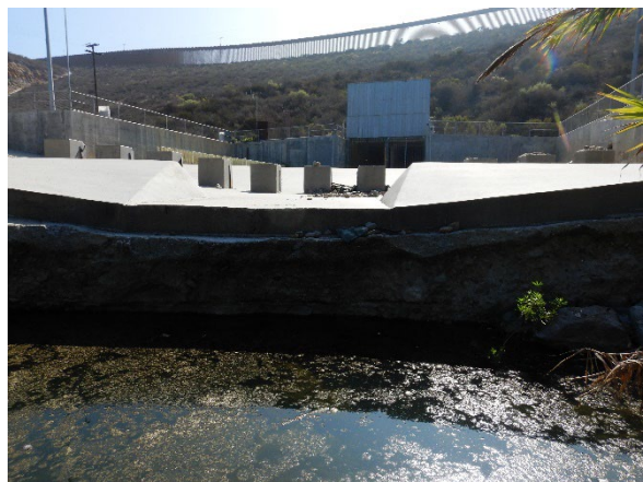
SG-P2: View South of drain at border
