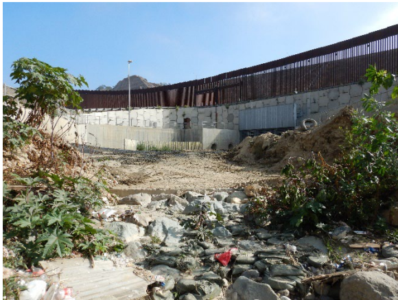
GC-P1: View south of border wall and canyon collector
