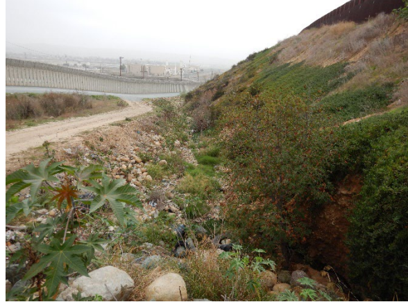
BS-P4: View east/downstream of BS-Ditch 1
