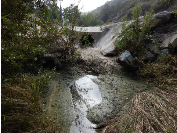
SG-P7/P8: View south of culvert under Monument Road and downstream channel
