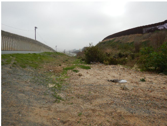
BS-P5: View from upstream of BS-Ditch 2
