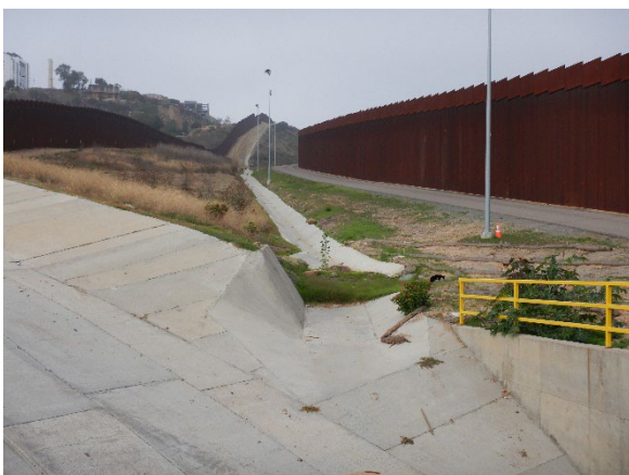
BS-P7: View west of concrete v-ditch near Canyon Drain 1
