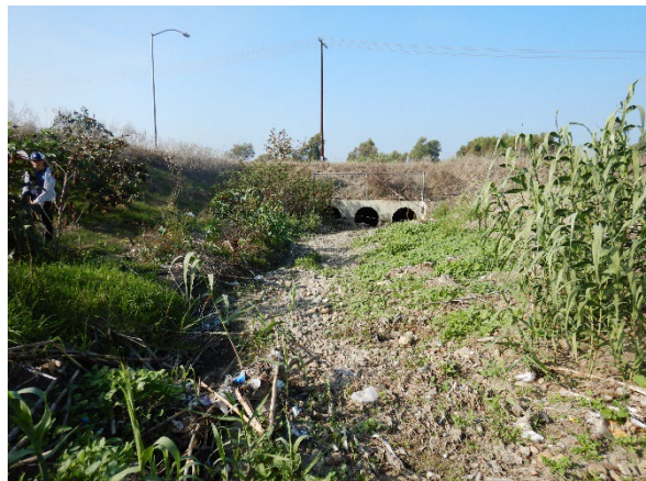
CS-P2: View north/downstream of Clearwater Swale 1 toward Dairy Mart Rd culverts
