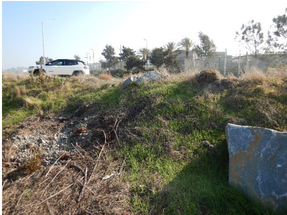
CS-P1: View upstream/southwest of culvert (Clearwater Swale 1)
