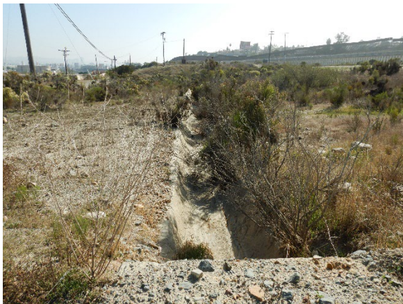
BS-P10: View northwest of v-ditch adjacent to Monument Road
