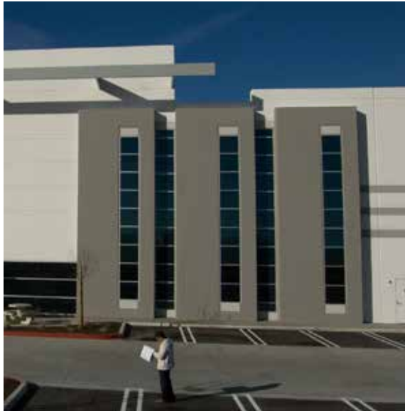
Windows can be used in a variety of shapes and arranged in a pattern to break up a long building plane.
