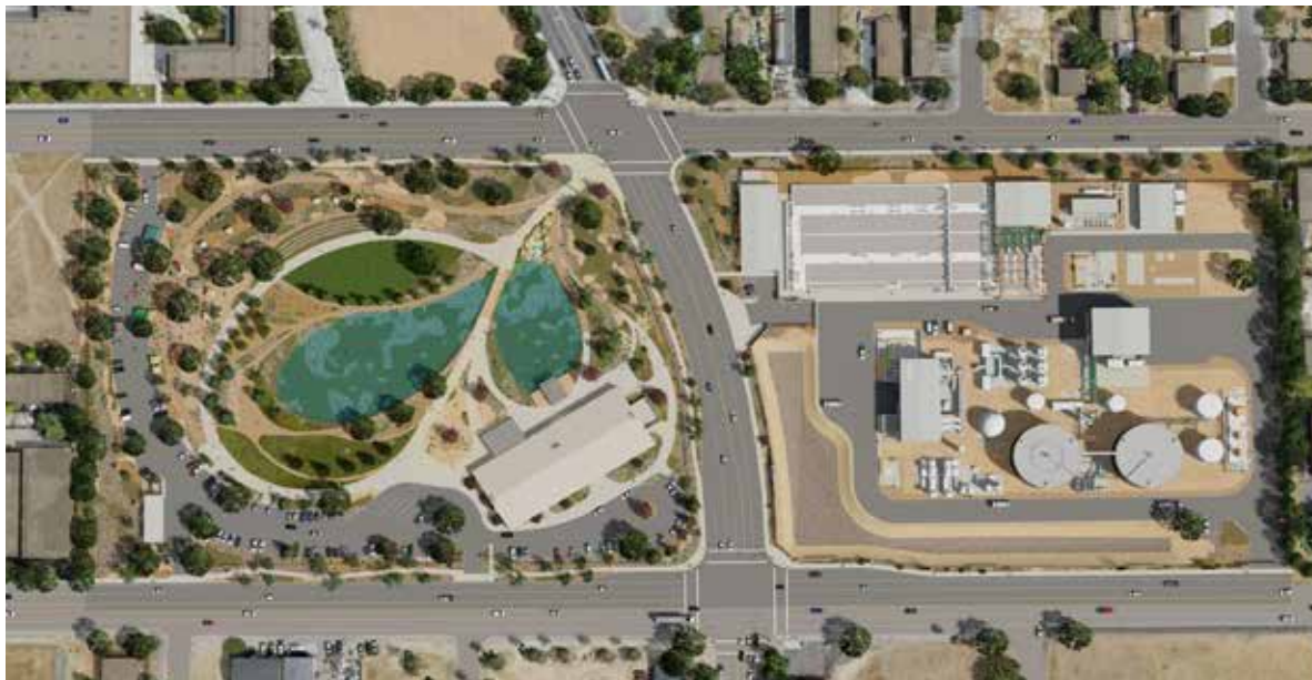
The Sterling Natural Resource Center is a recycled water facility currently under construction adjacent to the AGSP Project Area. Source: EVWD, 2020
