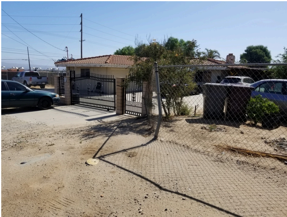
26. West adjoining residence
