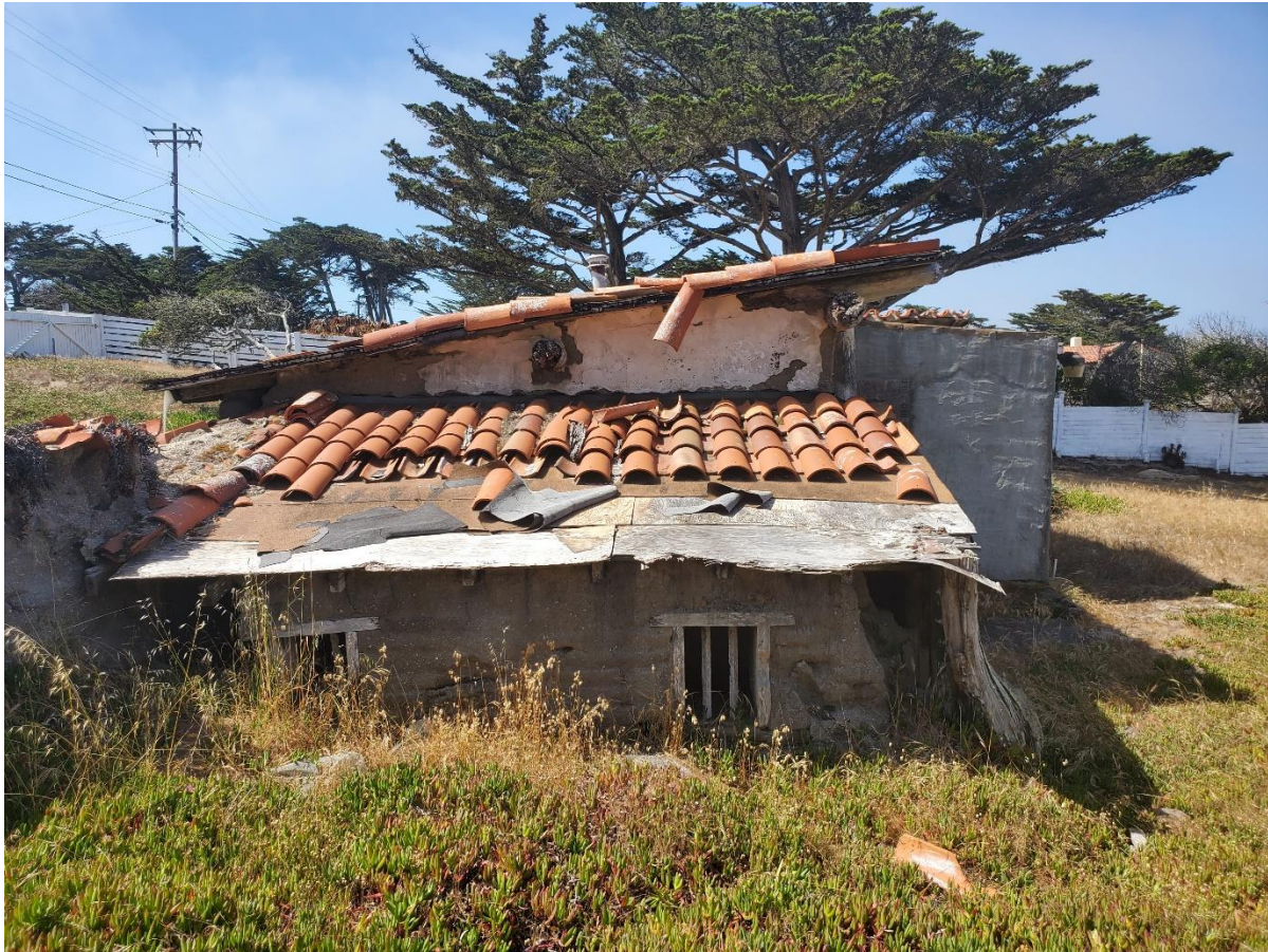
Figure 9 North Elevation of Accessory Building, View South
