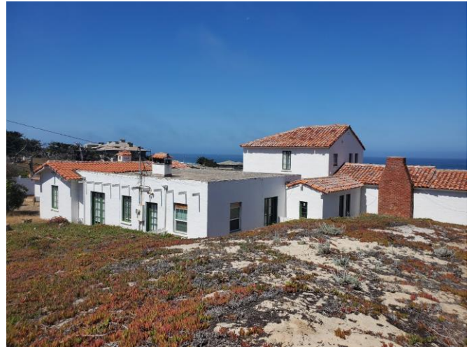
East and North Elevation, View Southwest
