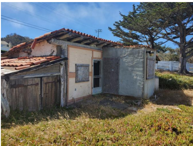
West Elevation of Accessory Building, View Southeast
