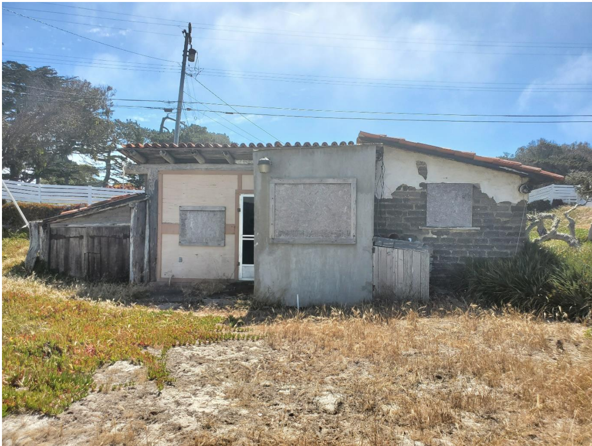
Figure 6 West Elevation of Accessory Building, View East
