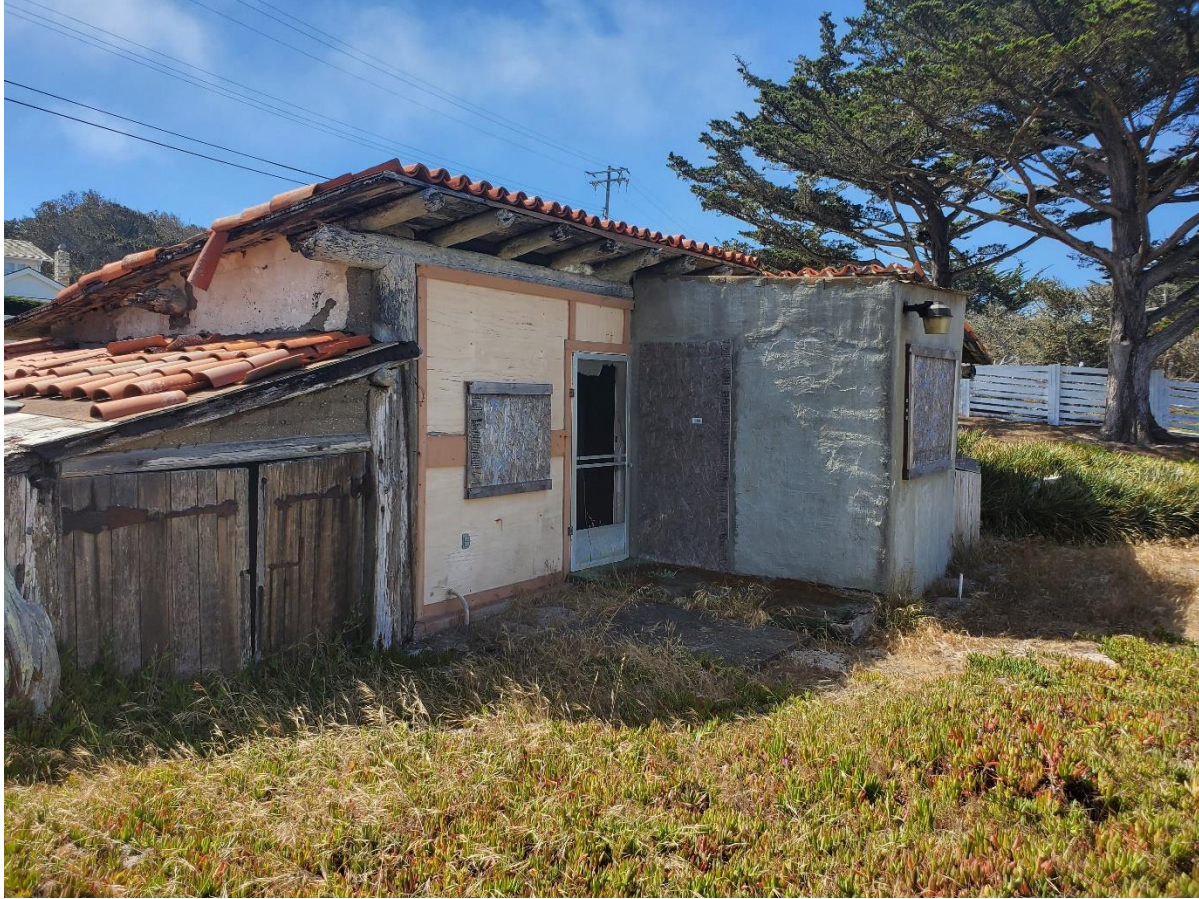
Figure 7 West Elevation of Accessory Building, View Southeast
