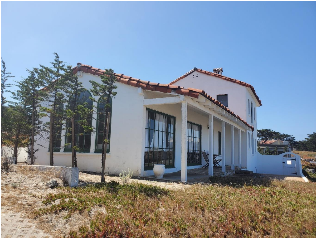
Figure 5 North Elevation of 1661 Sunset Drive, View Southeast
