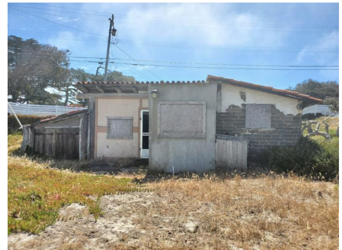
West Elevation of Accessory Building, View East
