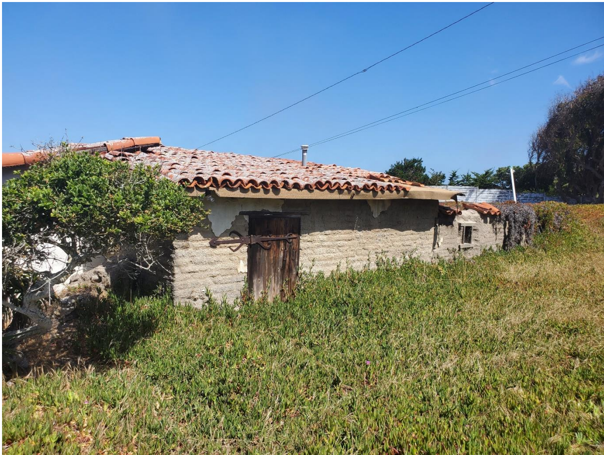
Figure 8 East Elevation of Accessory Building, View Northwest
