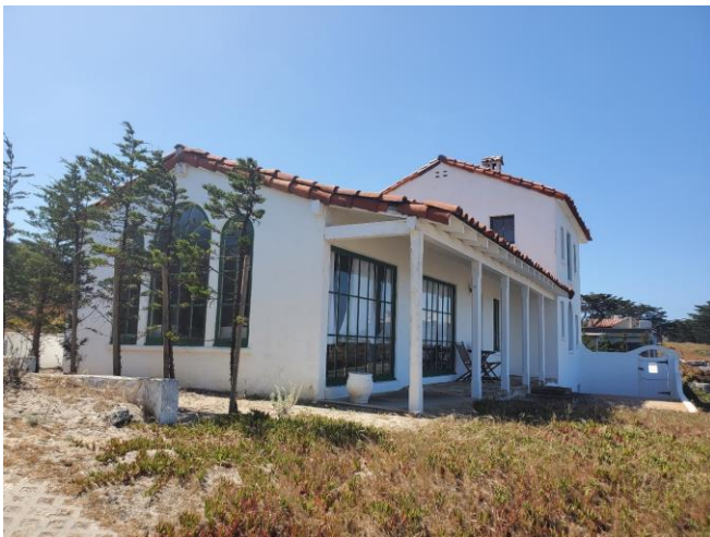
North Elevation of 1661 Sunset Drive, View Southeast
