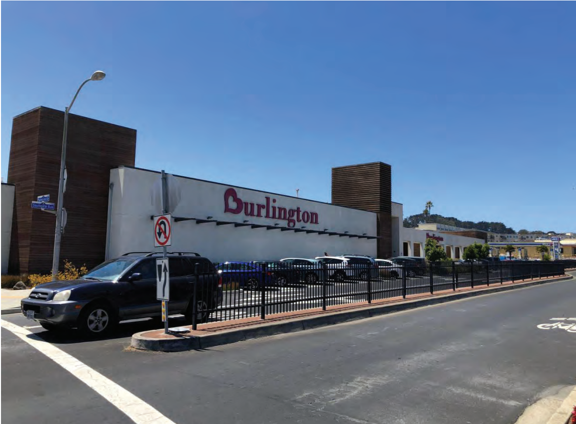
Photo 1: View of existing retail building, looking southwest across Southgate Avenue.
