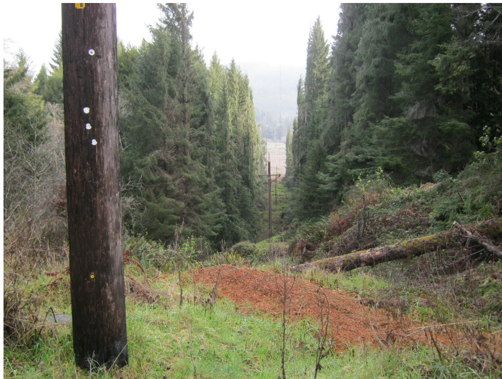
Existing PG&E Powerline
