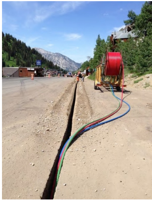
Saw Cut Installation
