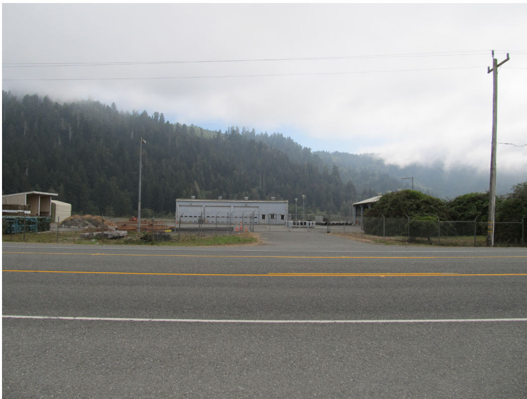
Caltrans Storage Yard at Highway 101 in Orick
