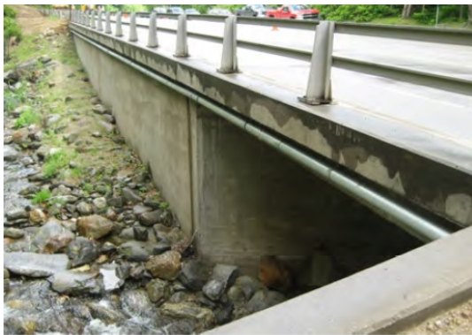
Bridge Hang Installation
