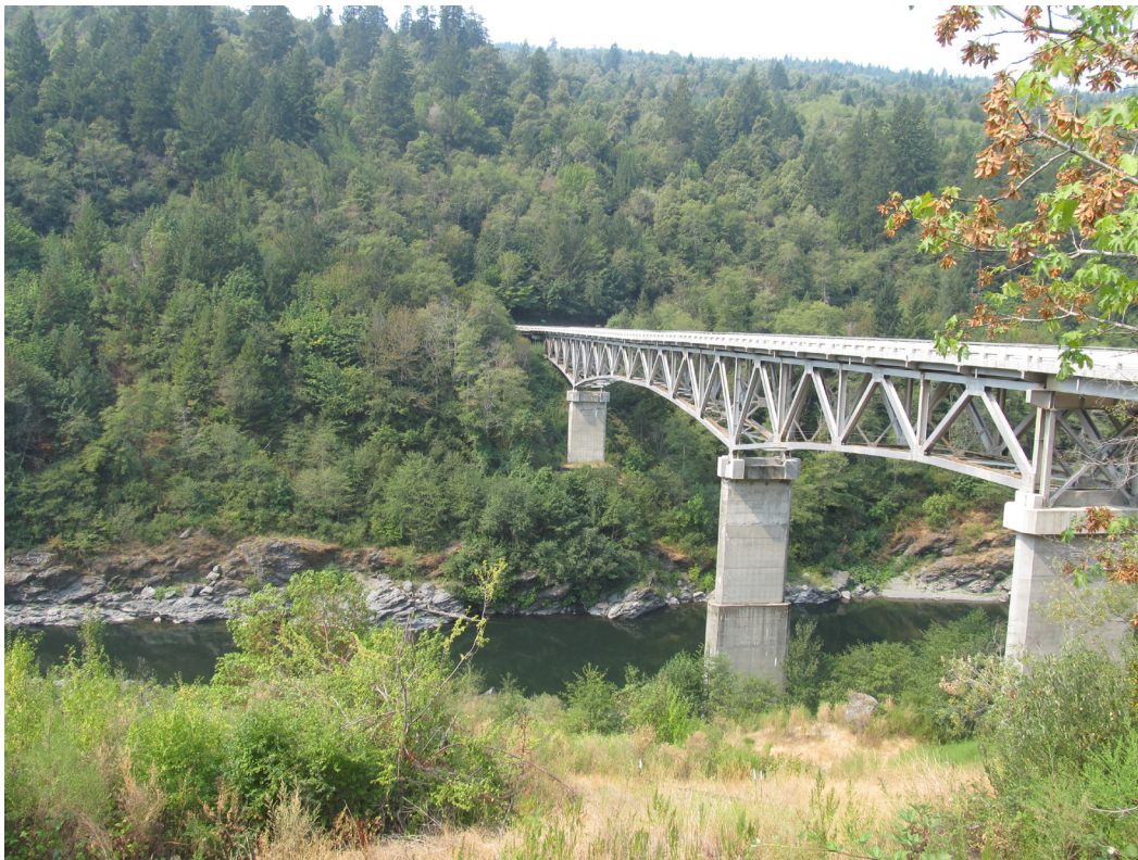
Highway 169 at the Klamath River
