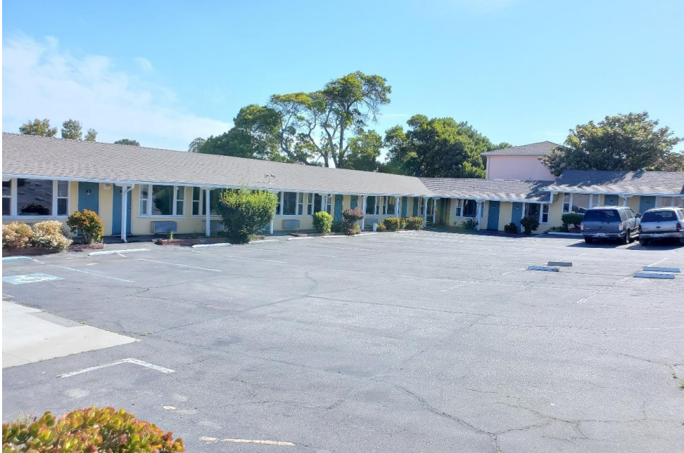
Photo 1: West and South Elevations of guest rooms, Facing Northeast
