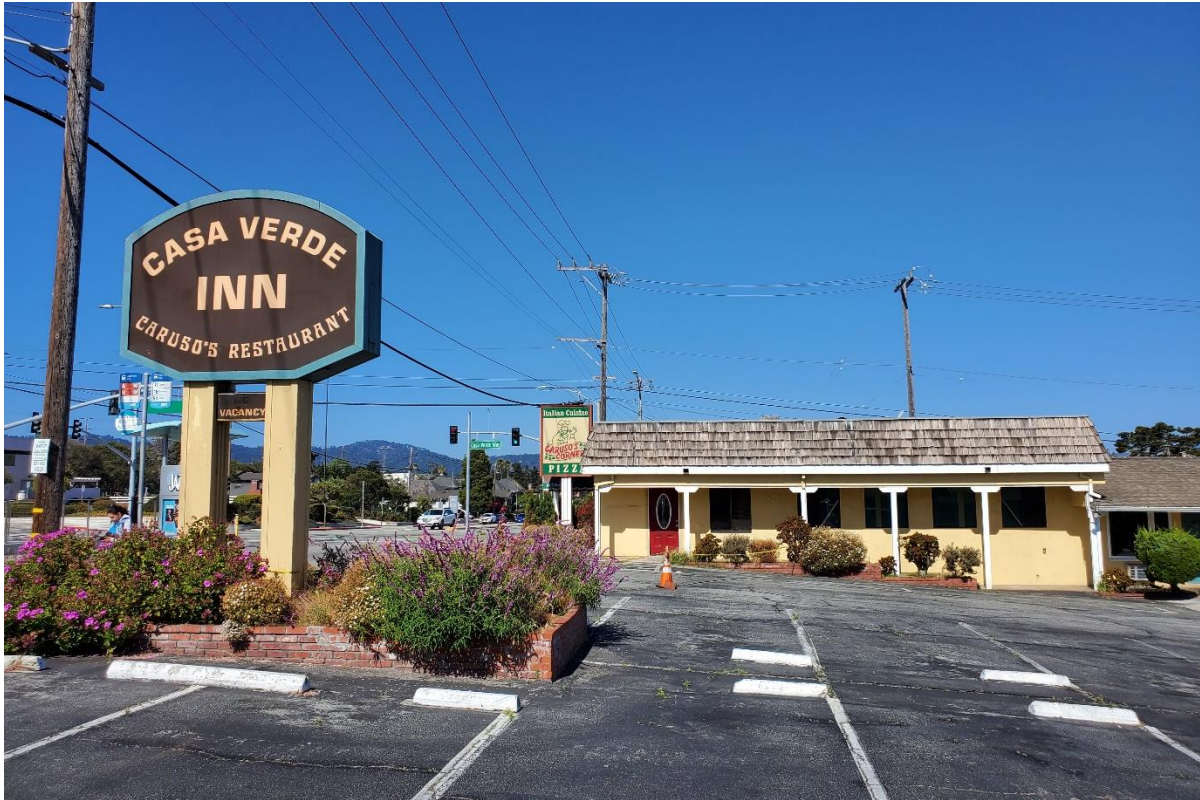
Figure 6 2101 Fremont Street, East Elevation of restaurant and sign, Facing Southwest
