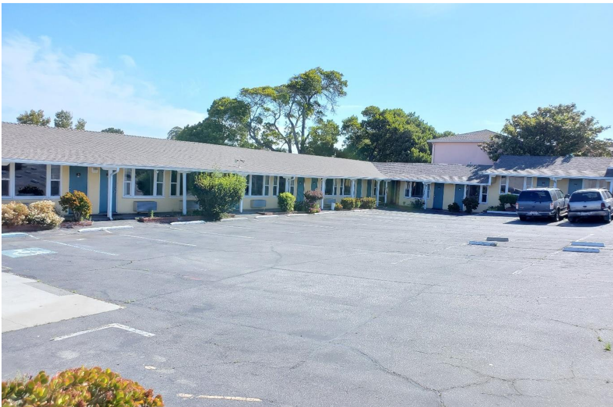
Figure 7 West and South Elevations of guest rooms, Facing Northeast
