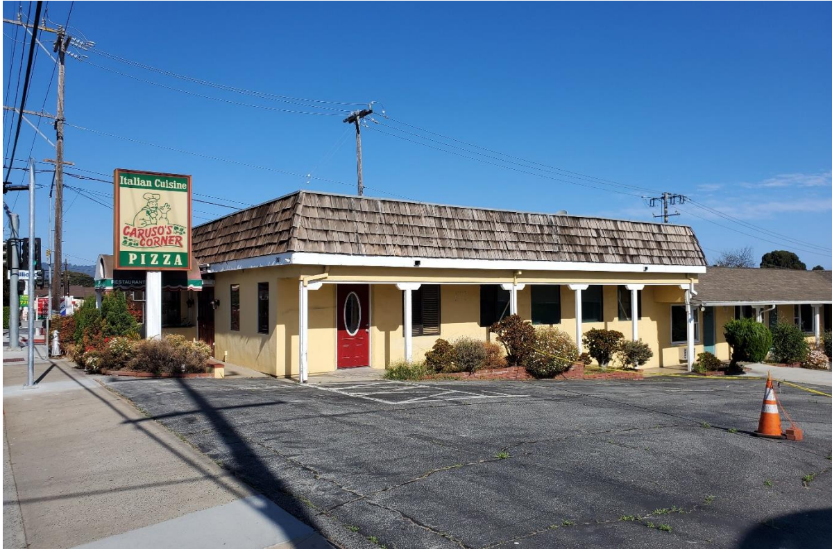
Figure 10 East and South Elevations of restaurant connected to the motel, Facing West
