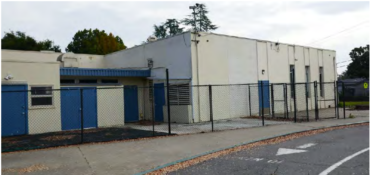
Figure 14. West façade of the multipurpose building. Photograph taken 1/17/2022.
