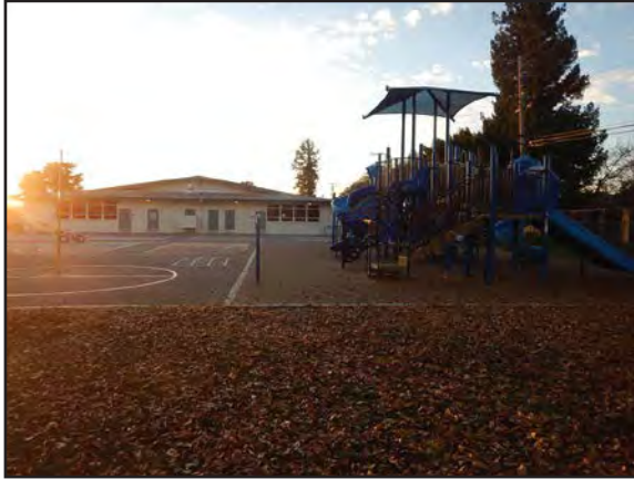
Photograph 1. Laurelwood Elementary overview, facing west.
