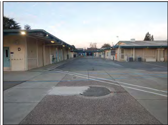
Photograph 4. Laurelwood Elementary overview, facing north.
