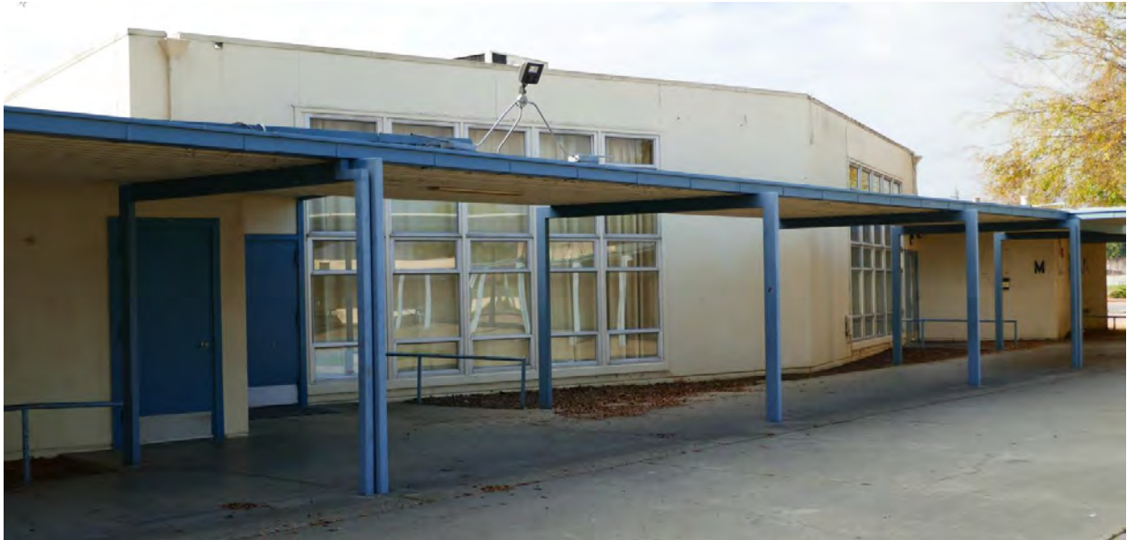
Figure 11. N North façade of the multipurpose building. Photograph taken 1/17/2022.
