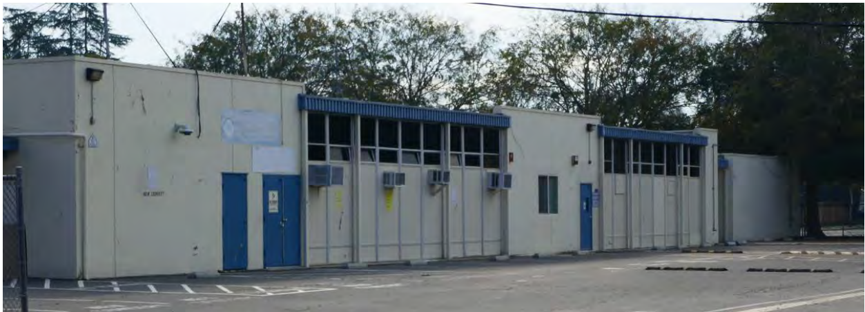
Figure 6. Classroom building A. Camera facing southeast. Photograph taken 1/17/2022.
