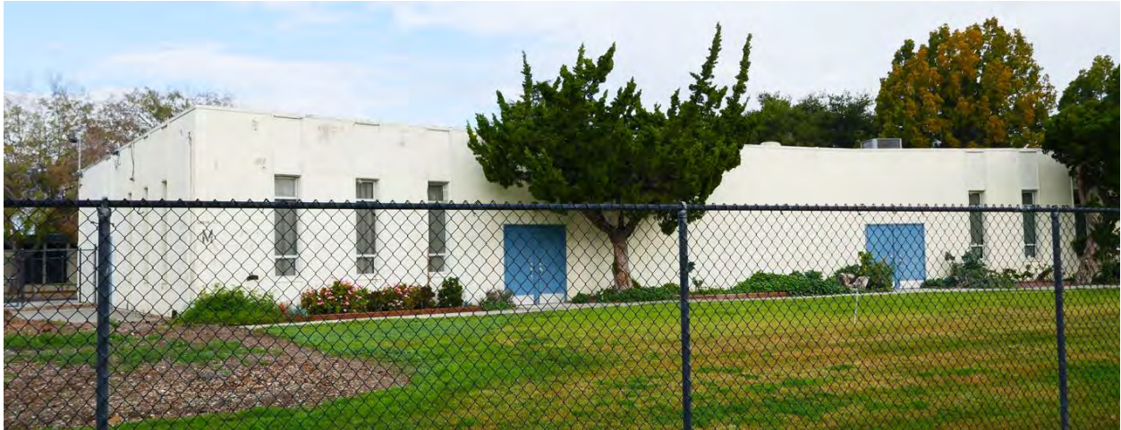
Figure 13. South façade of the administration building. Photograph taken 1/17/2022.
