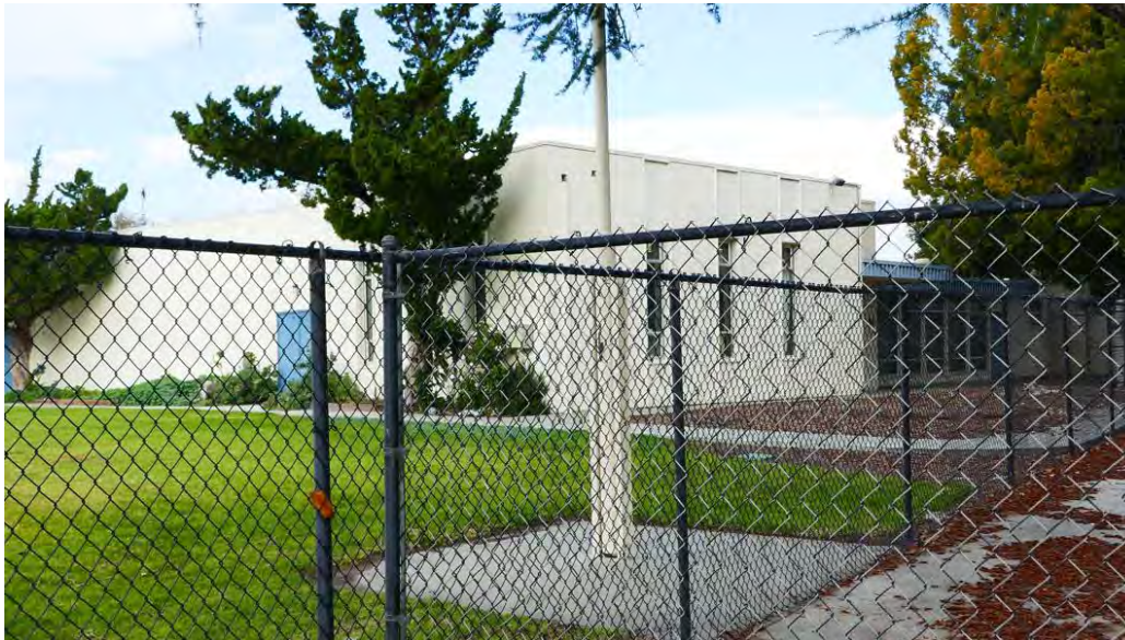
Figure 12. Southeast corner of the multipurpose building. Photograph taken 1/17/2022.
