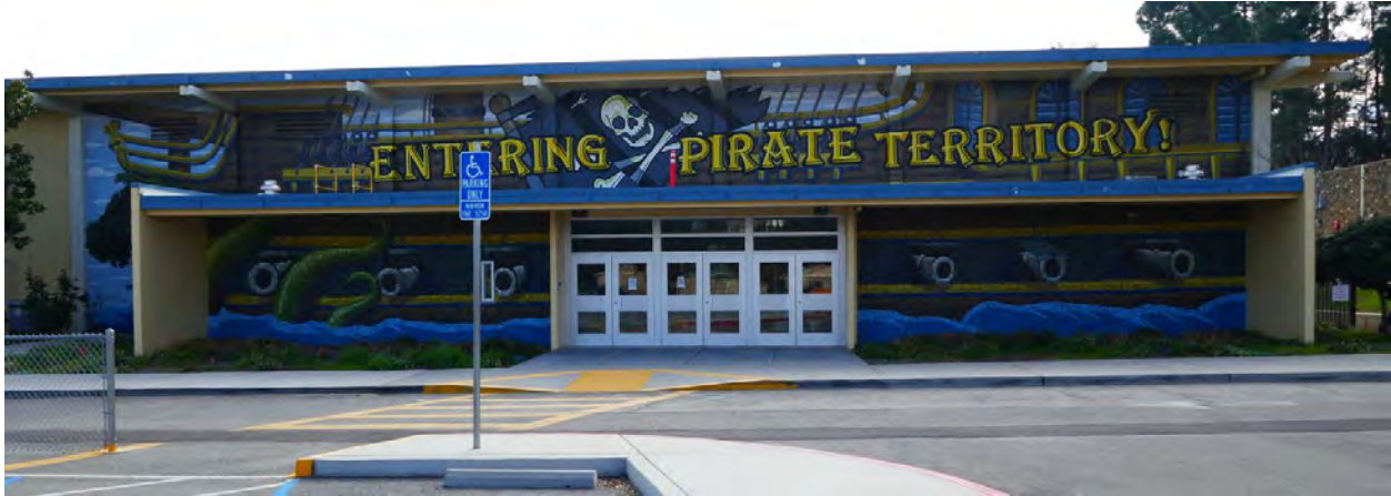
Figure 21. A portion of the north façade of the gymnasium showing the entrance. Photograph taken 1/17/2022.
