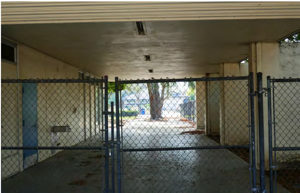
Figure 10. Walkway between the administration building (left) and multipurpose building. Photograph taken 1/17/2022.
