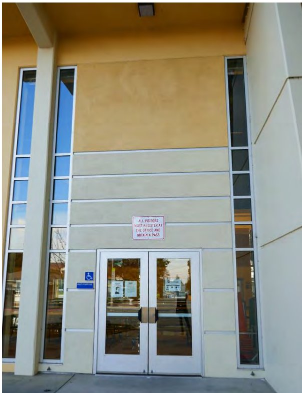
Figure 12. Detail of one of the entrances on the north elevation of the multipurpose building. Note the horizontal aluminum bands embedded in the wall and the scoring on the buttress. Photograph taken 1/17/2022.
