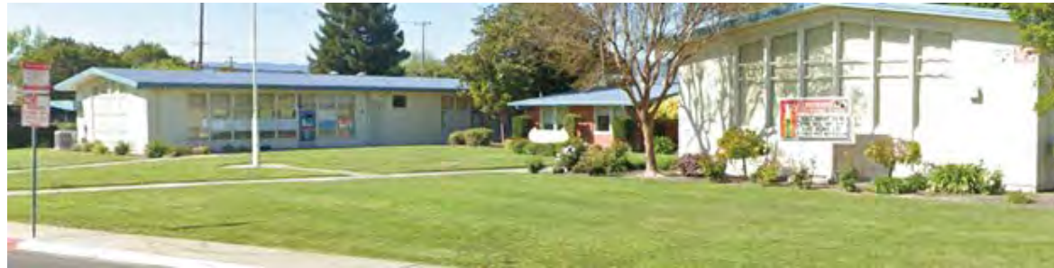
Constructed 1954-1956. Low gabled roofs, extended eaves, and generous expanses of fenestration are characteristic of Mid-Century Modern architecture. Likely designed by Clyde D. Goudie, Jefferson School District Architect
