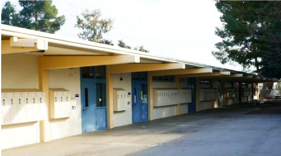
Figure 7. South elevation of classroom building B. Photograph taken 1/17/2022.
