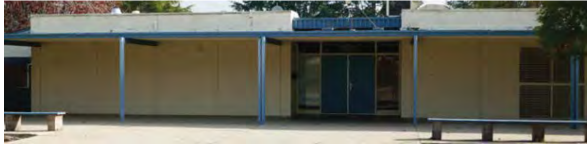
Photograph shows typical plain wall type, typical recessed entry with roof detail, and the covered walkway design.
