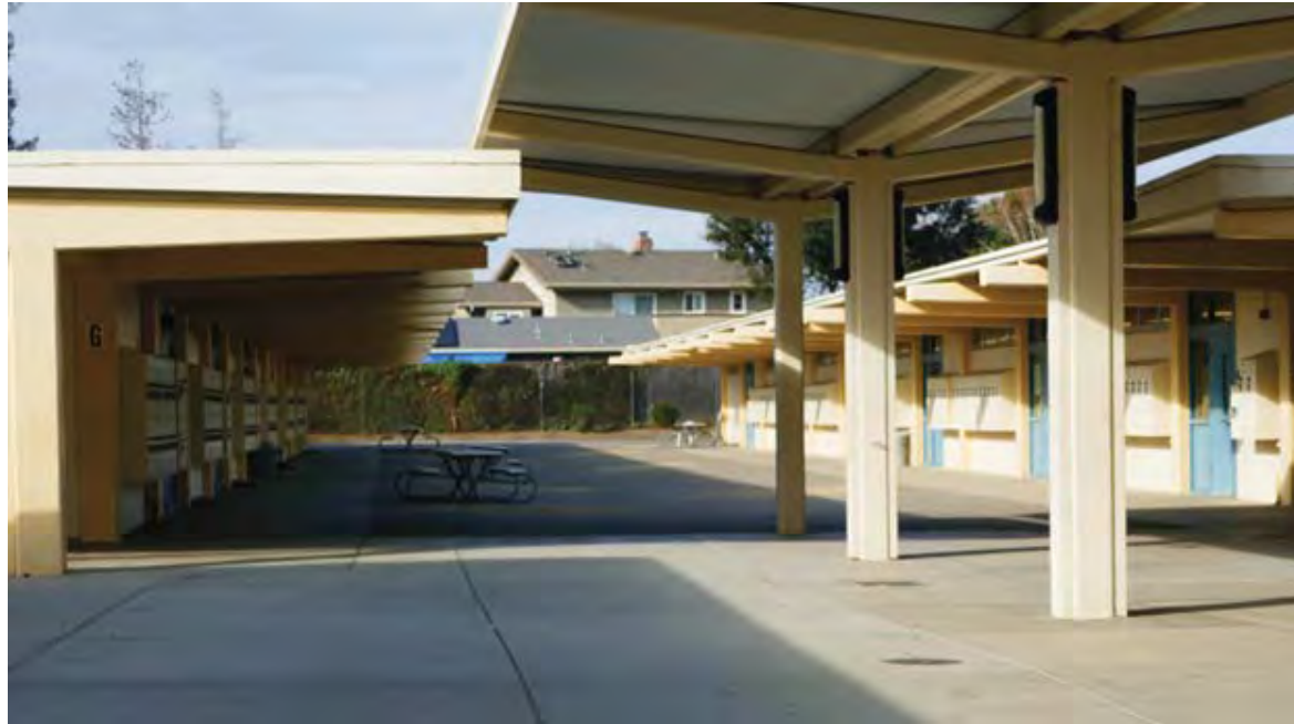
Camera facing west.
