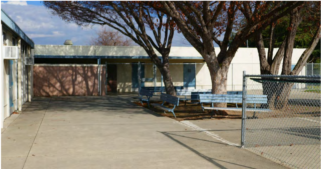
Figure 8. Northeast secondary courtyard. Building C. Camera facing north. Photograph taken 1/17/2022.
