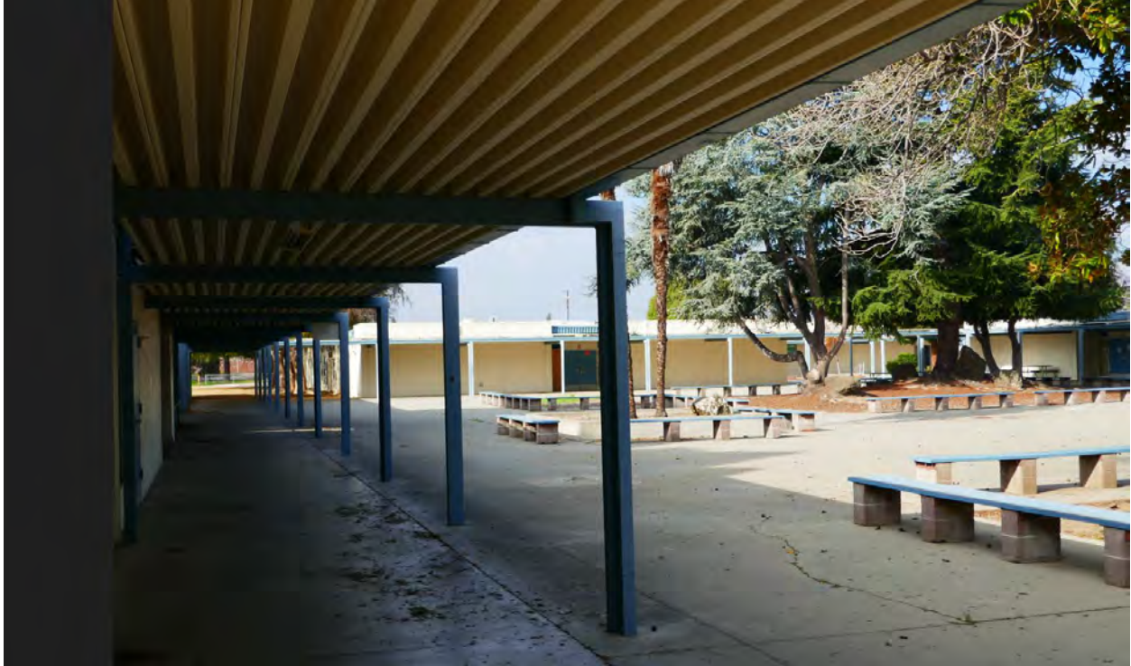
Figure 5. Central courtyard and covered walkway. Camera facing west. Photograph taken 1/17/2022.
