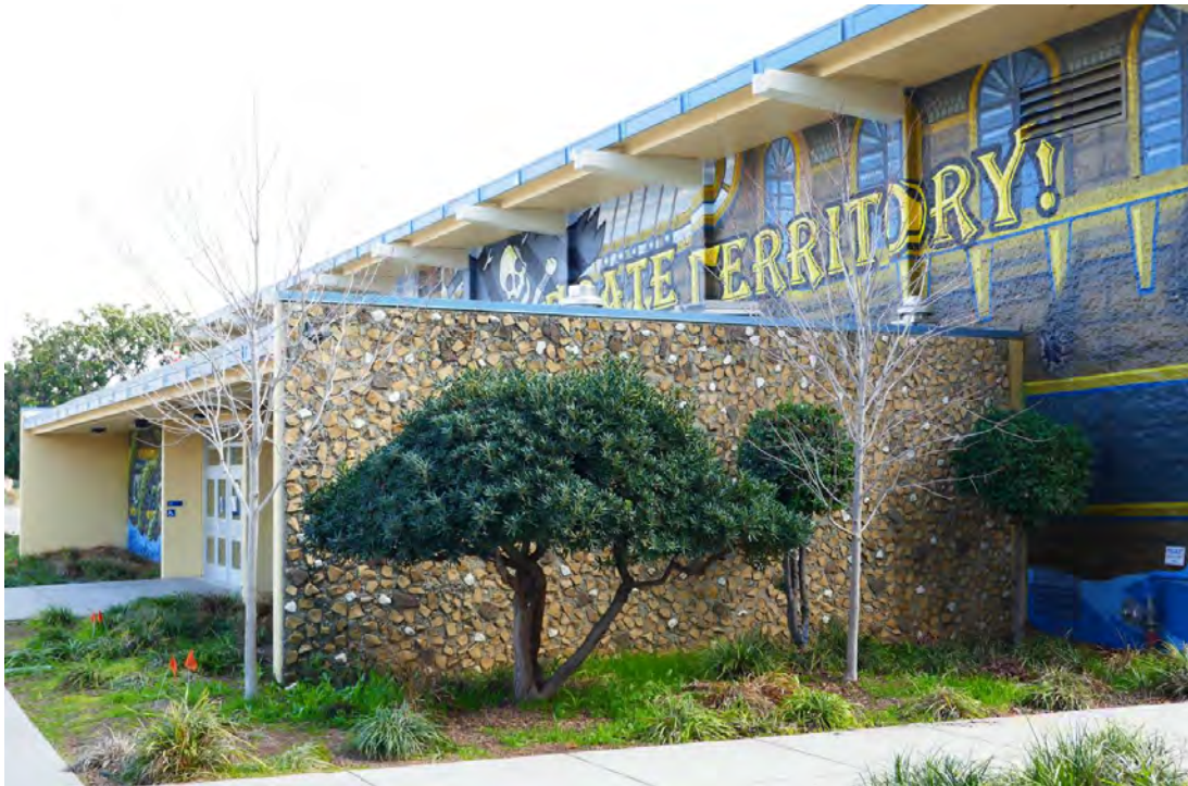
Figure 22. The northern entrance. Camera facing southeast. Photograph taken 1/17/2022.
