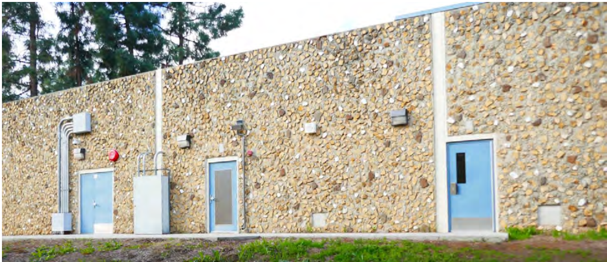
Figure 16. East elevation of the multipurpose building. Photograph taken 1/17/2022.
