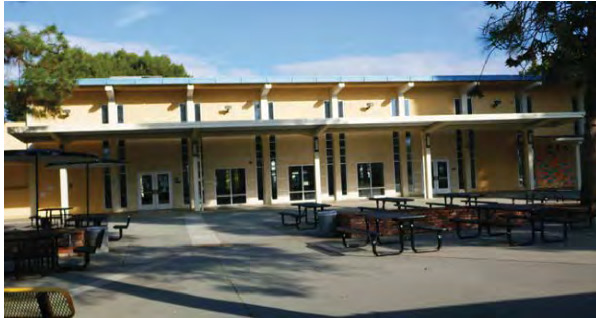
The central portion is sheltered by a free-standing butterfly canopy.
