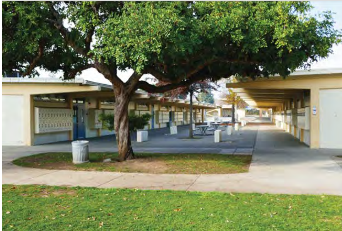
Camera facing west.
