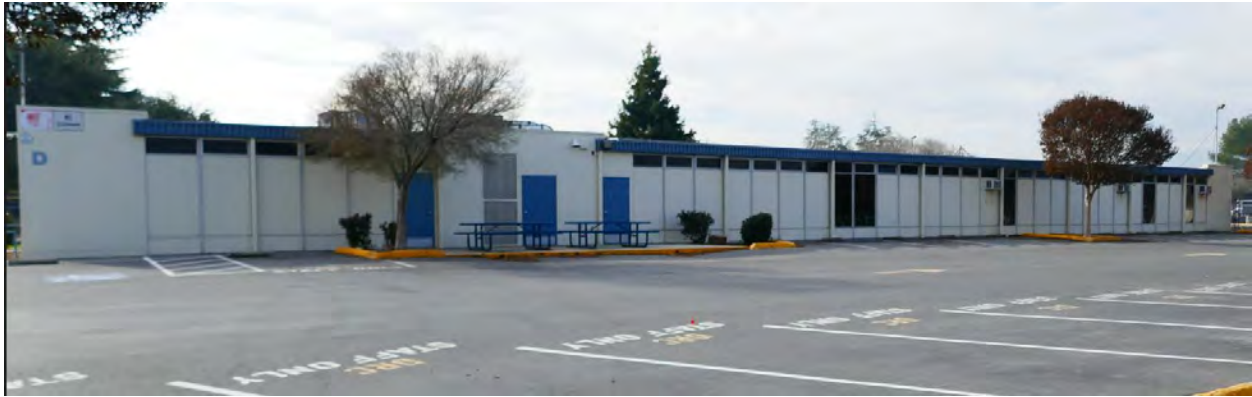
Figure 9. North elevation of classroom building D. Photograph taken 1/17/2022.
