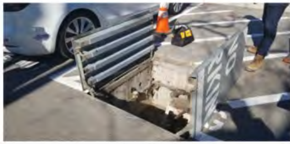
Intersil Extraction Well 12A
