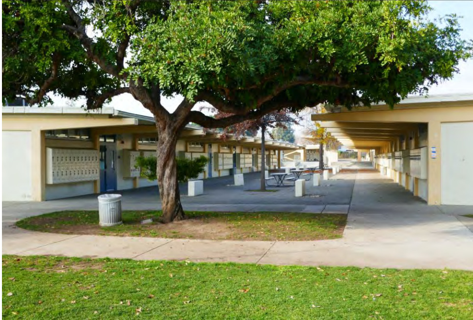
Figure 3. Outdoor space between classrooms A and B. Camera facing west. Photograph taken 1/17/2022.
