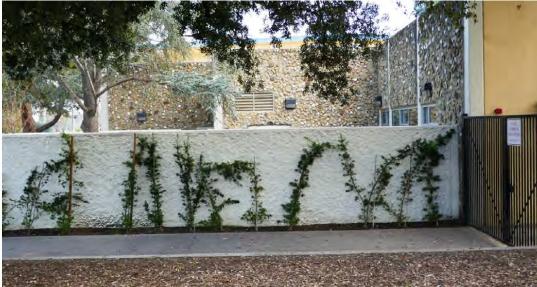
Figure 15. West elevation of the multipurpose building. Photograph taken 1/17/2022.
