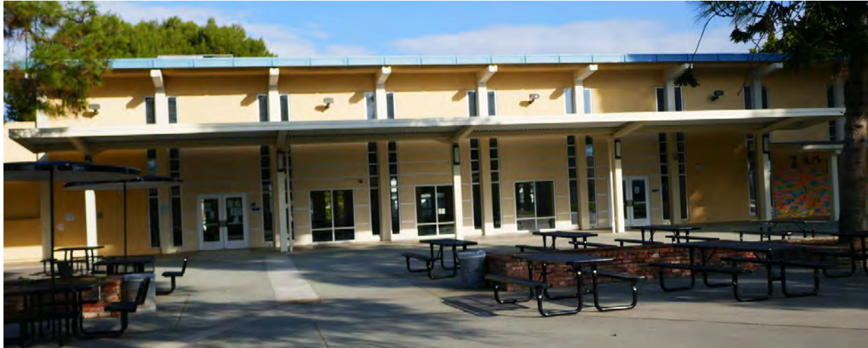
Figure 17. South elevation of the multipurpose building. The central portion is sheltered by a free-standing butterfly canopy. Photograph taken 1/17/2022.
