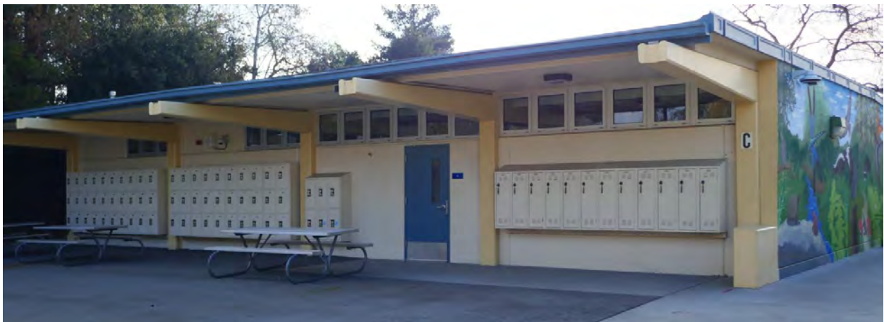
Figure 8. East elevation of classroom building C. Photograph taken 1/17/2022.
