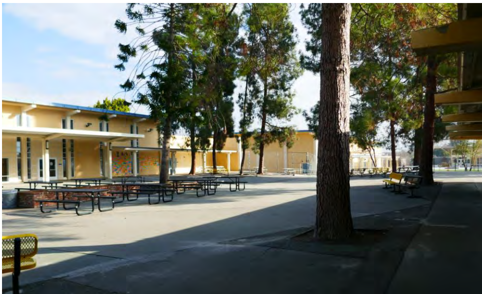
Figure 4. Open area between classroom building A and the multipurpose building. Camera facing northeast. Photograph taken 1/17/2022.
