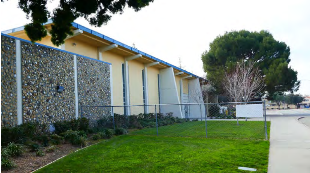
Figure 13. North façade of the multipurpose building. Photograph shows the scale of the buttresses and the exaggeration of the height of the building from the engaged columns and buttresses. The façade of the east elevation can also be seen on the left. Camera facing west. Photograph taken 1/17/2022.
