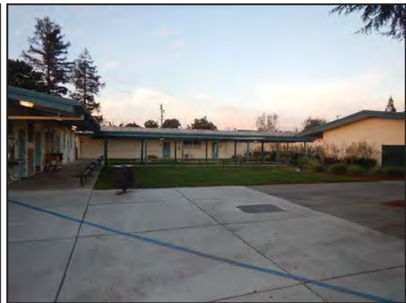
Photograph 6. Laurelwood Elementary overview, facing north.
