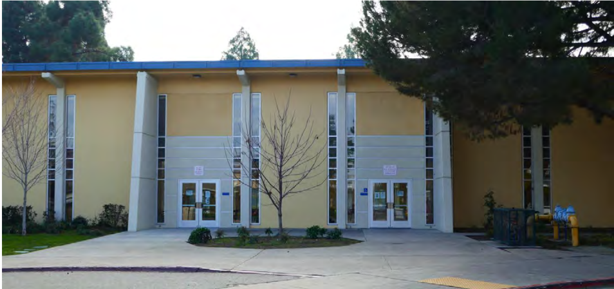
Figure 11. North entrance to the multipurpose building. Photograph taken 1/17/2022.
