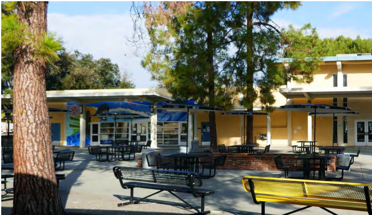
Figure 18. South façade of the west wing of the multipurpose building. Photograph taken 1/17/2022.
