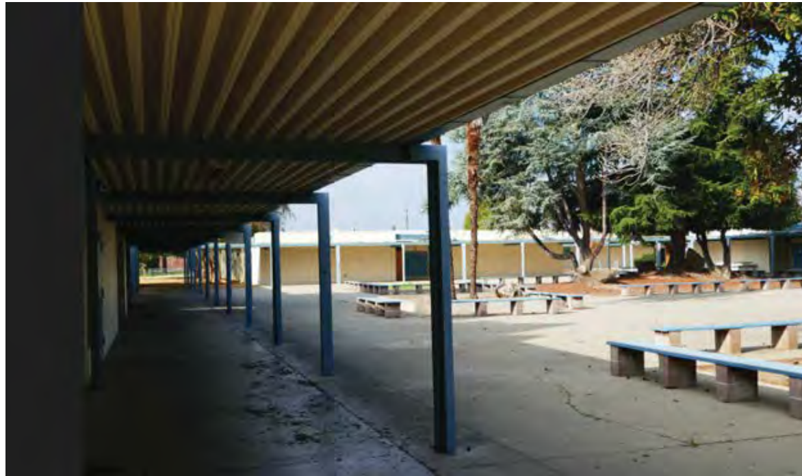
Camera facing west.
