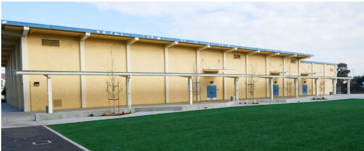
Figure 24. Southern façade of the gymnasium and additions. Camera facing northeast. Photograph taken 1/17/2022.
