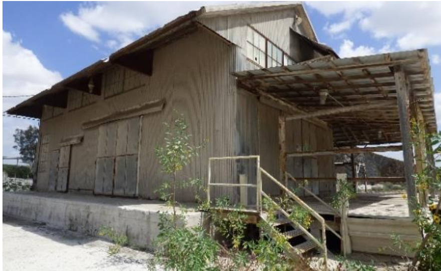
Figure 46: West and south elevations, view northeast.
