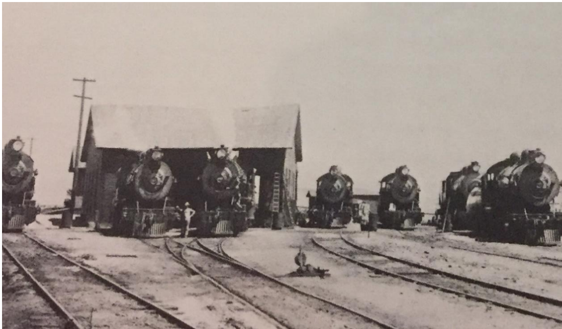
Riverside-Crestmore Cement Plant / D170213.00
