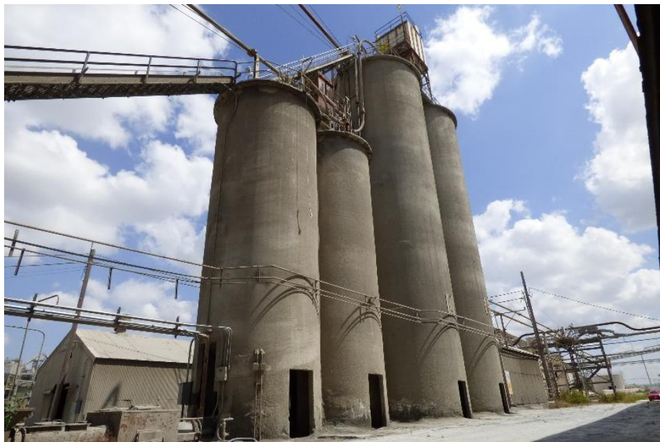
Figure 54: View of the silos near packing area, view southeast.
