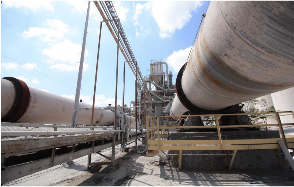
Figure 31: View of the north elevation, view south.
