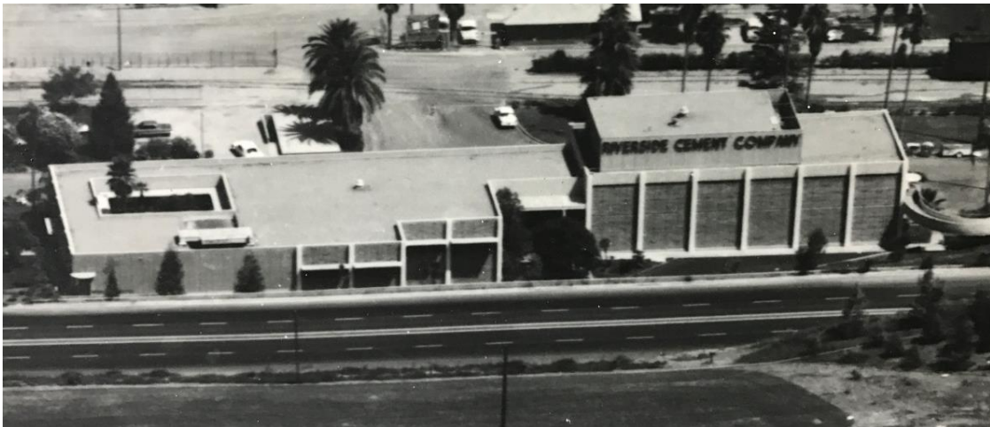
Riverside-Crestmore Cement Plant / D170213.00
