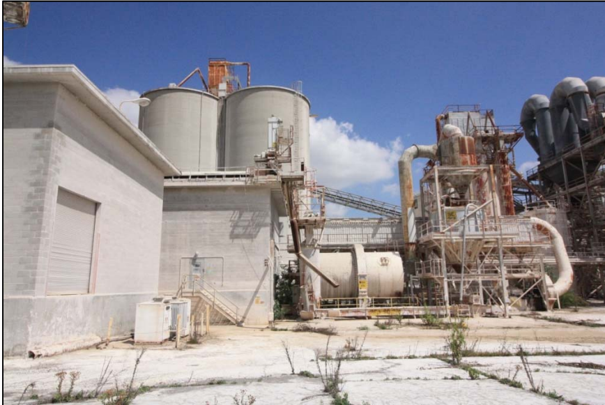
View of the east side and south elevations (view northwest) (ESA, 2017)
