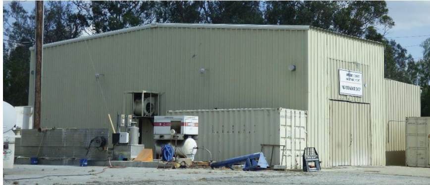
Figure 44: View of the Maintenance Shop, view south.
