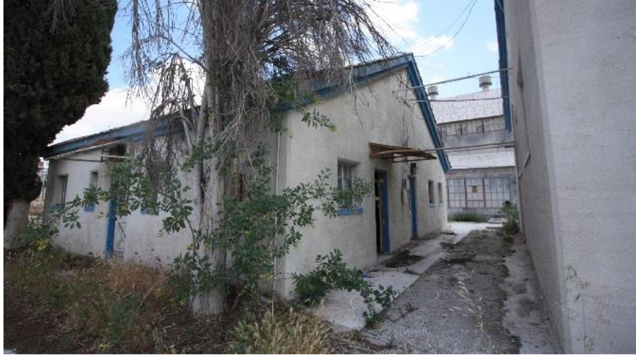
Figure 37: View of the south and west elevations, view northeast.
