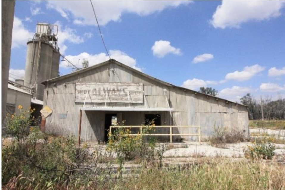
Riverside-Crestmore Cement Plant / D170213.00
