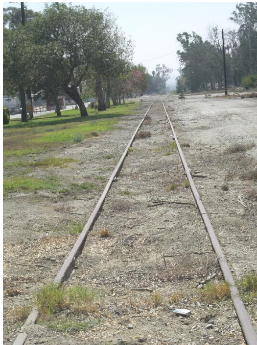
Photo 14: Study Area, P-33-013240 Railroad Spur, view towards the south.
