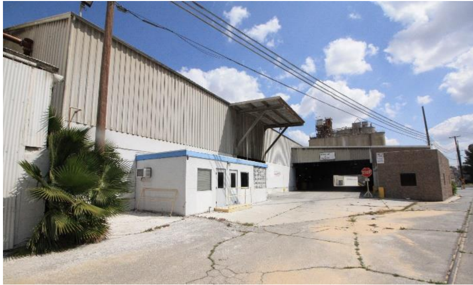
Figure 51: View of the northern portion of the west elevation, view southeast.
