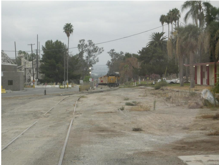
Photo 15: Study Area P-33-013240 Railroad Spur, view towards the south.
