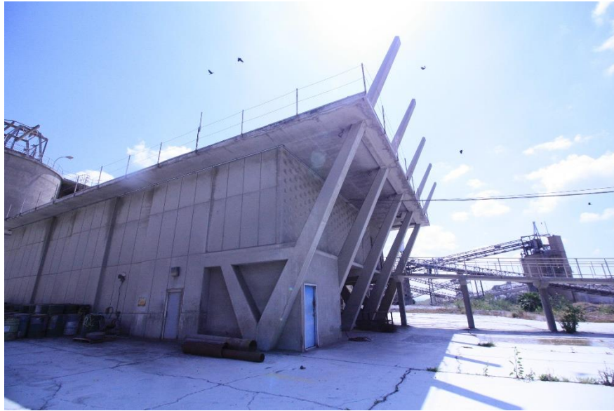
Figure 28: Gray Cement Mill Control Center, view south.
