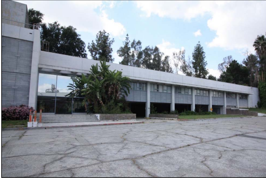
View of the building's primary (east) elevation, north end (view west) (ESA, 2017)
