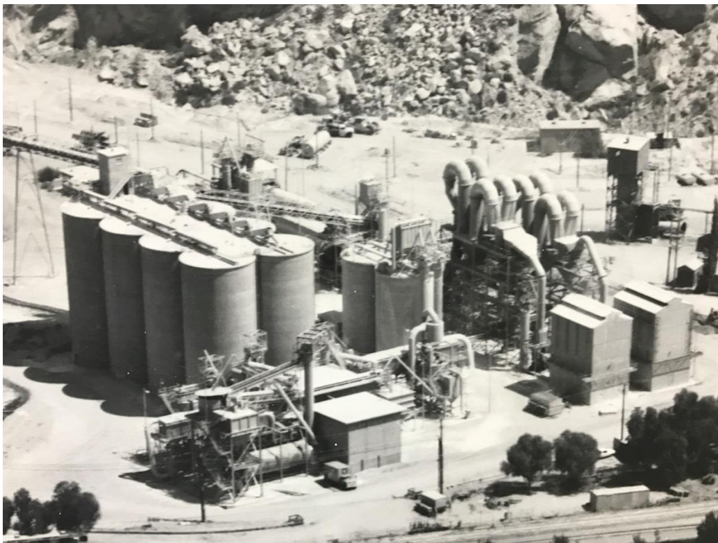
Riverside-Crestmore Cement Plant / D170213.00
