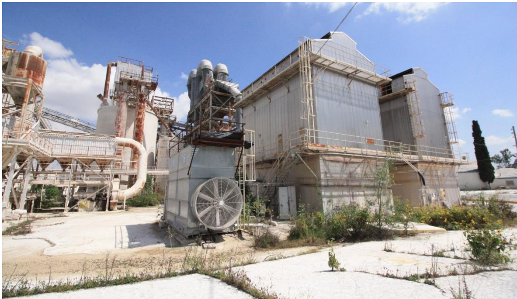
Figure 32: View of the north elevation, view south.
