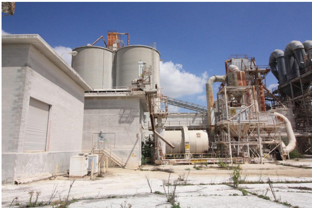
Figure 30: View of the east side and south elevations, view northwest.
