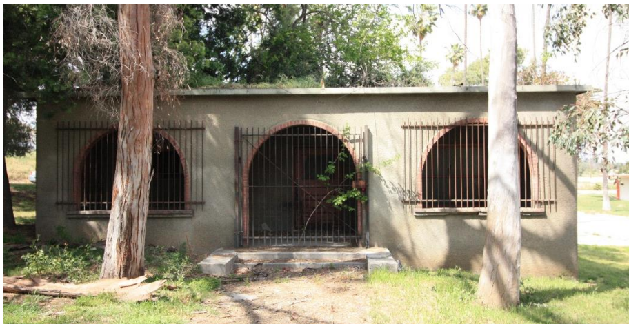
Figure 41: View of the building's primary (south) elevation (view north).
