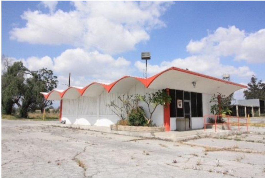
Figure 53: View of the south and west elevations, view northeast.
