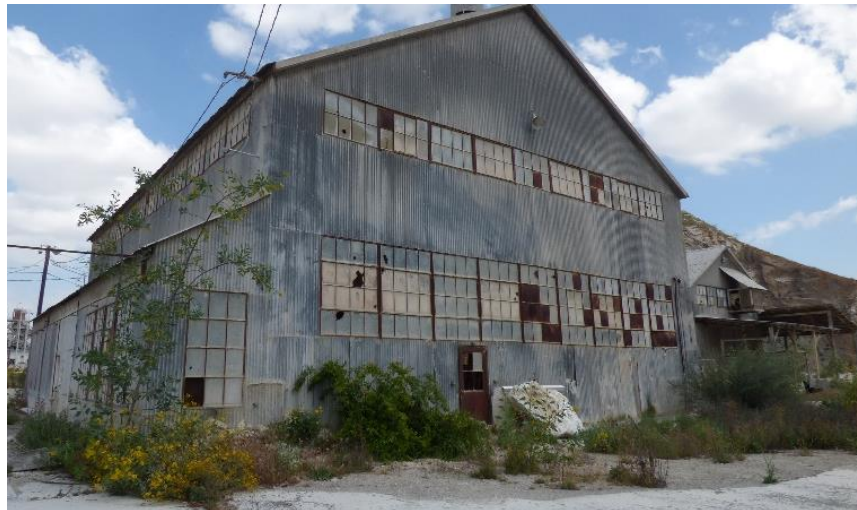
Figure 45: View of the north and west elevations, view northeast.
