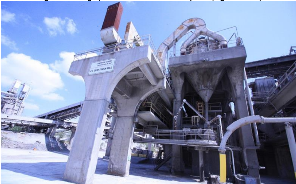
Figure 25: Gray Cement Mill, view of the west elevation, view northeast.
