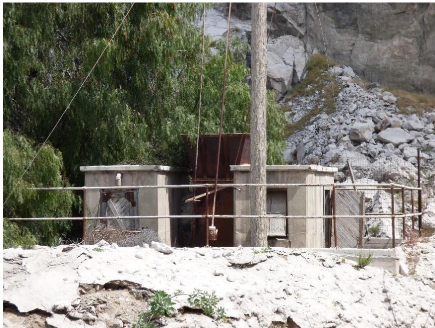
Figure 57: Northeast view of mine vents.
