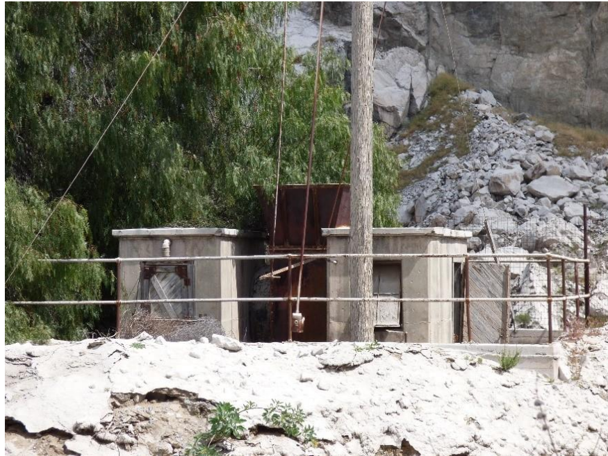
Riverside-Crestmore Cement Plant / D170213.00
