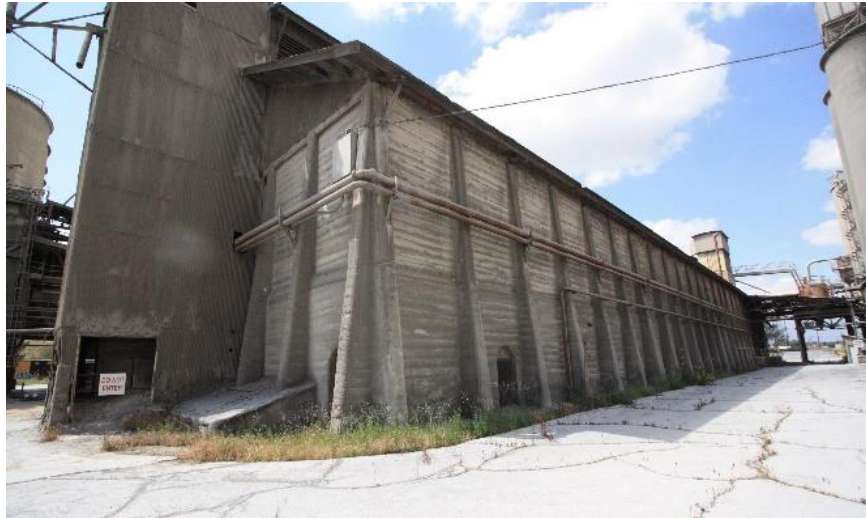
Figure 49: View of the east side and south elevations, view northwest.
