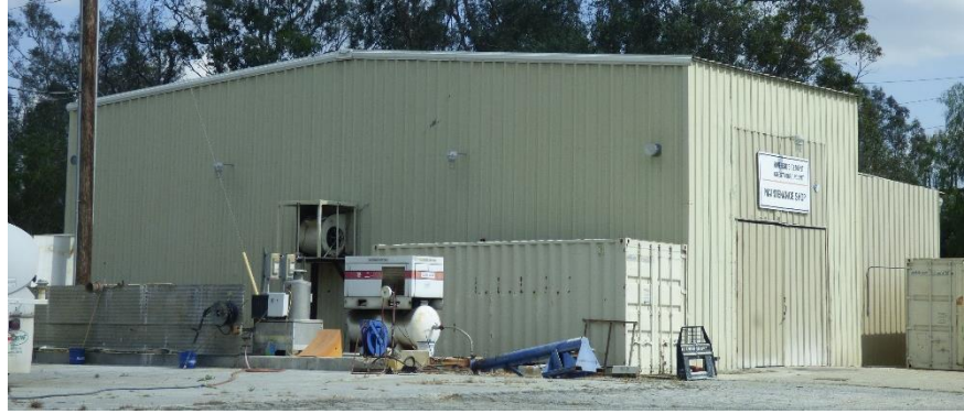
Riverside-Crestmore Cement Plant / D170213.00
