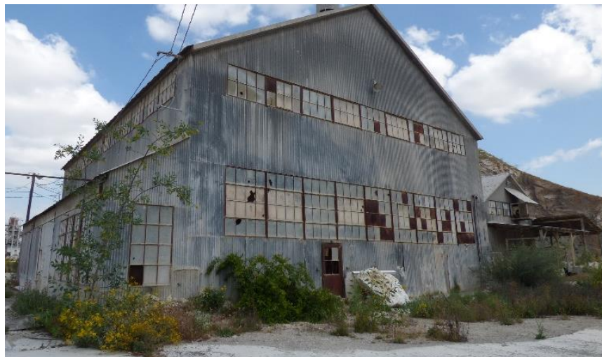
Riverside-Crestmore Cement Plant / D170213.00
