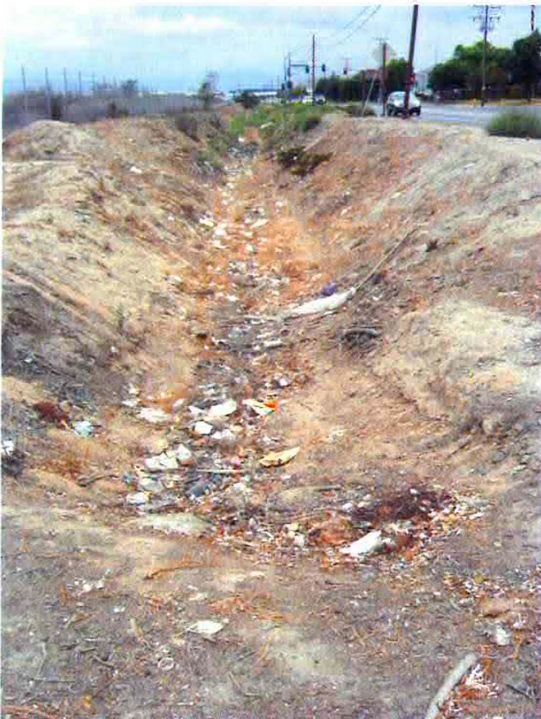
P-33-005044H, Along Auga Mansa Road, view towards the west
