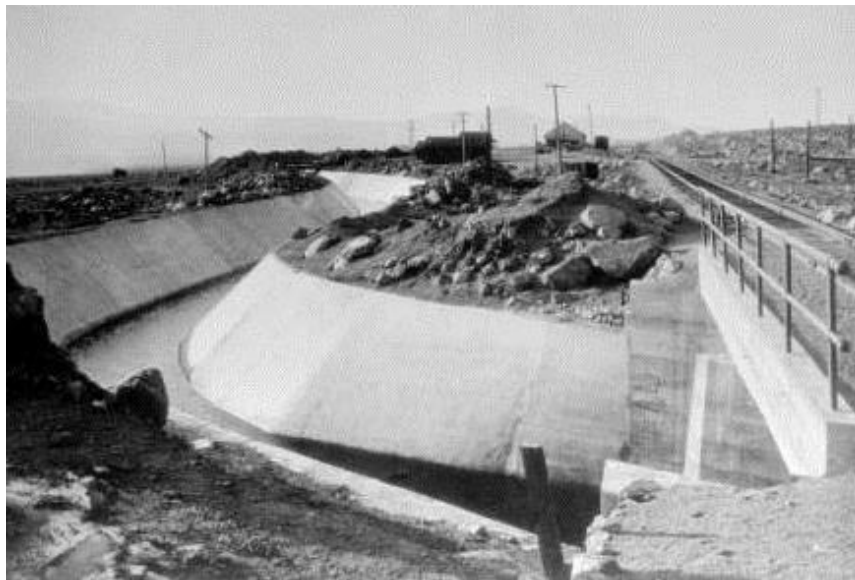
Riverside-Crestmore Cement Plant / D170213.00
