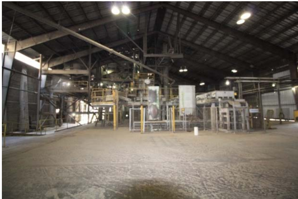
View of the northern portion of the west elevation (view southeast)
