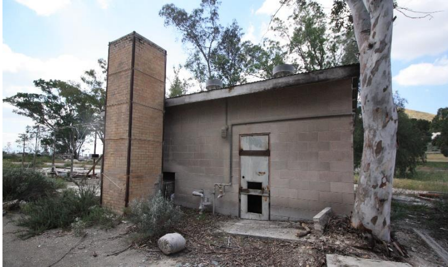
Figure 39: View of the east elevation, view west.
