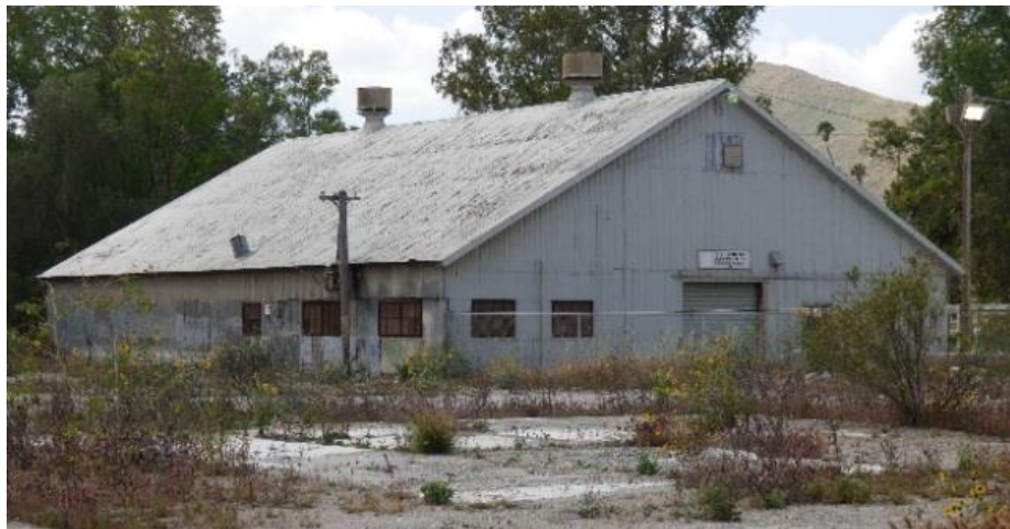
Figure 38: View of the north and east elevations, view southwest.
