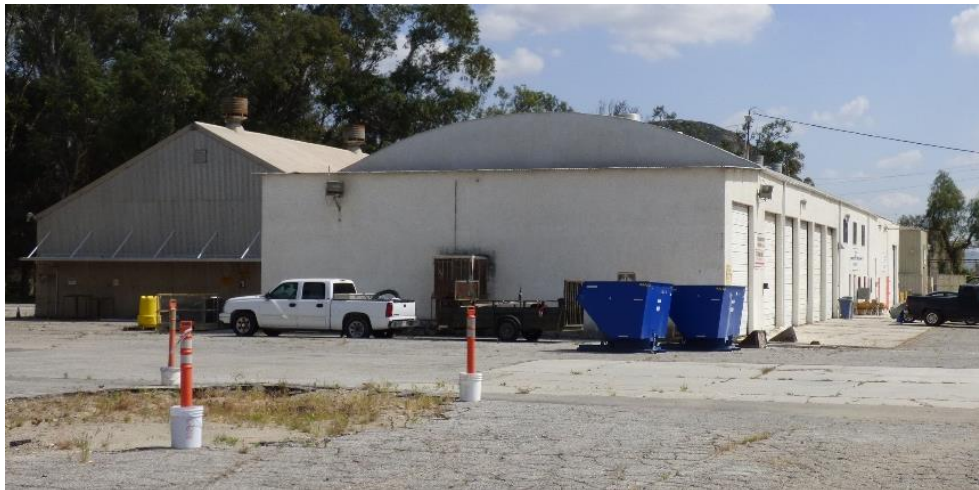
Figure 43: View of the Operation's Office and Tire Shop, view southwest.
