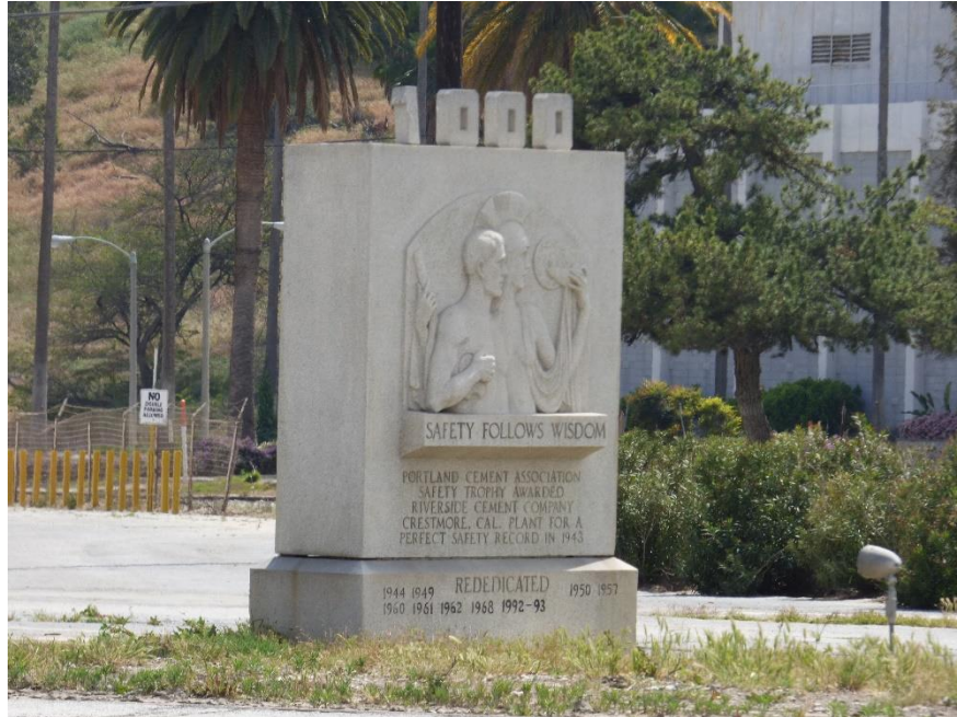
Riverside-Crestmore Cement Plant / D170213.00
