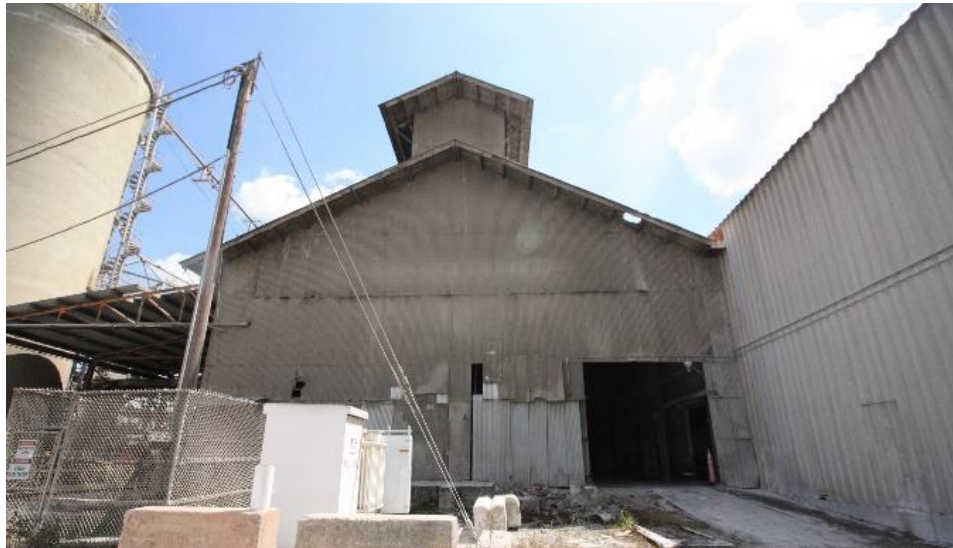
Figure 50: View of the north elevation, view south.
