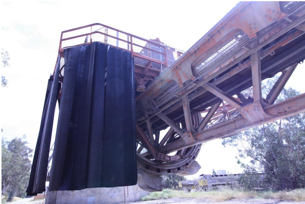
Figure 26: Reclaimer near the northeast corner of the Plant, view southeast.
