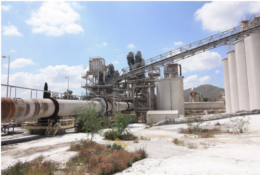
Figure 29: View of the south elevation, view northwest.
