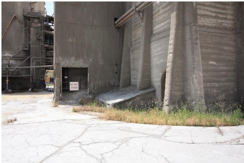
Figure 48: View of the south elevation, view northwest.
