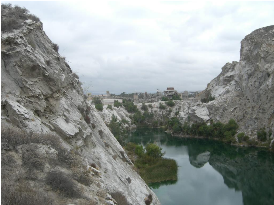
Photo 17: Study Area, view of previous quarry area.
