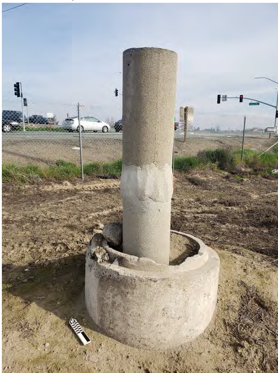
Photograph 3 Concrete Pipe and Base 1; View Northeast
