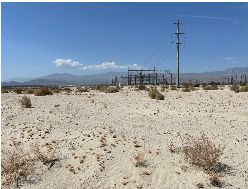
Photograph 5. Project Area north of the Ramon Substation, facing south.
