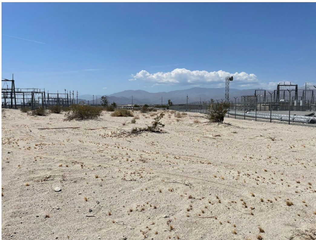
Photograph 1. Project Area west of the Ramon Substation, facing south.
