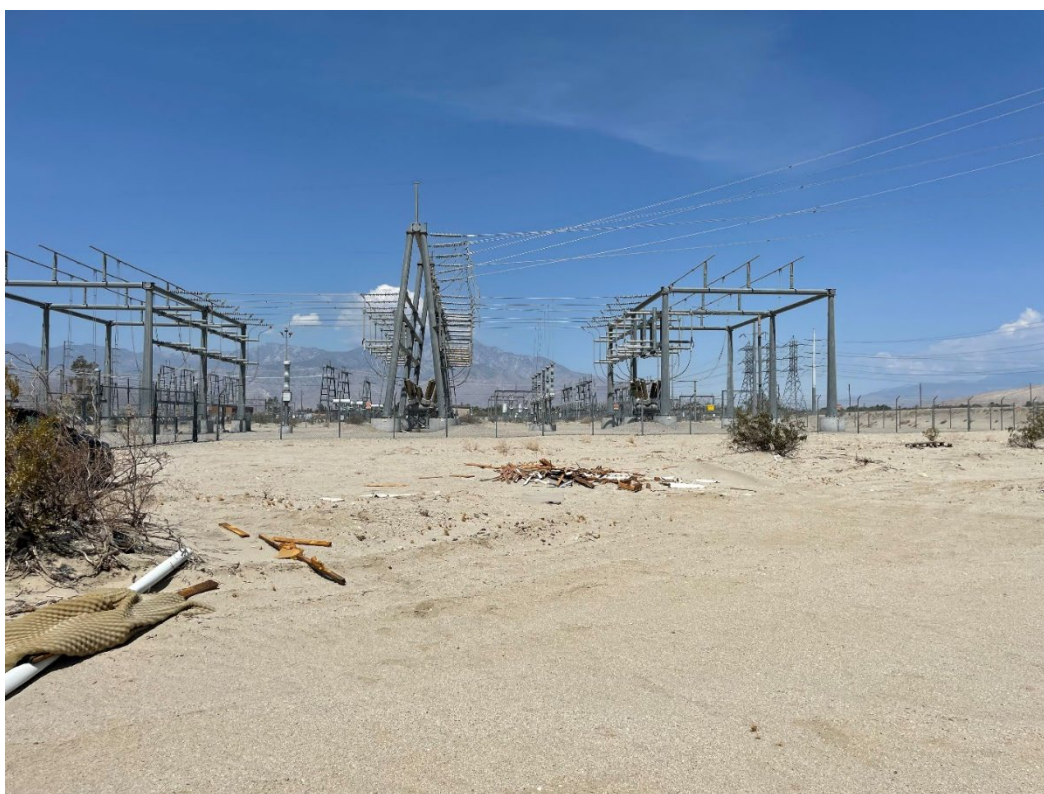
Photograph 4. Project Area east of the Ramon Substation, facing west.
