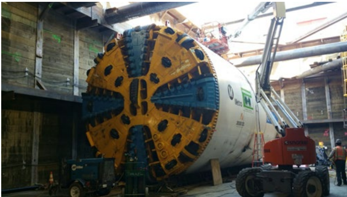
Figure 2: Tunnel Boring Machine
