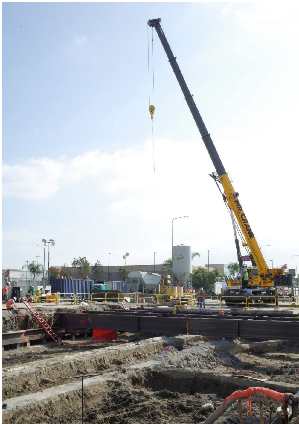
Figure 1: Example of Construction via Cut-and-Cover
