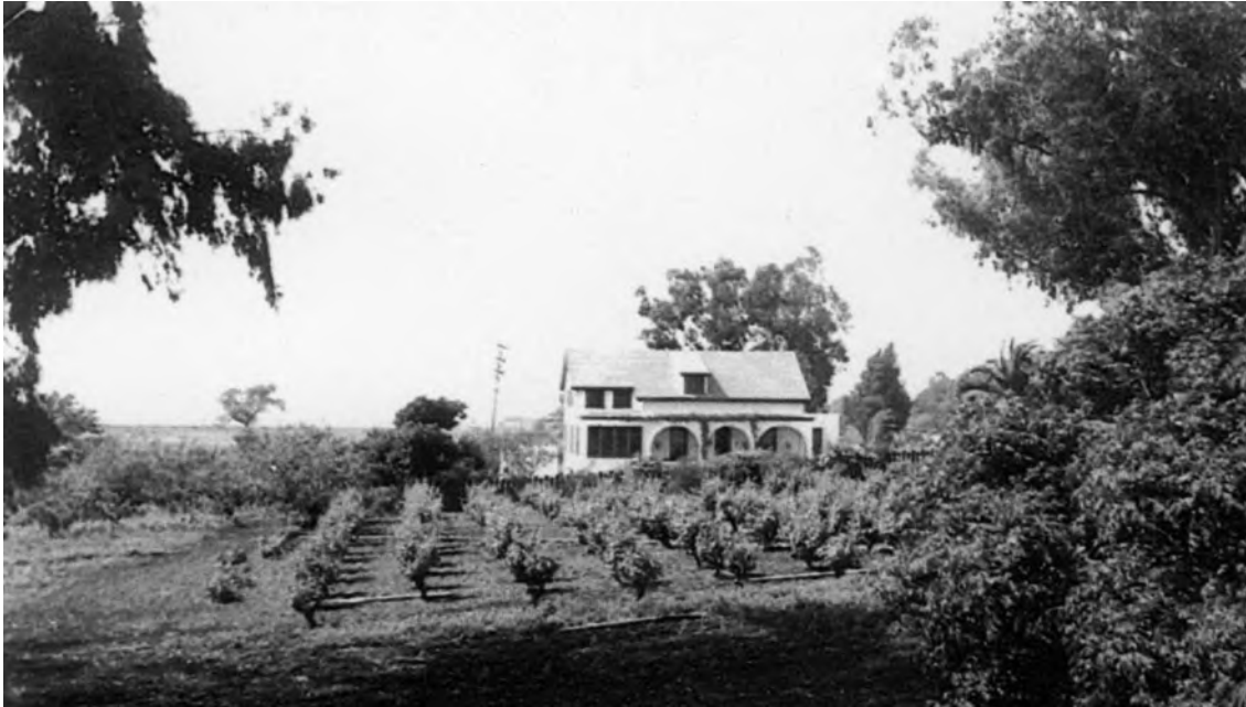
Figure 2. Undated photograph of the Ellerhorst Home after its Spanish Colonial Revival-style remodel in the early twentieth century (Vincent 2019:10)
