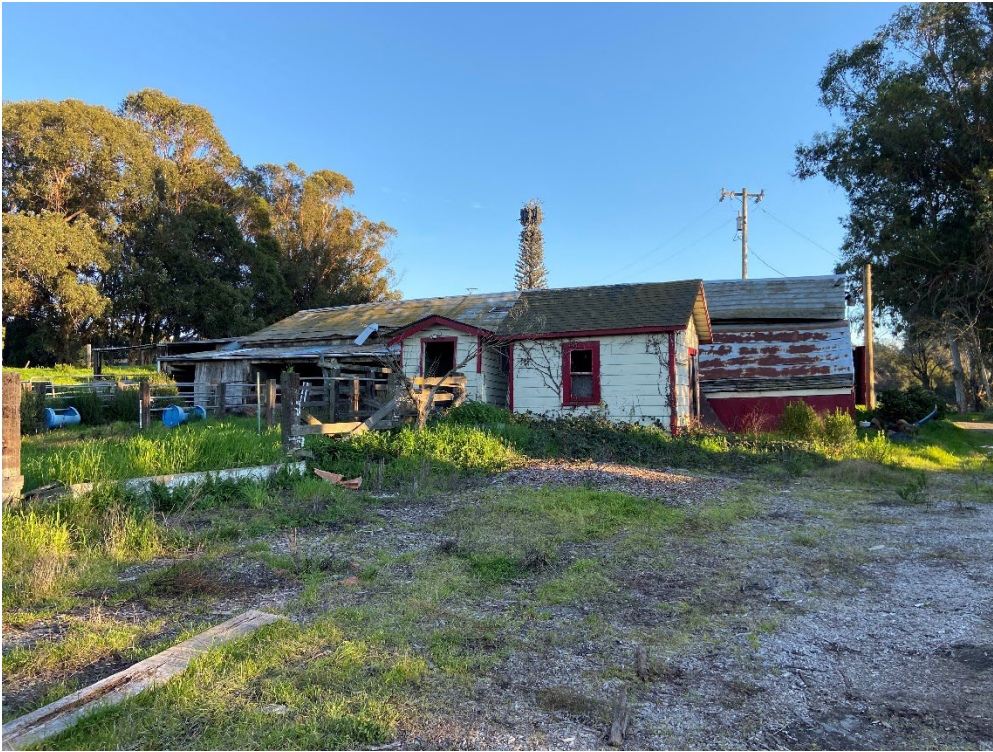
Photograph 39: A photograph of stables in the central portion of the project site
