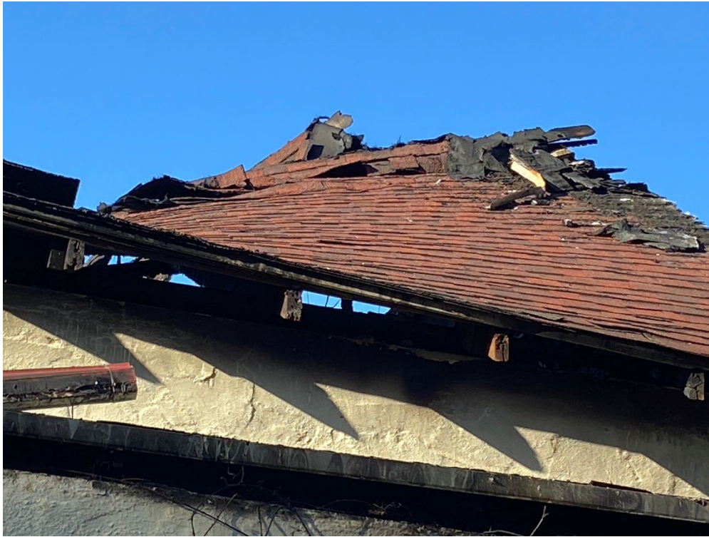
Photograph 23: A photograph of the roofing for the above house.
