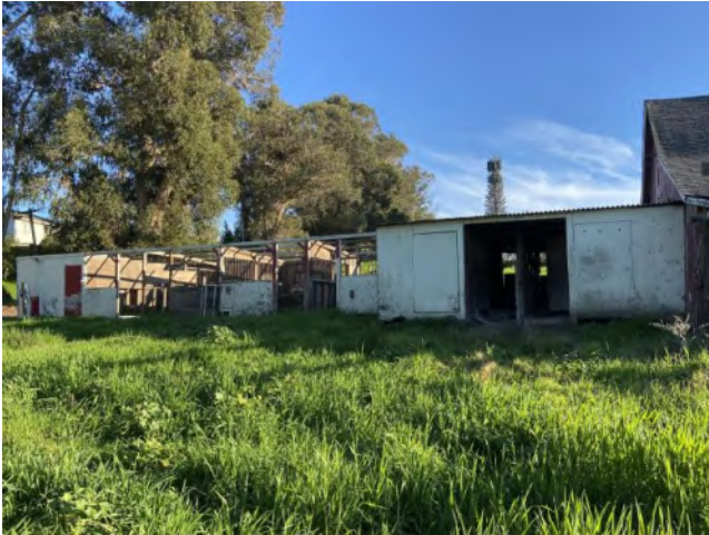
North elevation, view south
