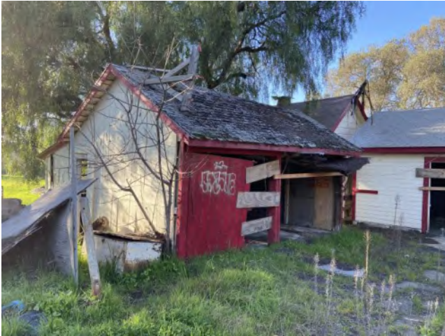
South (left) and east (right) elevations, view northwest
