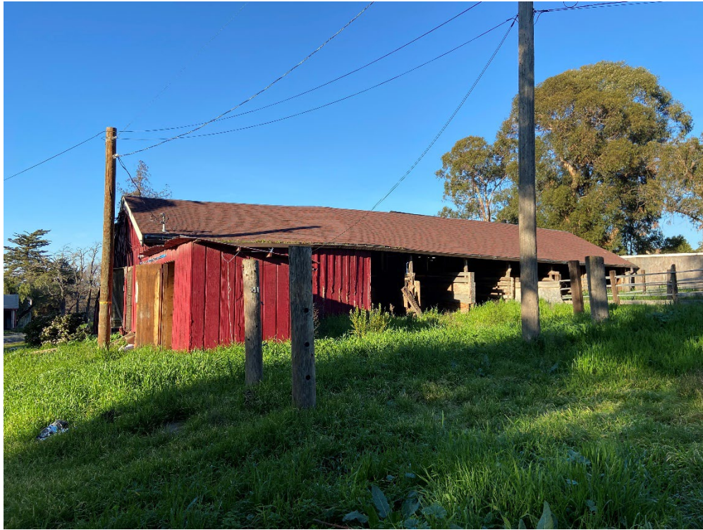
Photograph 33: A photograph of stables in the central portion of the project site.
