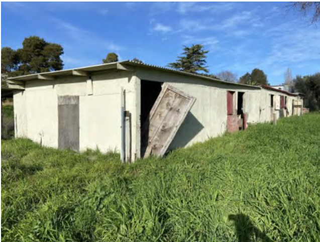
West (left) and south (right) elevations, view northeast
