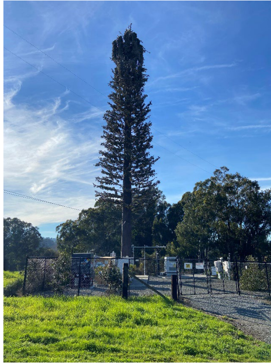
Photograph 1: Cellphone tower located in southeast corner of the project site.
