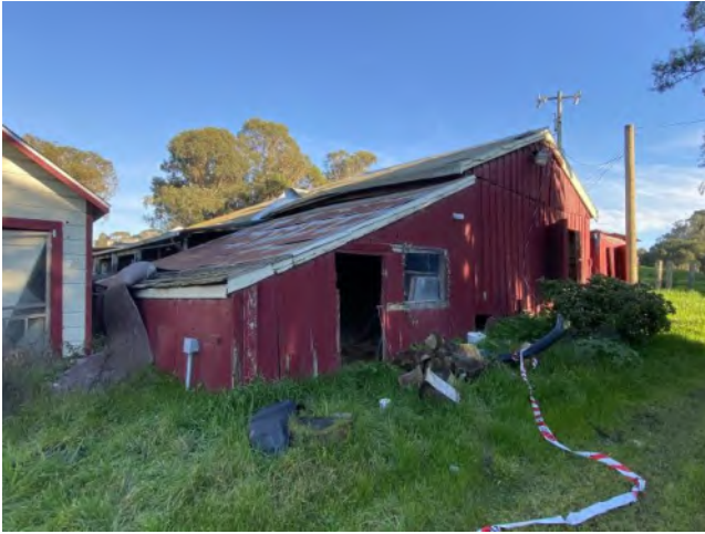
North (left) and west (right) elevations, view southeast
