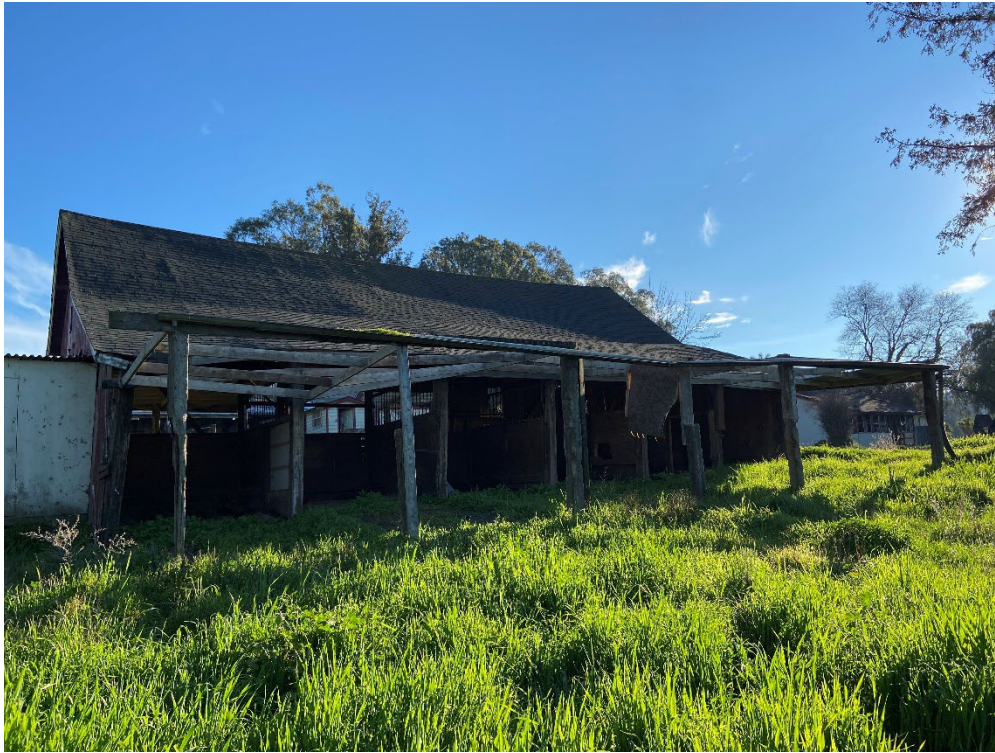
Photograph 27: A series of stables in the eastern portion of the project site.
