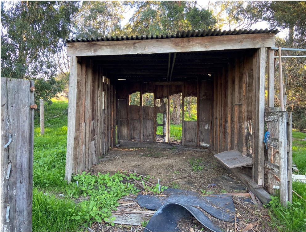
Photograph 35: A photograph of stables in the central portion of the project site.
