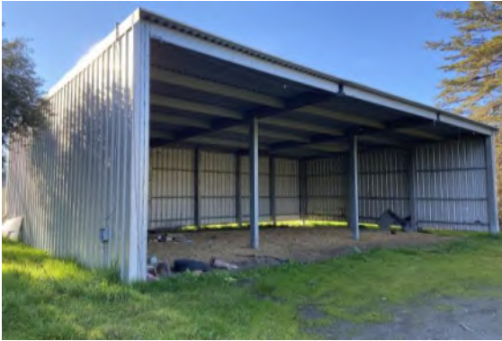
South (left) and east (right) elevations, view northwest.
