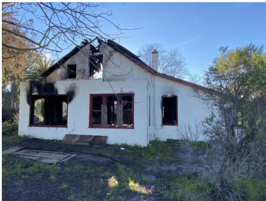
Photograph 3. East elevation; facing west.
