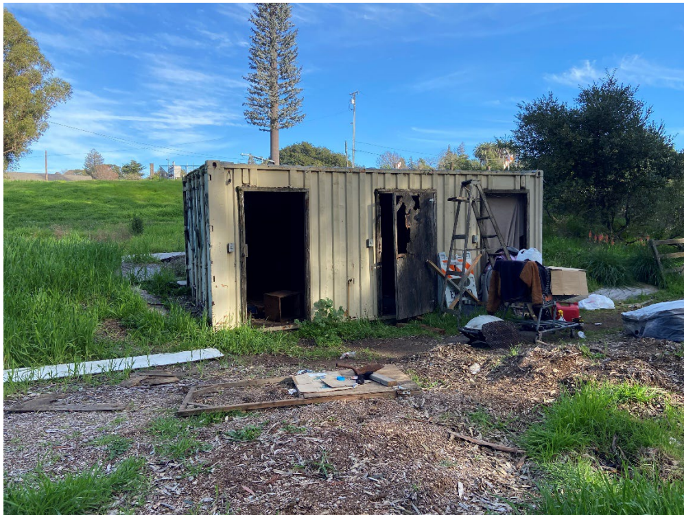
Photograph 10: Shipping container located in the central portion of the project site.
