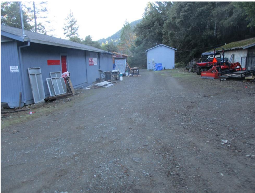
Palomino Estates water treatment and storage site. The existing water storage tank is on the right.
