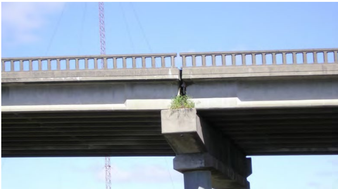
Photo 3. Petaluma River Bridge Existing Concrete Baluster Railing
