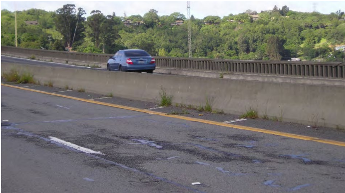
Photo 1. Petaluma River Bridge Existing Pavement Condition
