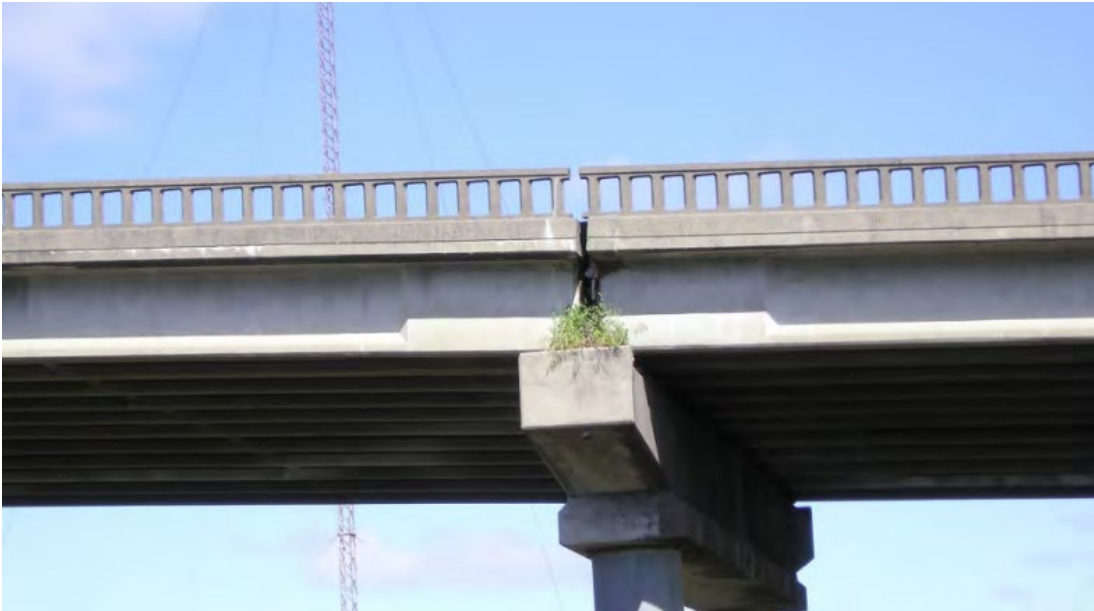
Photo 3. Petaluma River Bridge Existing Concrete Baluster Railing
