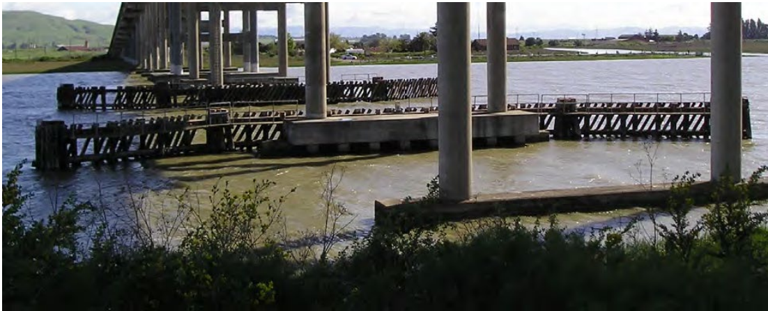
Photo 2. Petaluma River Bridge Timber Fender System (looking east)
