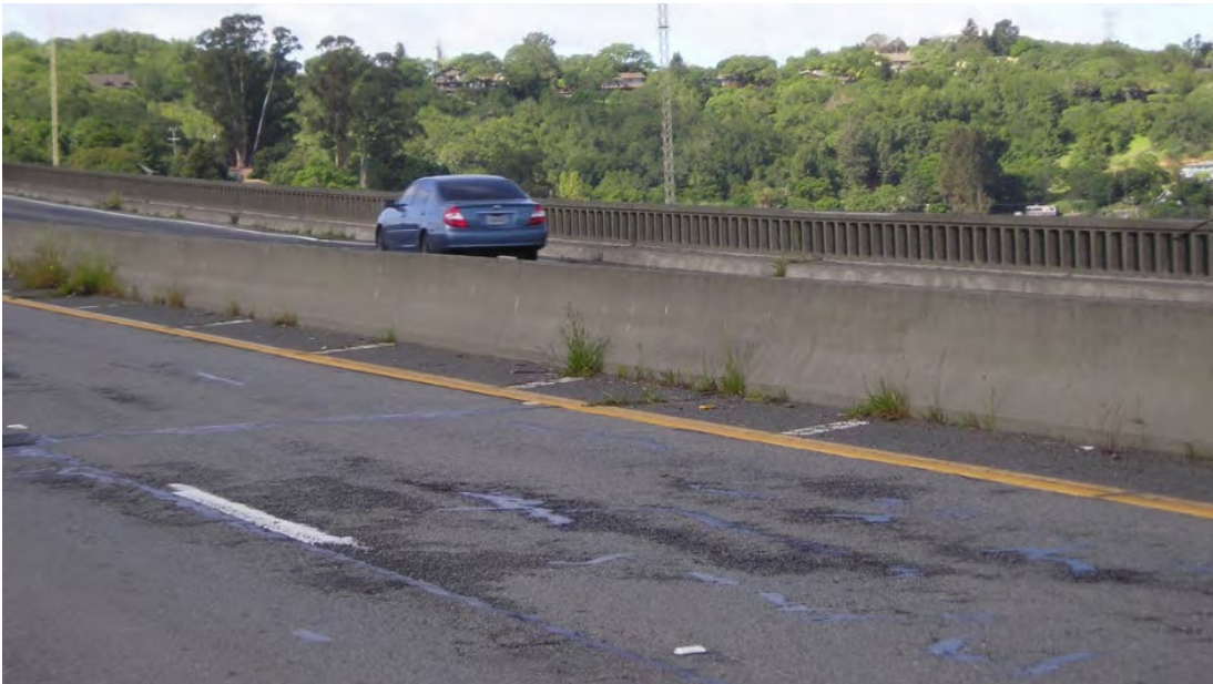
Photo 1. Petaluma River Bridge Existing Pavement Condition
