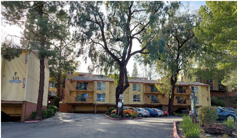
Photograph 3. Photograph of multi-family units from intersection of Chilpancingo Parkway and Old Quarry Road looking north
