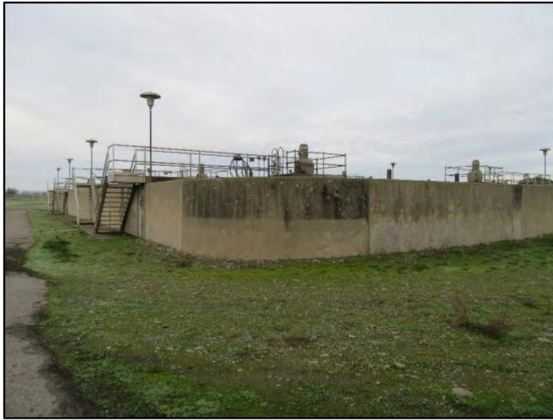
Figure 3-5. West view of Resource OW-001 - 1970s aeration basin located on plant
