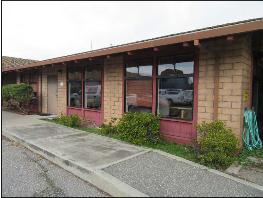
Figure 9. OW-001, 1970s main office located at the plant (view northwest) January 23, 2020.
