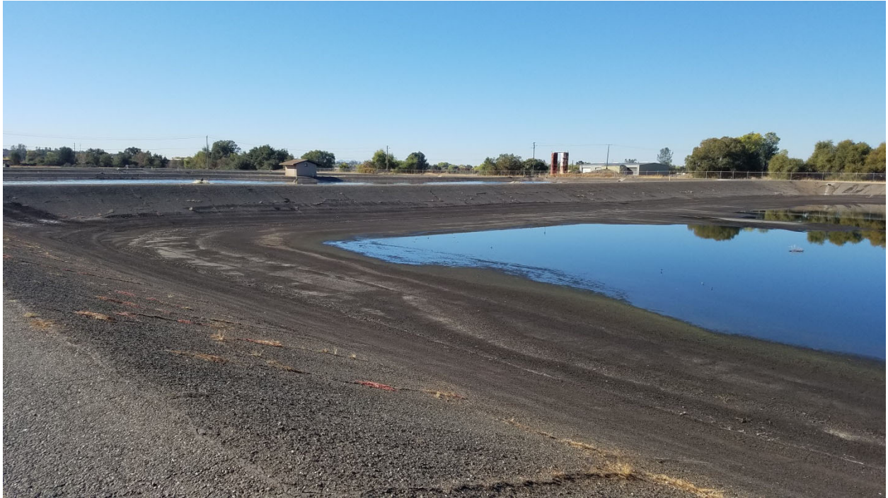
Picture 3: Developed WWTP habitat (sewage treatment lagoons).
