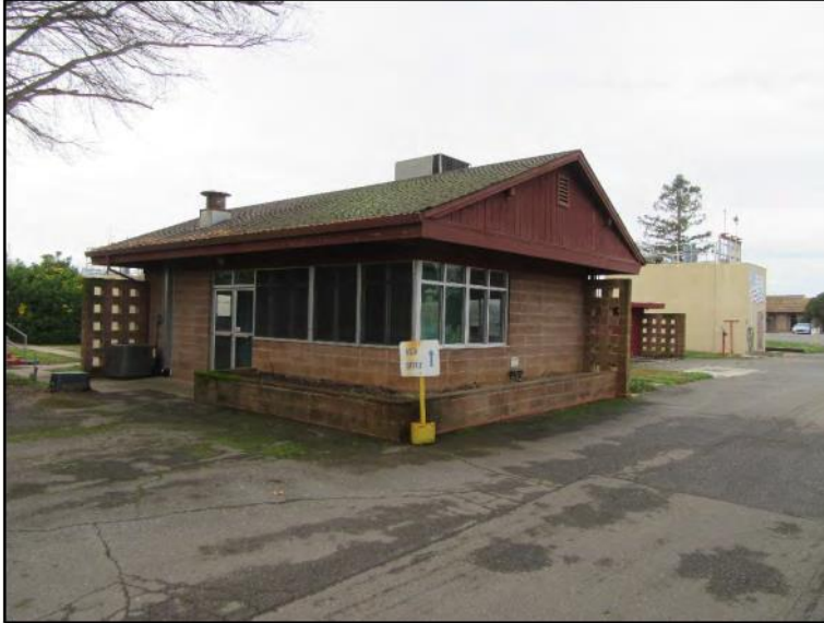
Figure 3-3. Southwest view of Resource OW-001 - 1950's building located at the plant
