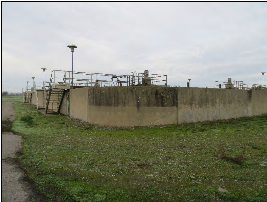
Figure 8. OW-001, 1970s aeration basin located at the plant (view west) January 23, 2020.
