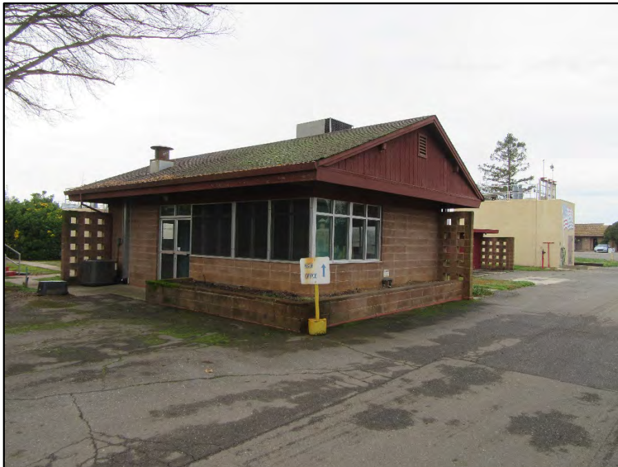
Figure 6. OW-001. 1950s building located at the plant (view southwest) January 23, 2020.
