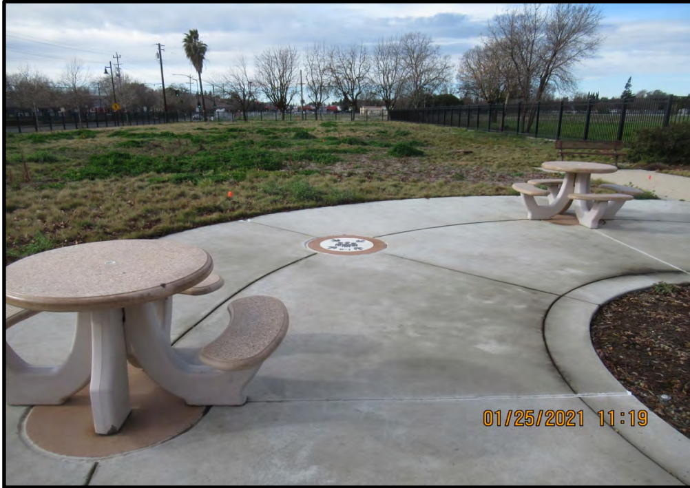
Seating area in the northeast corner of the Phase 2 Building site, looking southwest along the north edge of the site; 01/25/21.
