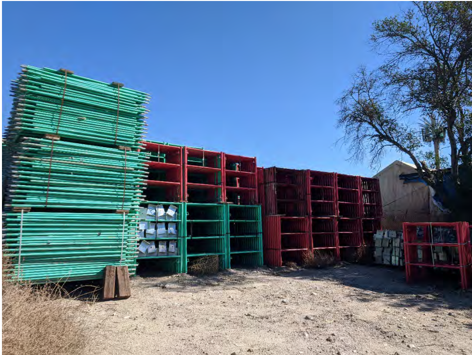
Photo 2: View of staged scaffolding equipment in the Study Area. Photo taken February 5, 2022.
