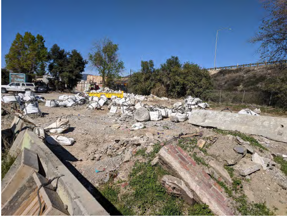
Photo 1: View of construction debris in the Study Area. Photo taken February 5, 2022.
