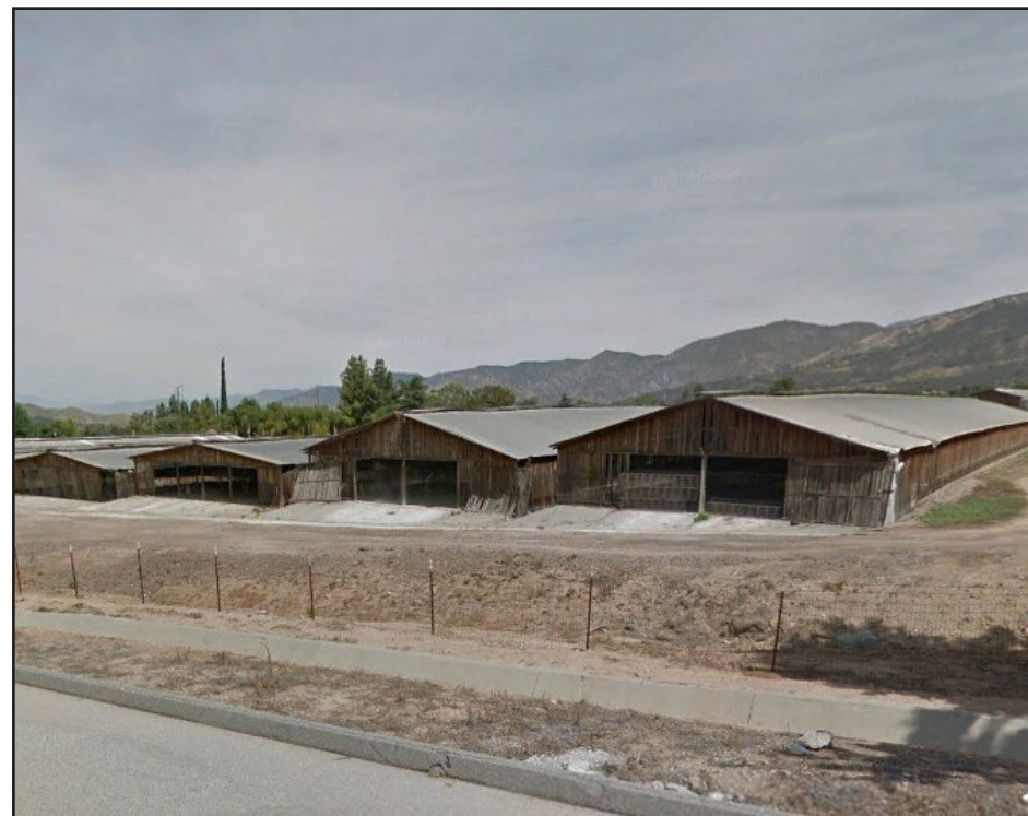
⑤ View 5: From the western portion of the project site along Fir Avenue, looking northwest to chicken ranches on the project site.
