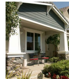
Stone Pier and Battered Wood Support
