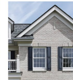
Cornice Returns on the Gable Ends
