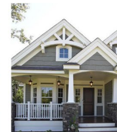
Wood Corbels and Wood Railings
