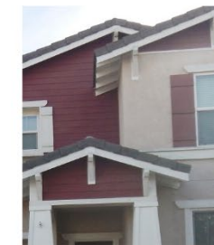
Exposed Rafter Tails and Knee-Brace Brackets
