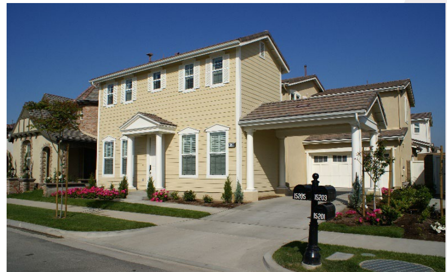
A porte-cochere architectural element may be used to provide covered parking area.
