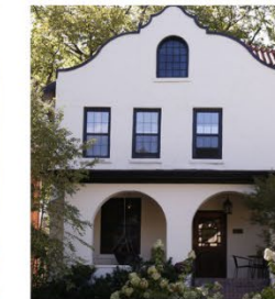
Mission-Shaped Roof Parapet
