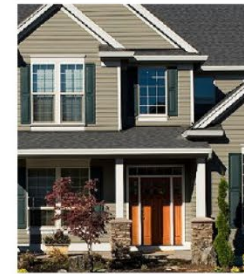
Porch with Slender Columns
