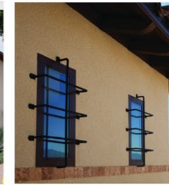
Windows with Metal Grilles
