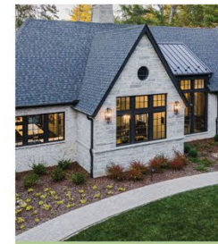
Stone or Brick Walls
