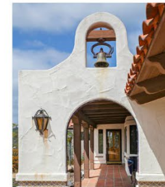
Exposed Wood Beams
