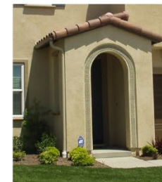
Arched Window/Door Openings
