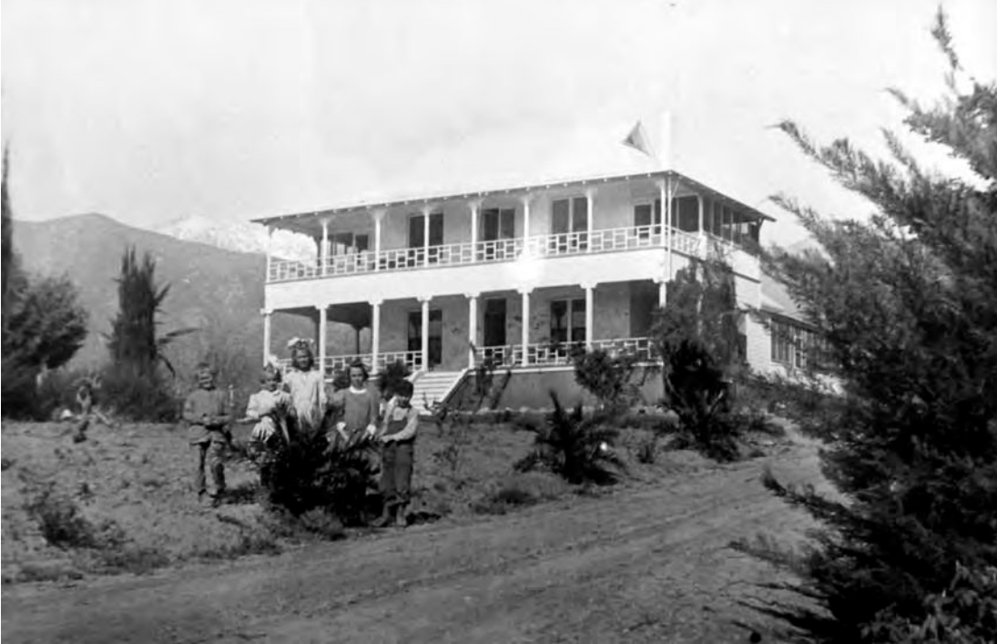
Atwood house (Feature 1), circa 1912, after the addition of the second-story porch. Front (west) and south elevations. View to northeast. (Photo courtesy of Yucaipa Valley Historical Society Museum)
