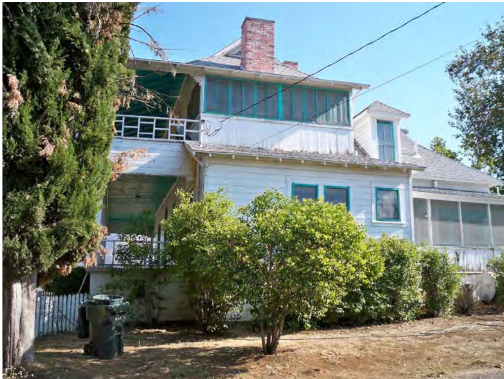
Casa Blanca Ranch house (Feature 1), south elevation. View to north, 8/17/2012.
