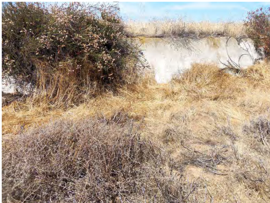
Concrete-lined earth dam (Feature 12a), upstream side. View to west, 8/15/2012.
