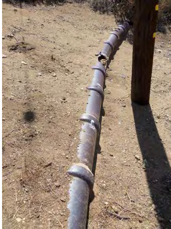
Terra cotta pipe (Feature 12g) north of holding pond (Feature 12f). View to southeast, 8/15/2012.
