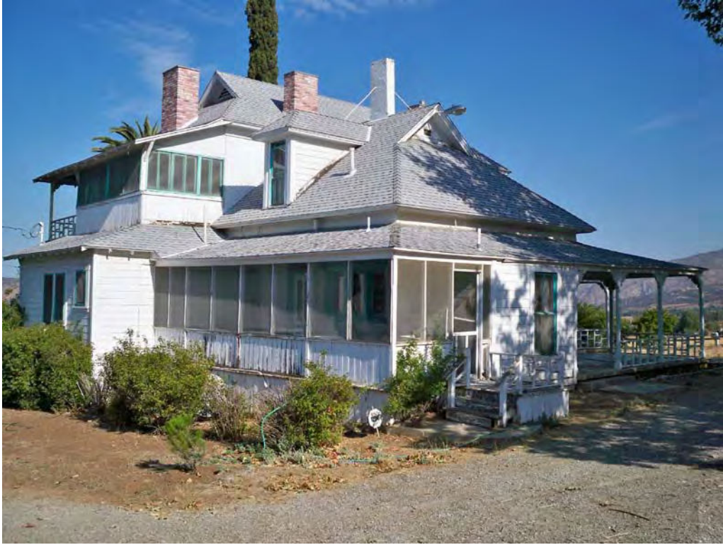
Casa Blanca Ranch house (Feature 1), south and rear (east) elevations. View to northwest, 8/17/2012.
