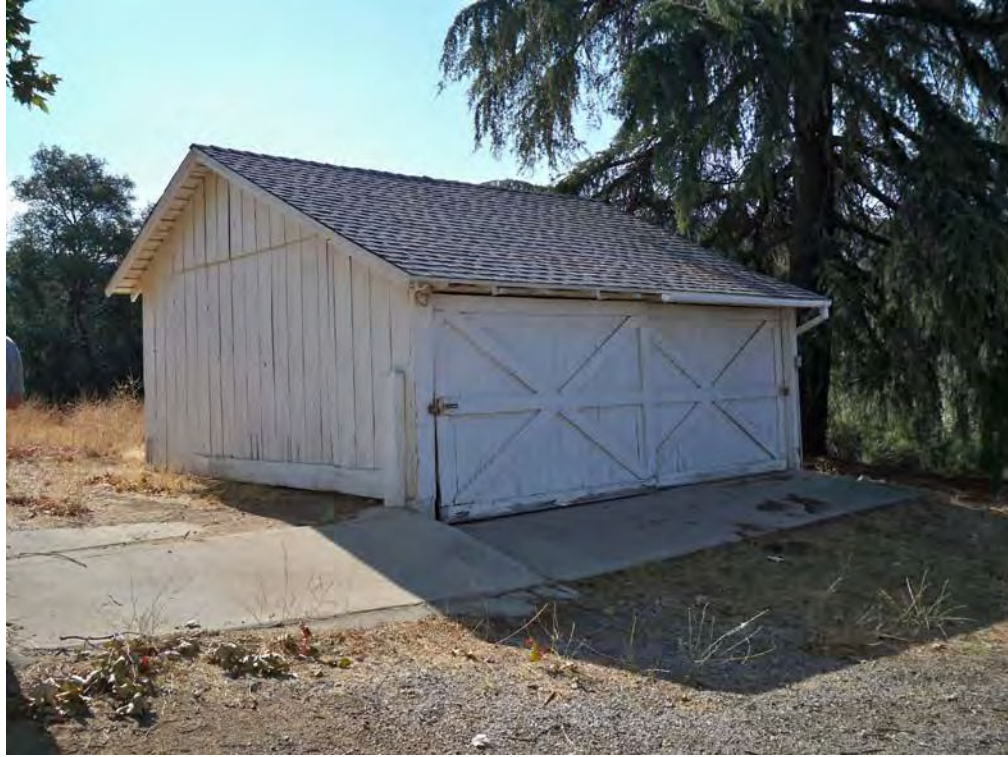
Garage (Feature 2), north and west (front) elevations. View to southeast, 8/17/2012.
