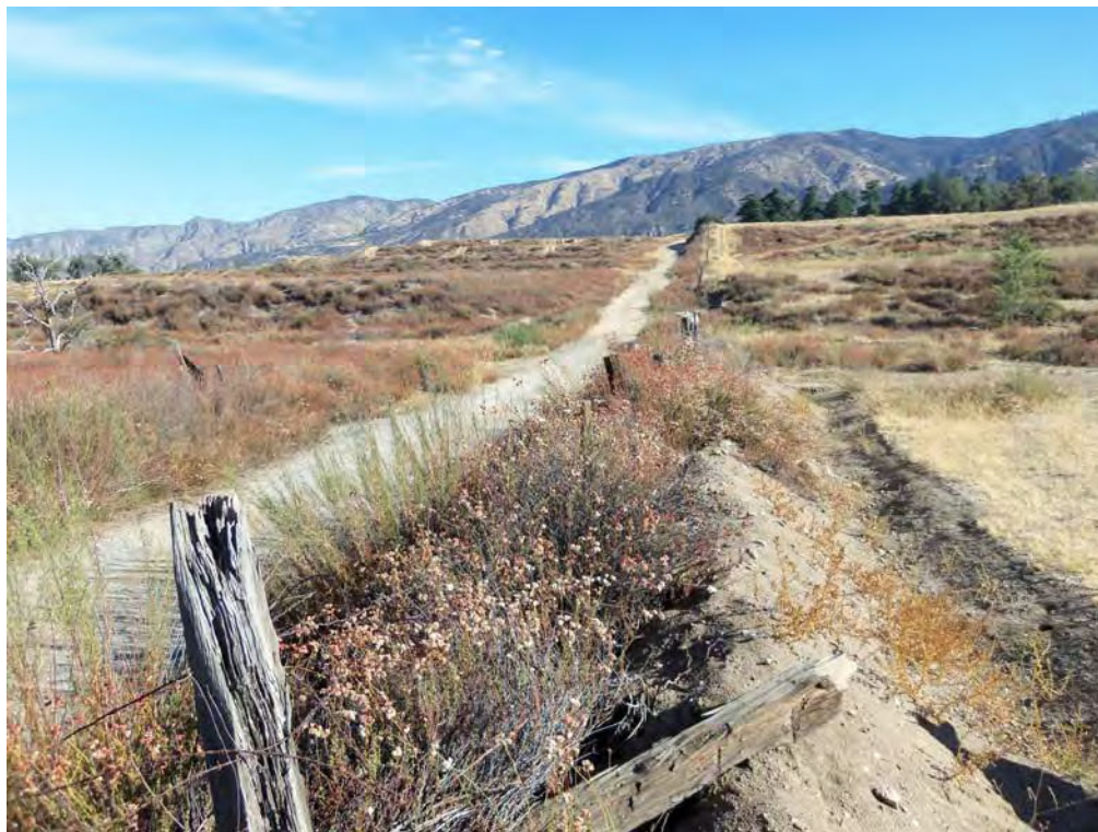
Fence line along west boundary of site (Feature 15). View to north, 8/15/2012.
