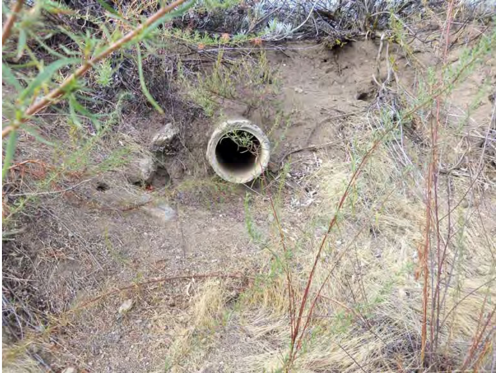
Concrete irrigation pipe in north half of site (Feature 25). View to south, 8/16/2012.
