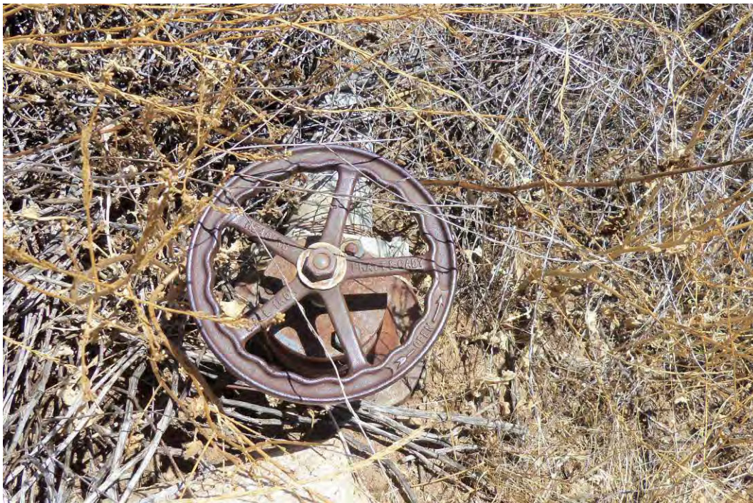
Valve wheel on west side of holding pond (Feature 12f). View to west, 8/15/2012.
