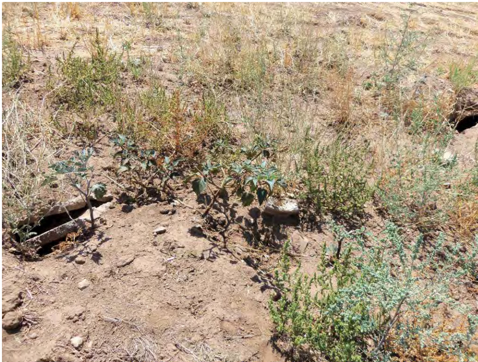
Concrete pipe in northeast quarter of site (Feature 29b). View to southwest, 8/16/2012.
