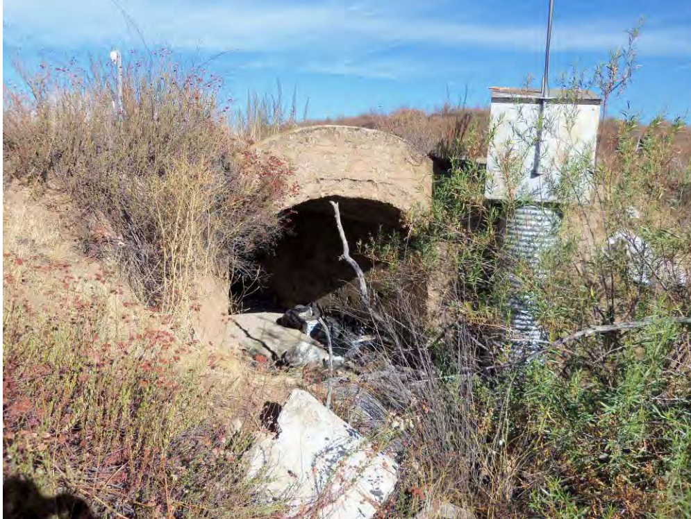
Wilson Creek concrete culvert (Feature 16) under Jefferson Street. View to west, 8/15/2012.
