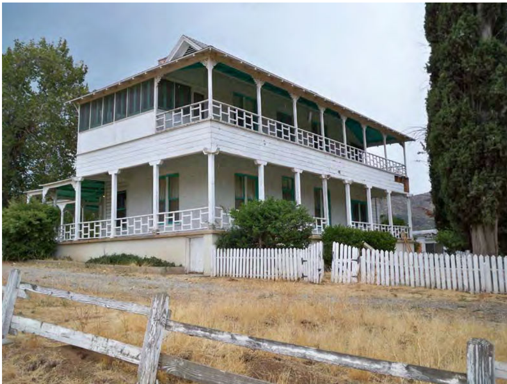
Casa Blanca Ranch house (Feature 1), north and front (west) elevations. View to southeast, 8/17/2012.
