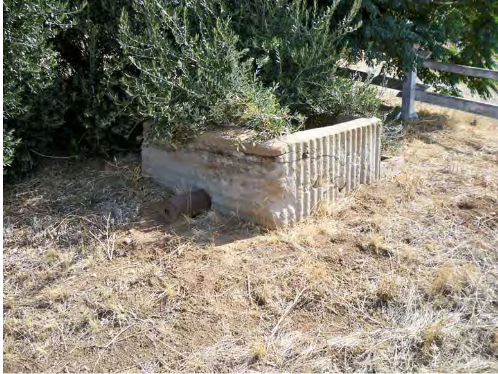
Concrete weir box (Feature 10) near Rodriguez house (Feature 5). View to northeast, 8/17/2012.
