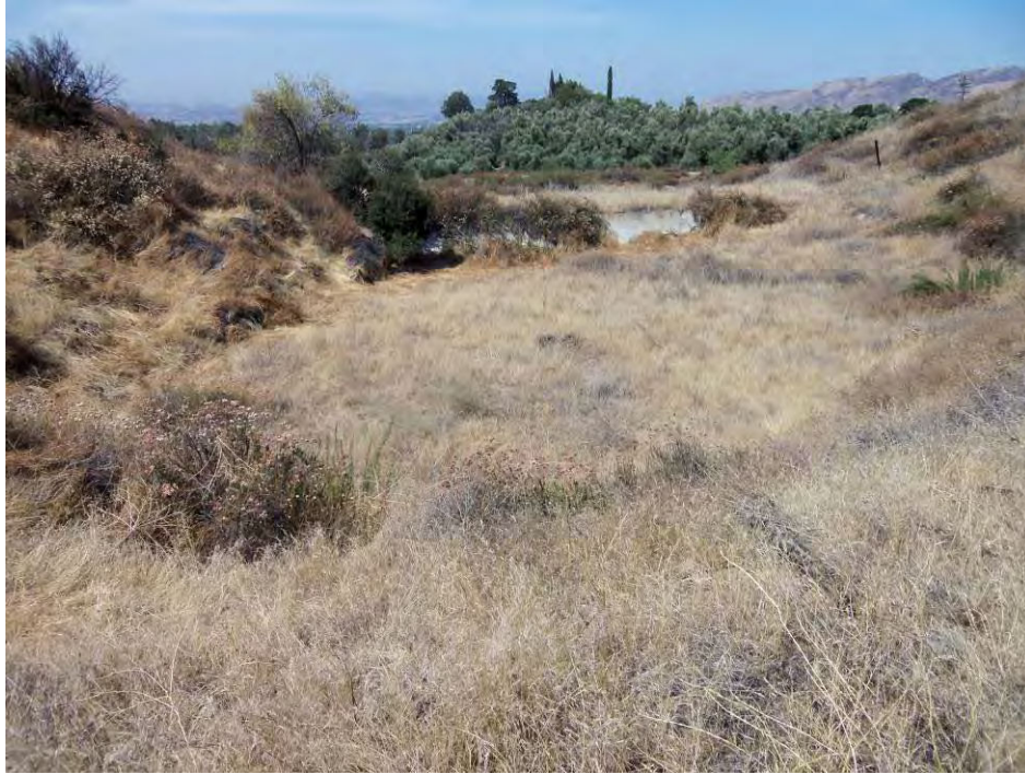
Concrete-lined earth dam (Feature 12a) in background, retention basin (Feature 12b) in foreground. View to southwest, 8/15/2012.
