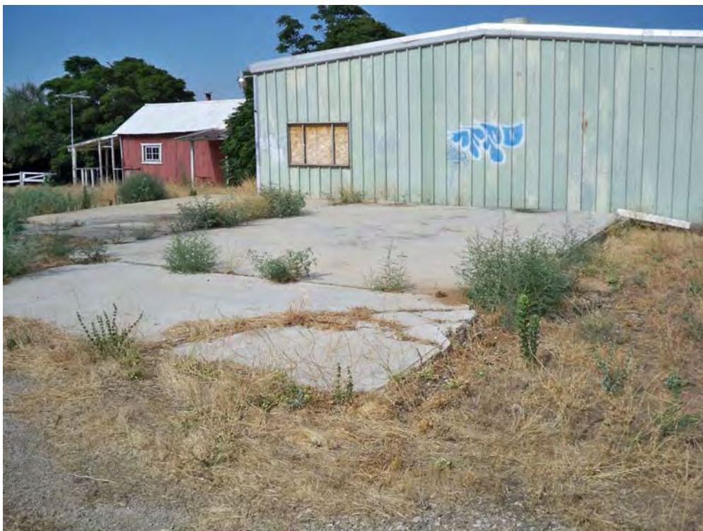
Modern prefabricated metal building and concrete slab (Feature 6) in foreground, Rodriguez house (Feature 5) in background, east elevations. View to southwest, 8/17/2012.
