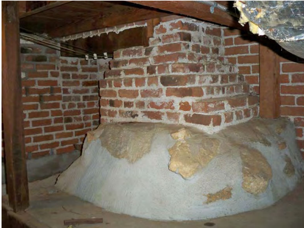
Casa Blanca Ranch house (Feature 1), stone and brick footing inside front basement. View to northwest, 8/17/2012.
