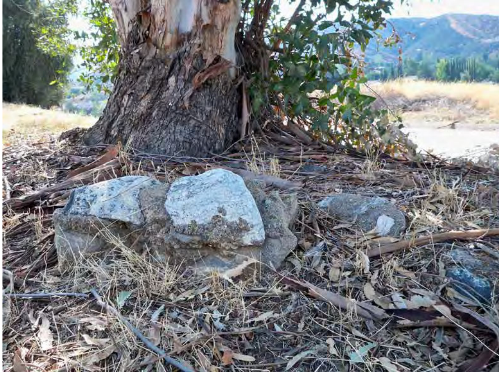
Remains of southern pillar of Casa Blanca Ranch entry gate (Feature 7). View to southeast, 8/17/2012.
