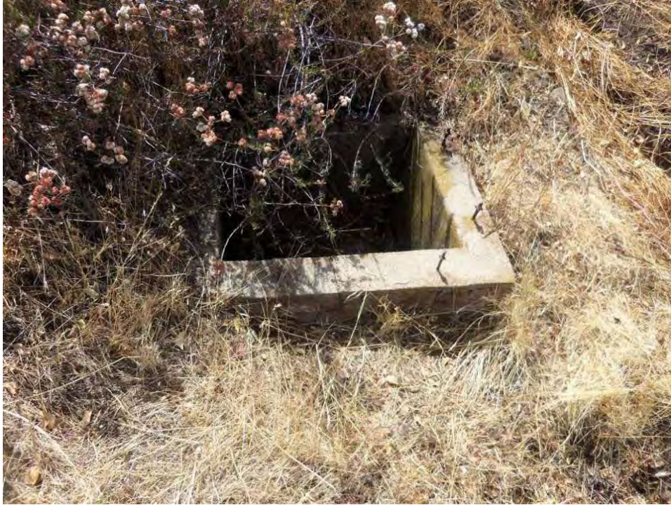
Concrete weir box (Feature 12c) next to concrete-lined dam (Feature 12a). View to east, 8/15/2012.
