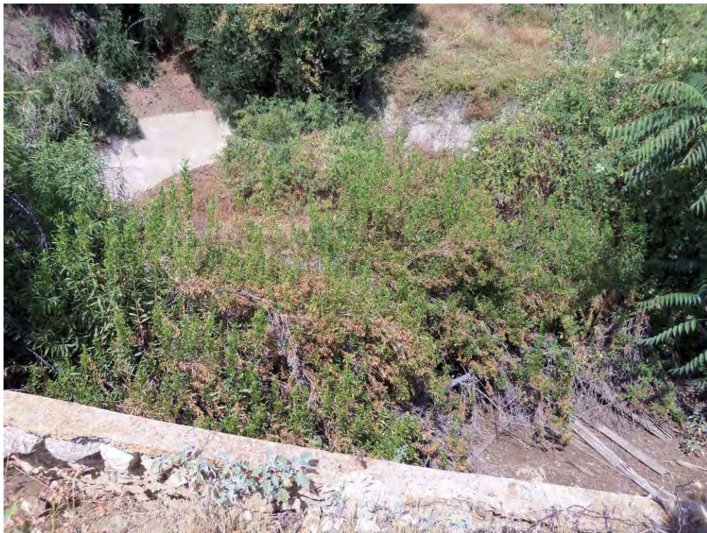
Concrete reservoir (Feature 22d). View to northeast, 8/15/2012.
