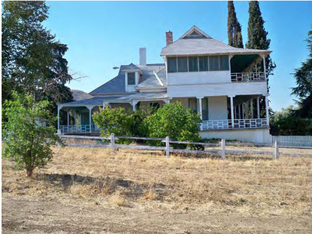
Casa Blanca Ranch house (Feature 1), north elevation. View to south, 8/17/2012.
