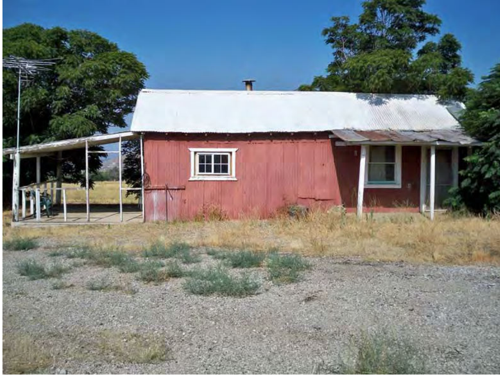
Rodriguez house (Feature 5), east elevation. View to west, 8/17/2012.
