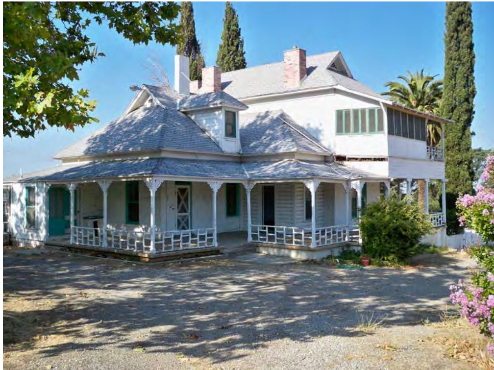
Casa Blanca Ranch house (Feature 1), Rear (east) and north elevations. View to southwest, 8/17/2012.
