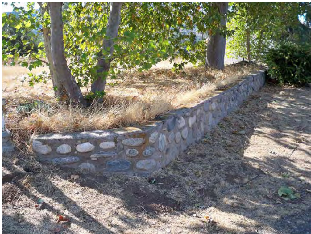
Stone retaining wall (Feature 8) behind main house (Feature 1). View to southeast, 8/17/2012.
