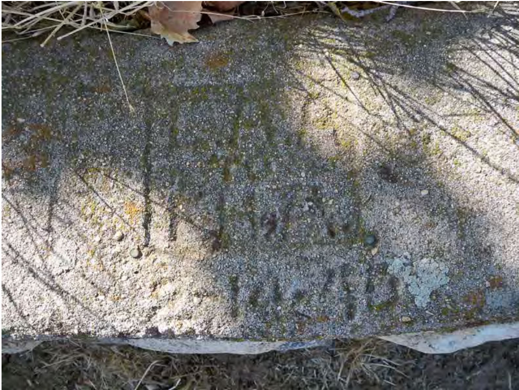
"L.A.A. to F.H.A", "2-14-40" inscribed in stone retaining wall (Feature 8). View to south, 8/17/2012.
