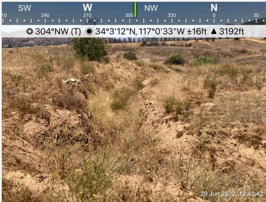
Photo 17. View of a ditch grown over with post-fire herbaceous species in the southern portion of the Project site, facing northwest.
