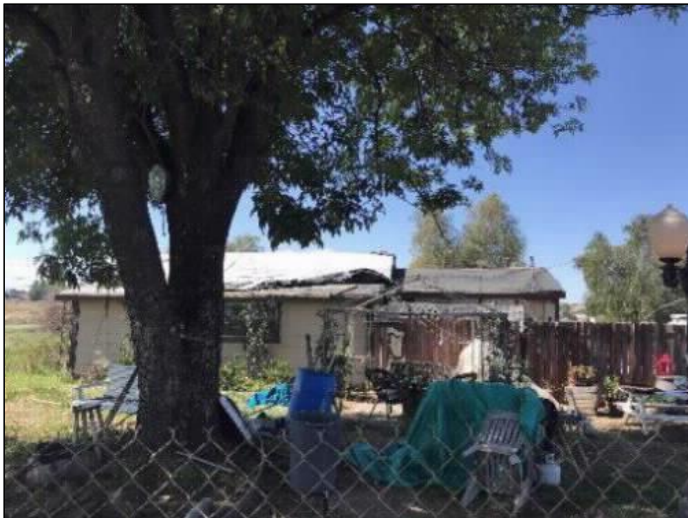
Figure 27. Overview of historic residence, view east
