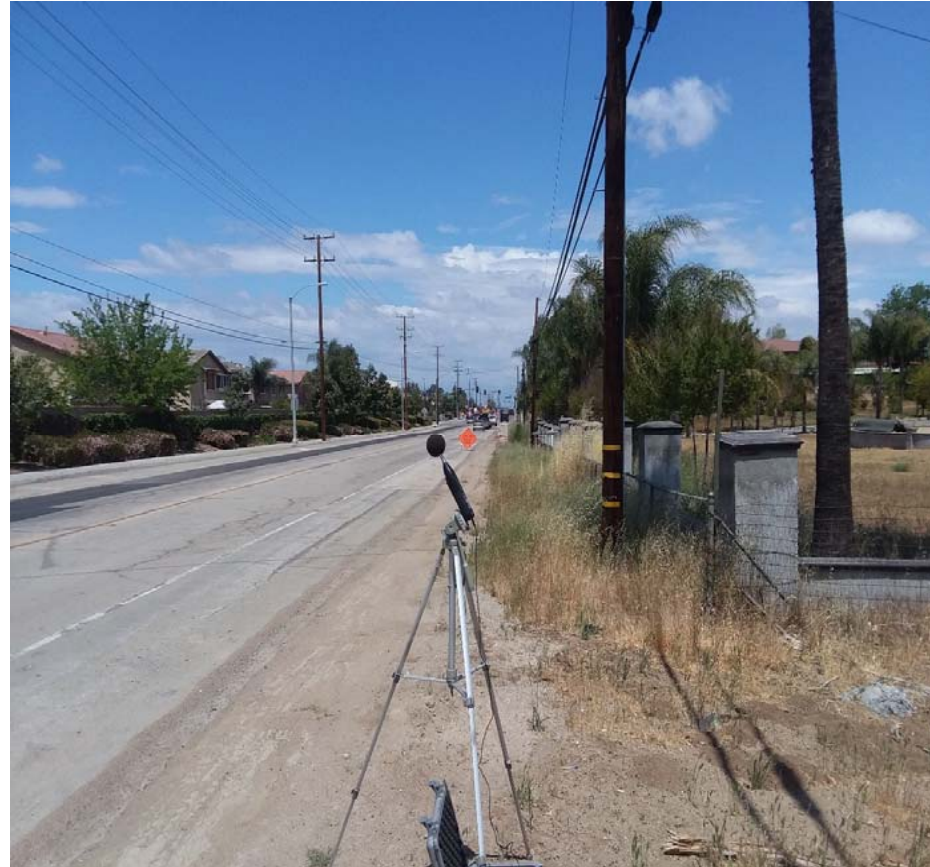
NM2 looking N up Wood Road towards Krameria Avenue intersection ( 220 yards ), road works in operation just beyond intersection. Residence 16588 Wood Road, Riverside on the right of photo.
