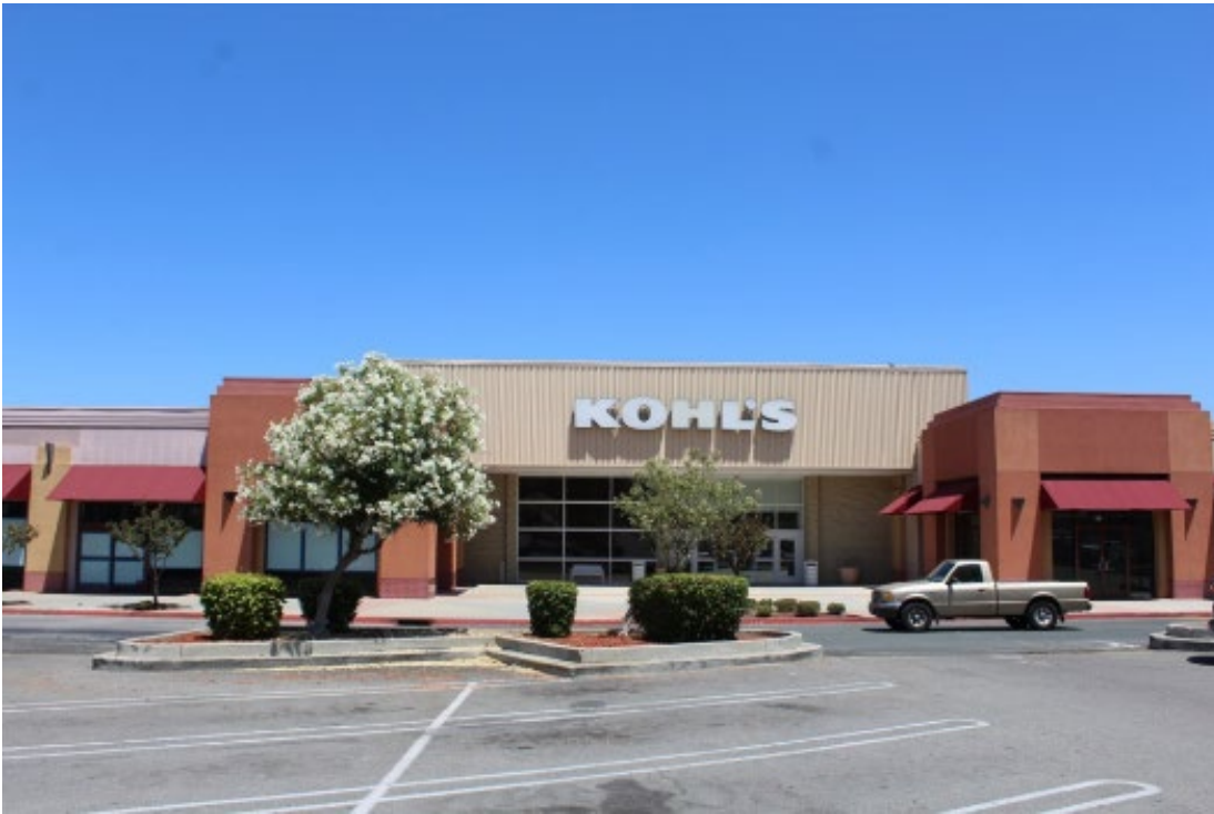
Photograph 9: 350 Showers Drive, south elevation, camera facing northeast, July 26, 2022.
