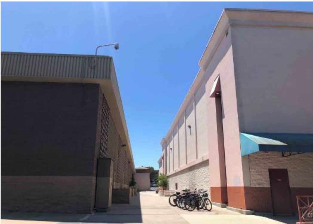
Photograph 11: 350 Showers Drive north elevation and 2535 California south east elevation, camera facing southwest, July 26, 2022.
