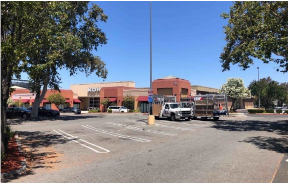
Photograph 8: 350 and 510 Showers Drive, south and east elevations, camera facing northeast, July 26, 2022.
