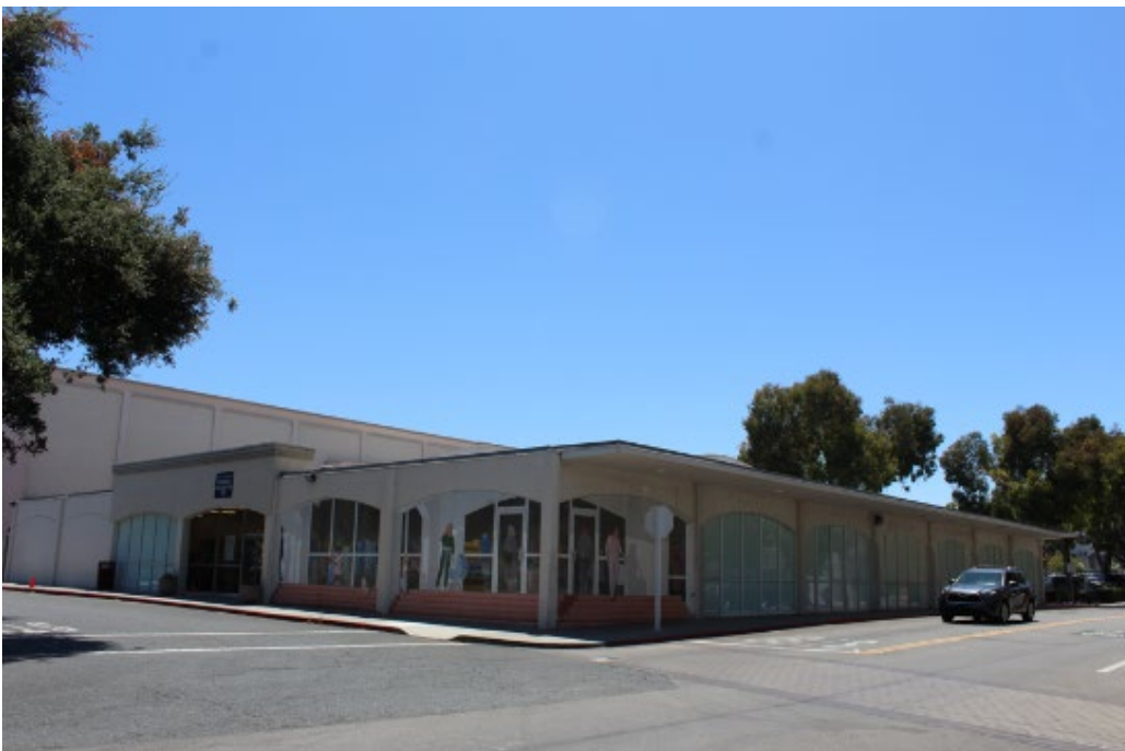
Photograph 3: 435 San Antonio Road, east and north elevations, camera facing southwest, July 26, 2022.
