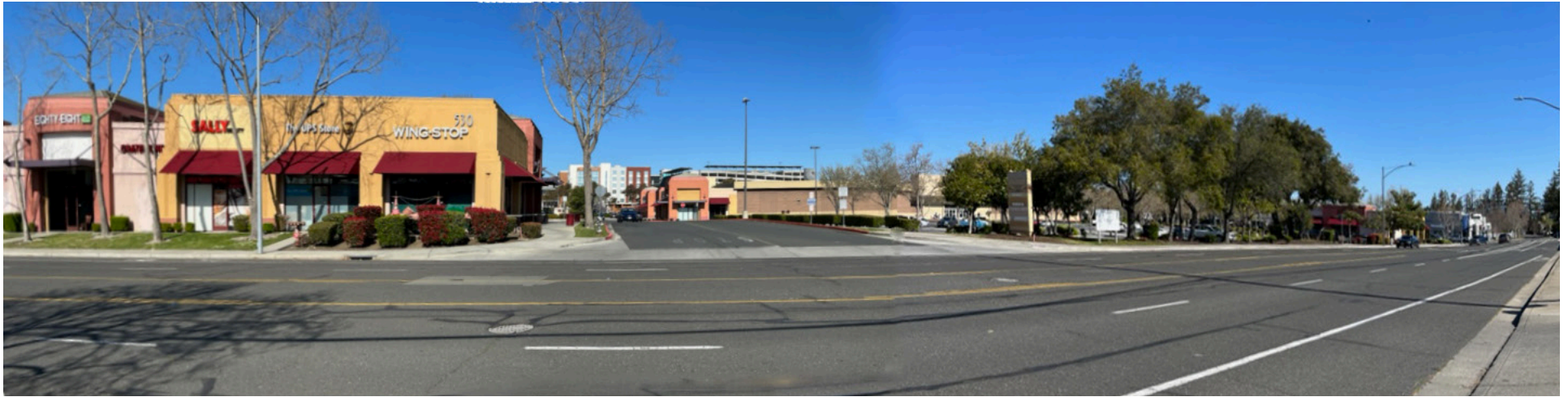
A. View of Showers Drive site frontage, looking northwest, with main entrance at center of photo. Existing commercial buildings at left would remain. Street trees on right screen view of site where new school would be built.
