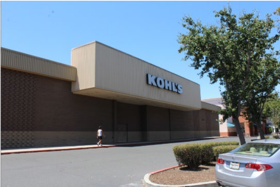
Photograph 7: 350 Showers Drive, north elevation, camera facing west, July 26, 2022.
