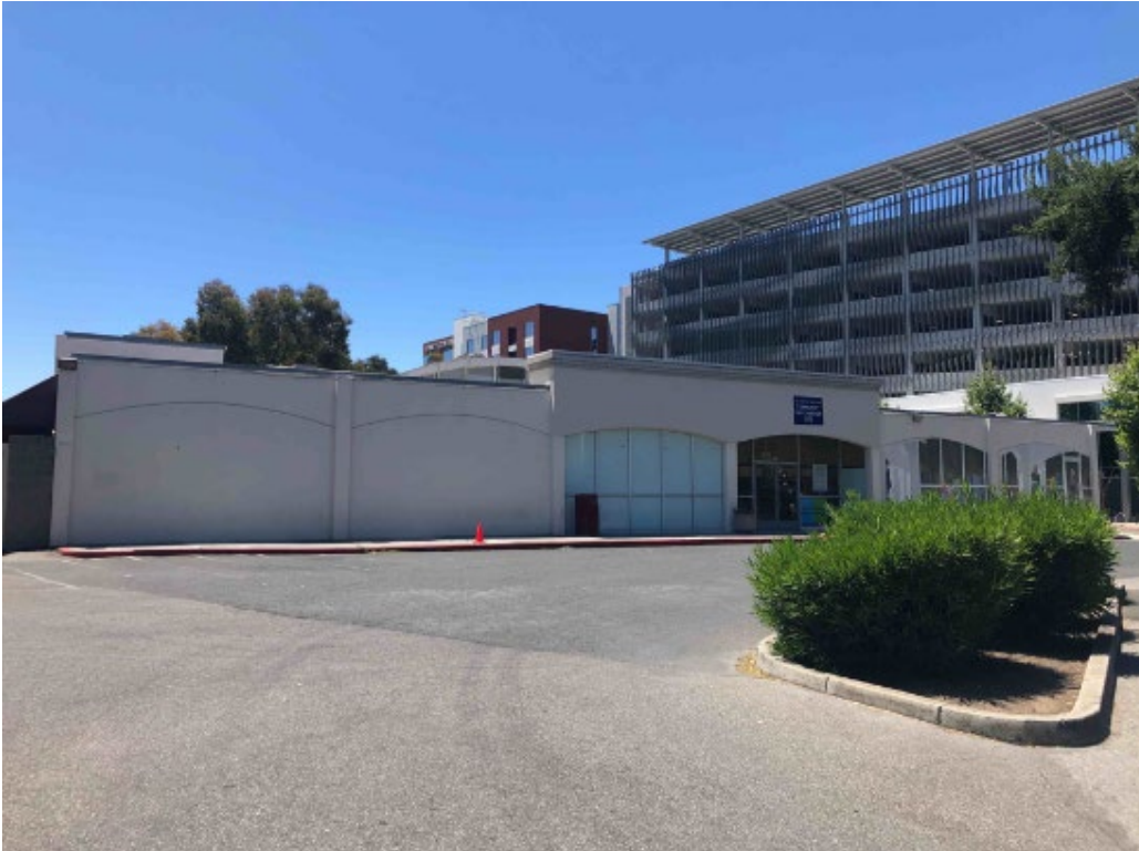
Photograph 2: 435 San Antonio Road, east elevation, camera facing southwest, July 26, 2022.
