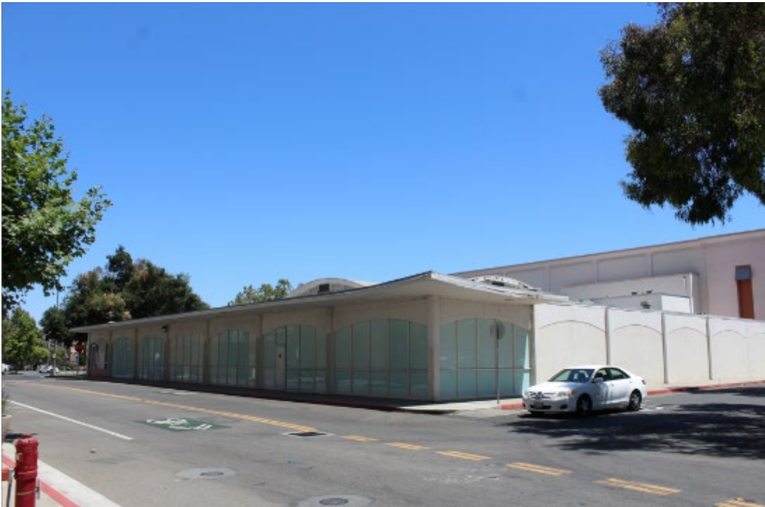
Photograph 4: 435 San Antonio Road, north and west elevations, camera facing southeast, July 26, 2022.
