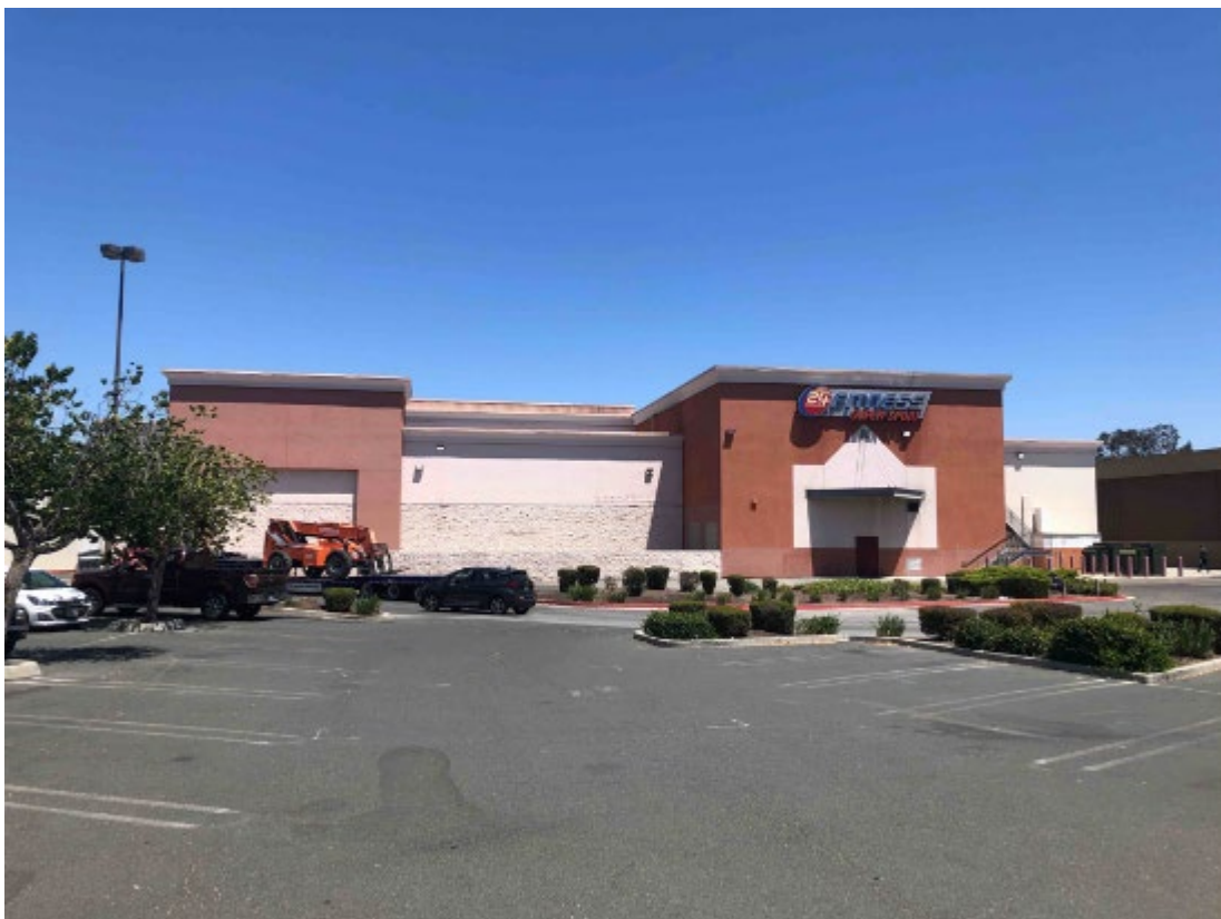
Photograph 12: 2535 California Street, west elevation, camera facing northeast, July 26, 2022.
