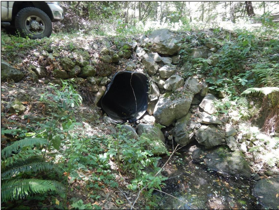
Photo 7. The culvert and stream crossing over the unnamed Class II watercourse in the northwestern portion of APN: 105-101-011. This may need to be replaced in order to comply with regulation sizing (Map 2).
