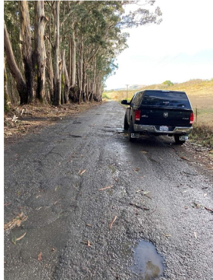
Image 4. Representative of RS2 conditions (looking west). Details asphalt surface, 20'+ average road width, shoulders, turnouts, crowned geometry with fair drainage, average slopes <5% - max <12%.
