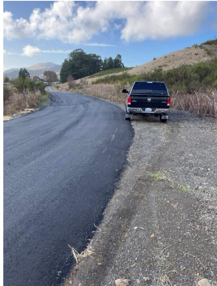
Image 6. Representative of RS2 conditions (looking west). Details asphalt surface, 20'+ average road width, shoulders, turnouts, crowned geometry with fair drainage, average slopes <5%.
