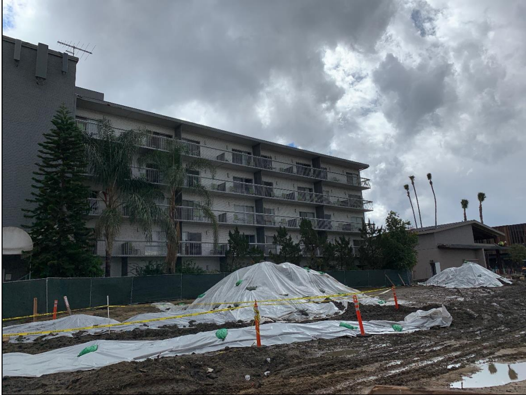
Photo 1. Construction work area in the existing parking lot, view facing southwest
