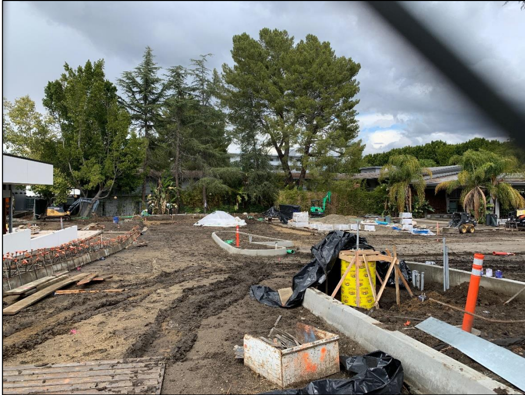
Photo 3. Construction work area adjacent to the hotel, view facing northeast
