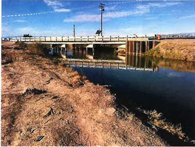
Photograph 3: Looking at the bridge from the east.
