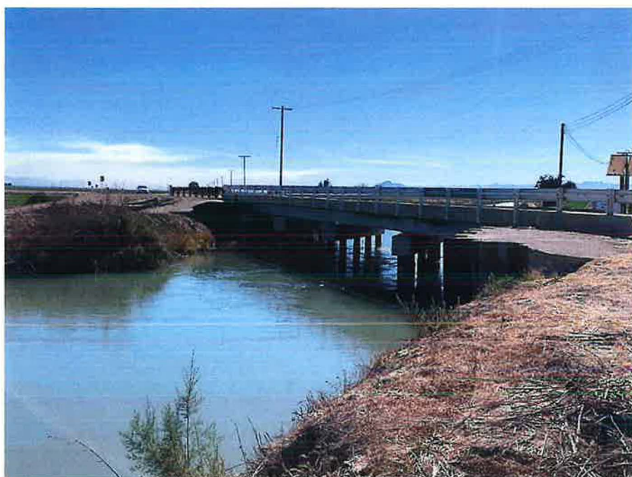
Figure 6. View of CA-IMP-7834, Westside Main Canal from the central portion of the survey coverage area facing south, also showing Bridge No. 58C-0114.
