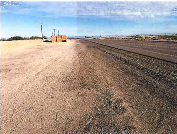
Photograph 5: Roadway to the south of the bridge.
