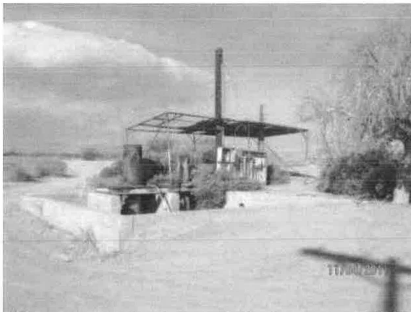
IMG_2832 view to west. Reservoir, shed roof and panel.
