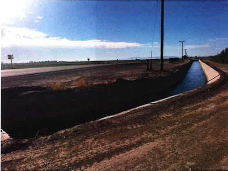
Photograph 8: Looking south at the Westside Canal.
