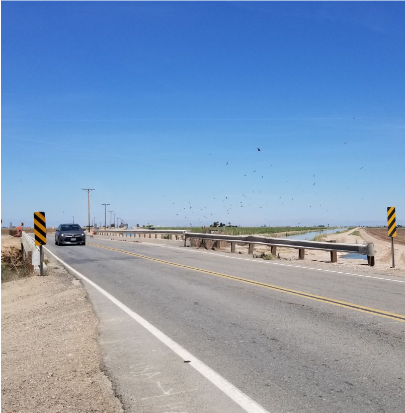
Figure 2 Project Site Photos
