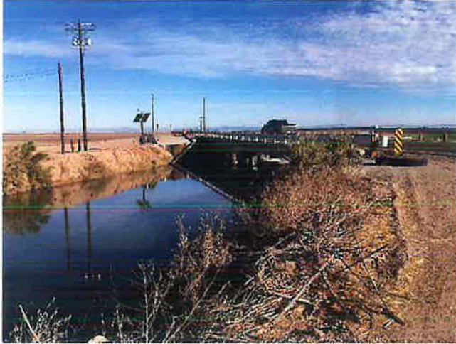
Photograph 6: West side of the bridge.
