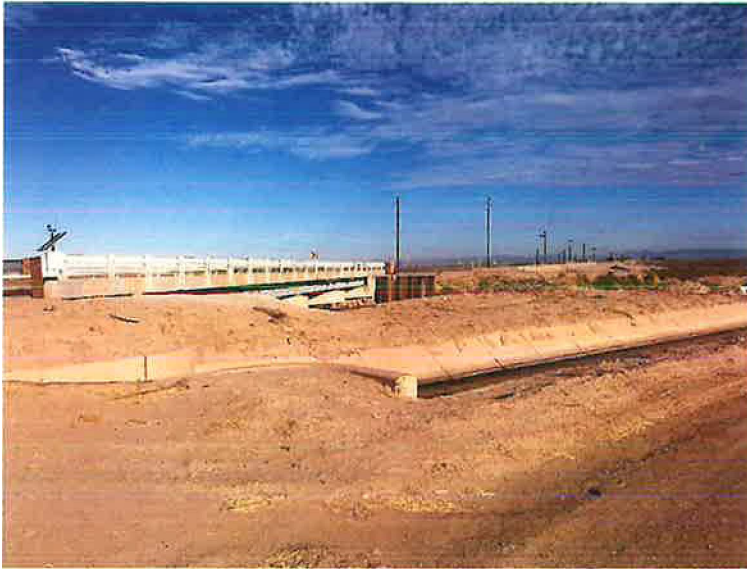
Photograph 1: Looking at the bridge from the southeast.
