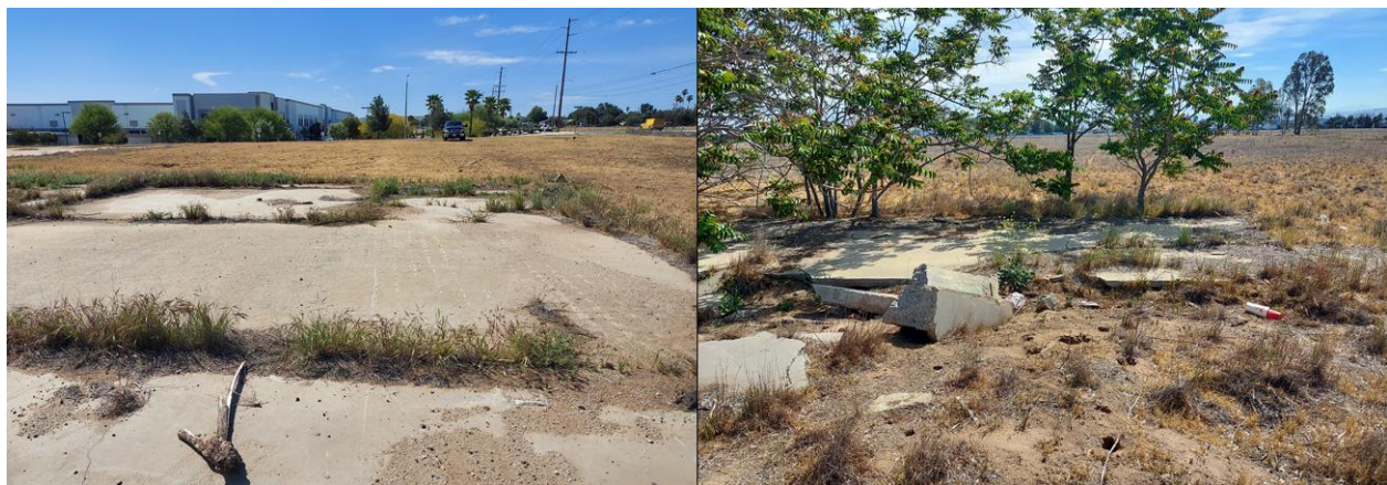
Figure 10. Structural remains in the project area. Left : foundation of a barn built before 1939; right : foundation of a small building constructed in 1967-1978. (Photographs taken on April 19, 2022)
