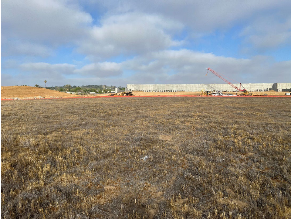
Photo 15 – View from eastern side of Property towards the west.
