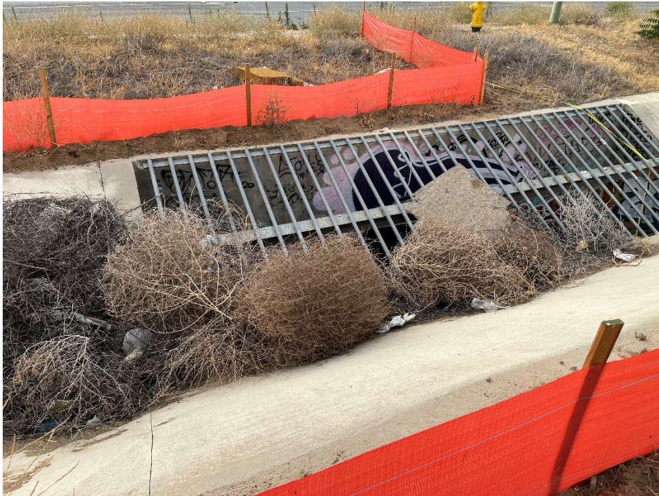
Photo 10 – Stormwater drain at southeastern corner of the Property.
