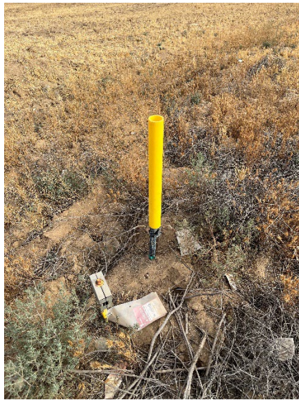
Photo 14 – Marker for SoCal Gas line along eastern side of Property.
