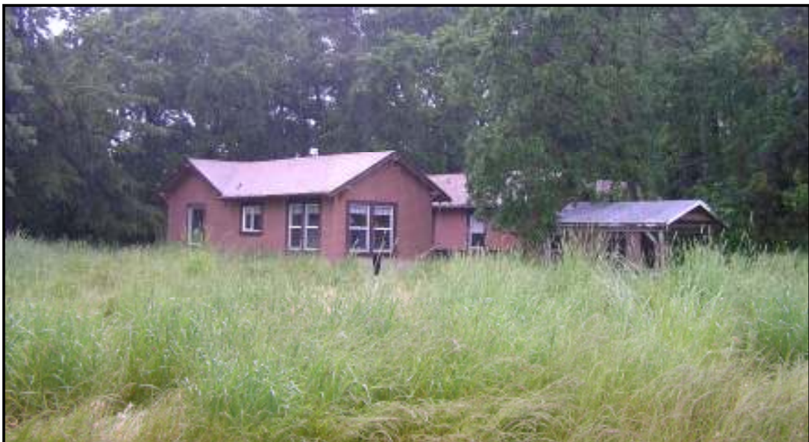
Figure 6. View of the south and east (rear) house elevations.
