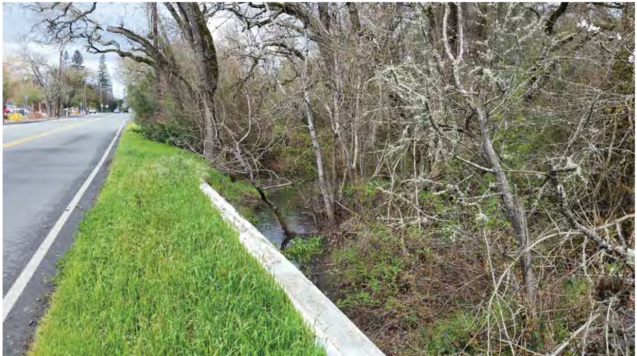
Photo 6: Viewing north along the project site frontage on Burbank Avenue from the Roseland Creek bridge.
