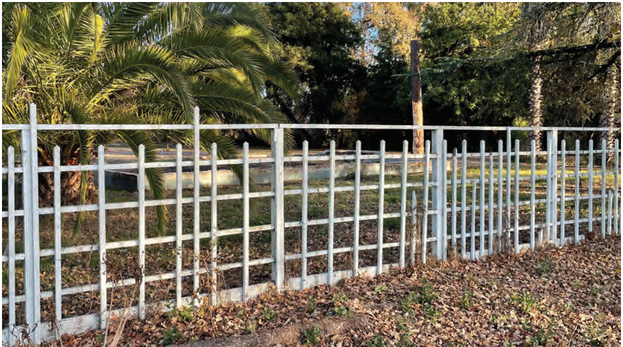
Photo 2: View of 1370 Burbank Avenue property, looking southeast, with remnant fencing and building foundation in the foreground.
