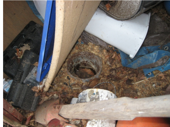
Photo 22: Grouted well in Pump House.
