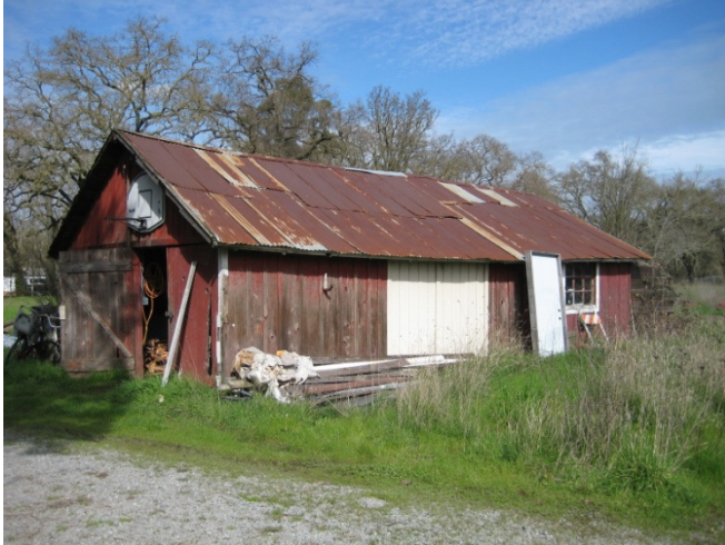
Photo 7: South Side of Barn.
