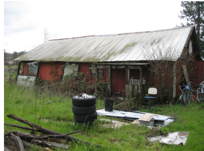
Photo 6: North side of barn.
