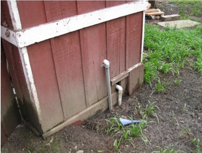
Photo 21: West side of Pump house.
